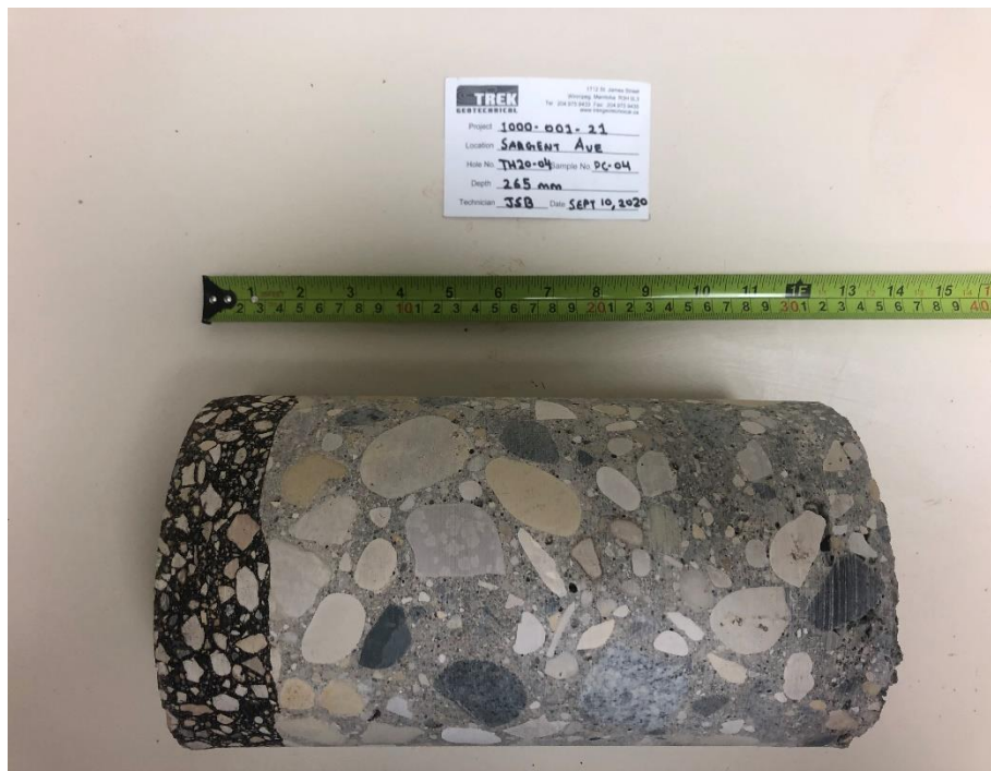
Photo 4: Pavement Core Sample at Test Hole TH20-04
