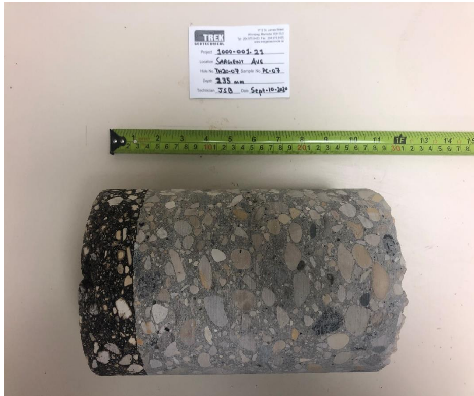
Photo 7: Pavement Core Sample at Test Hole TH20-07
