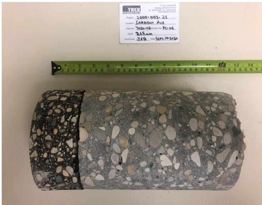
Photo 6: Pavement Core Sample at Test Hole TH20-06
