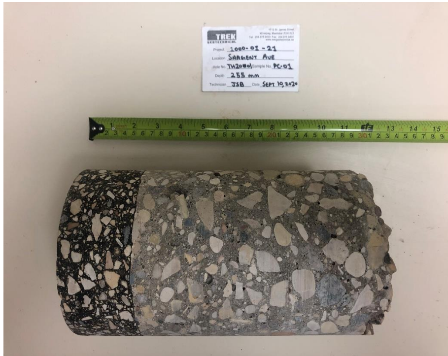
Photo 1: Pavement Core Sample at Test Hole TH20-01
