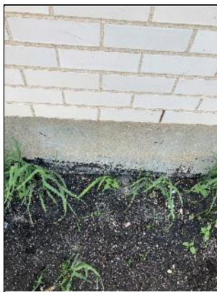
Asbestos-containing tar mastic in GOOD condition.
