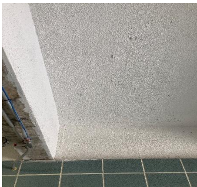
Asbestos-containing textured ceiling finish observed in GOOD condition.
