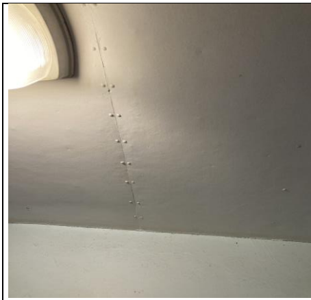
Transite cement board presumed to contain asbestos in GOOD condition.
