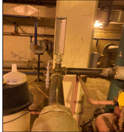
Damaged fittings removed, Location No.11
