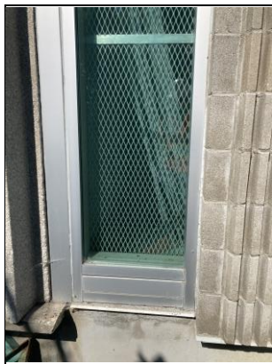
Asbestos-containing caulking in GOOD condition.
