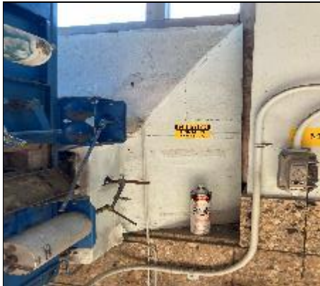
Asbestos-containing parging cement on ducting in GOOD condition.
