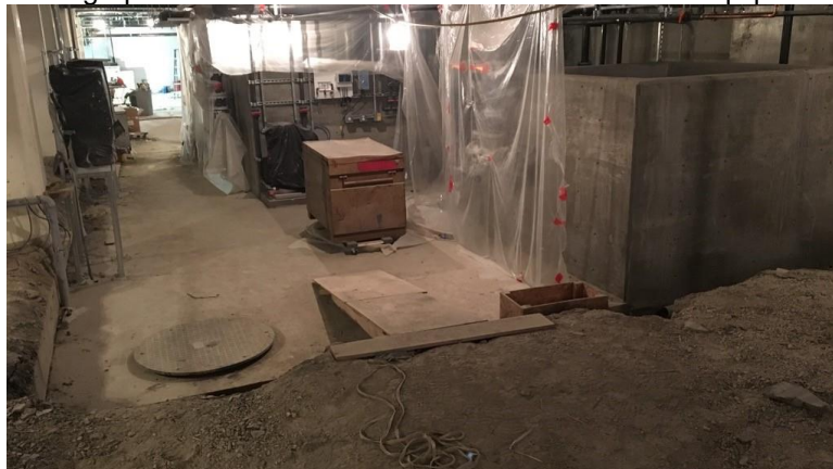
Photograph 3.2.1.1-2: Partial view of new mechanical equipment.
