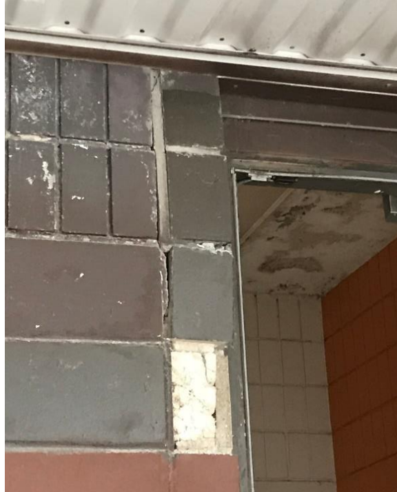
Photograph 3.3.1.4-6: Localized mortar joint deterioration at the bottom ledger course of the brick cladding and caulking debonding at the brick masonry control joint was observed.
