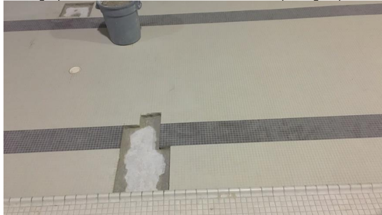
Photograph 3.2.2.2-1: Soffit delamination and spalling at pool tank drain.
