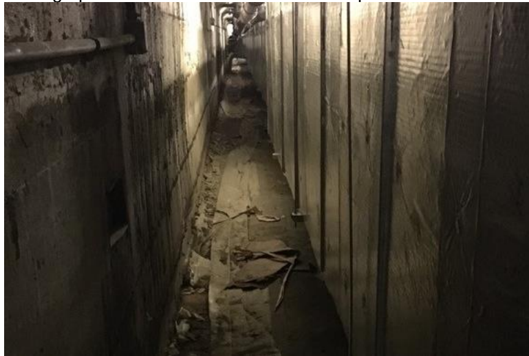
Photograph 3.2.1.1-4: Partial view of crawlspace below the west pool deck.
