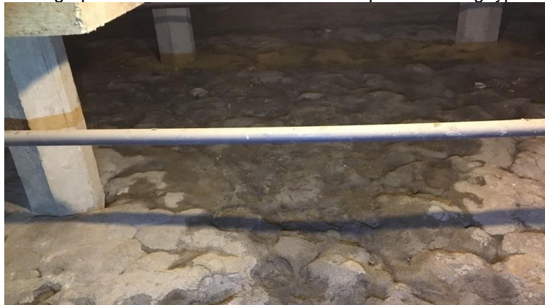
Photograph 3.2.1.1-6: Partial view of crawlspace showing typical ground cover.
