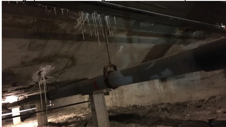
Photograph 3.2.2.1-4: Leakage and efflorescence in pool tank.
