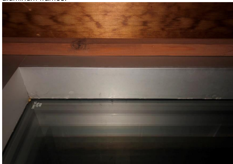
Photograph 3.3.2.1-3: Typical example of condensation and water staining on the aluminum frames.
