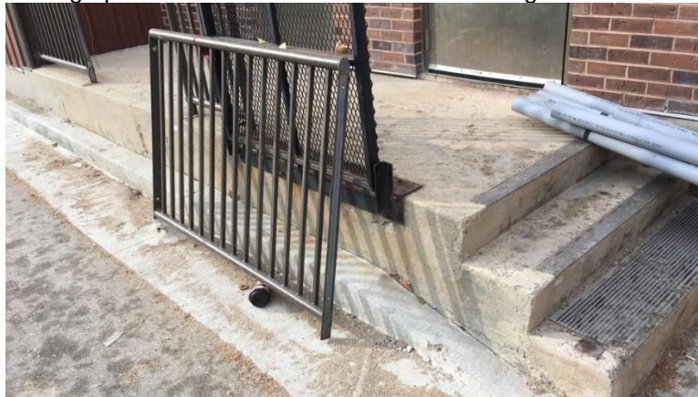
Photograph 3.1.1.1-1: Partial view of east loading dock.
