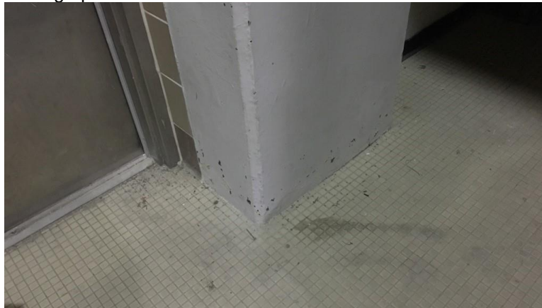
Photograph 3.2.2.5-1: Deterioration of concrete column.
