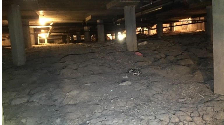
Photograph 3.2.1.1-5: Partial view of crawlspace below pool tank.
