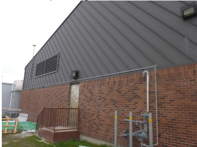
Photograph 3.3.1.4-2: Thermal bridging at the existing metal cladding steel girt support was observed during thermographic scanning along the West elevation.
