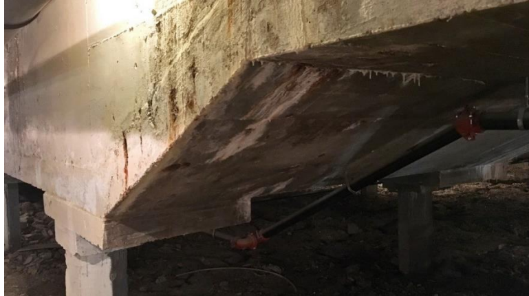
Photograph 3.2.2.1-1: Soffit delamination and spalling at pool tank drain.
