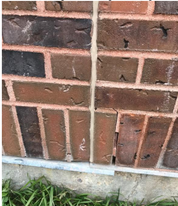
Photograph 3.3.1.4-6: Localized mortar joint deterioration at the bottom ledger course of the brick cladding and caulking debonding at the brick masonry control joint was observed.
