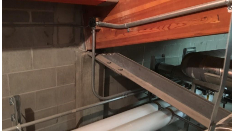
Photograph 3.2.4.2-1: Glulam tension tie at north support.
