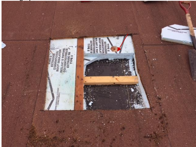
Photograph 3.3.3.1.4: View rusted fastener.
