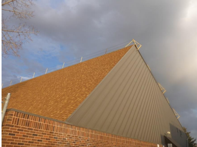
Photograph 3.3.1.4-3: General view of the existing metal cladding along the East elevation of the pool building.
