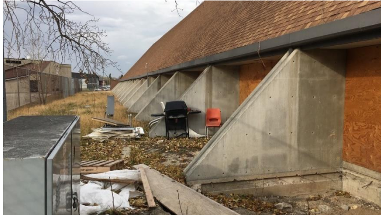
Photograph 3.1.2.3-1: Partial view of south elevation.
