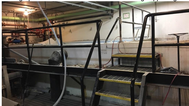
Photograph 3.2.1.5-1: Corrosion on steel framing supporting filtration room platform.
