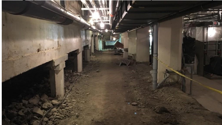
Photograph 3.2.1.1-1: Partial view of crawlspace below north pool deck.
