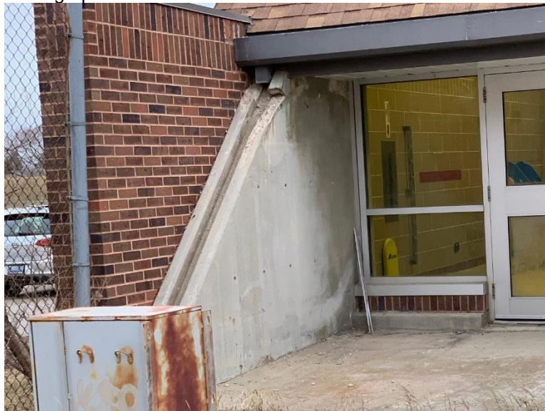
Photograph 3.1.2.4-1: Partial view of concrete buttress.
