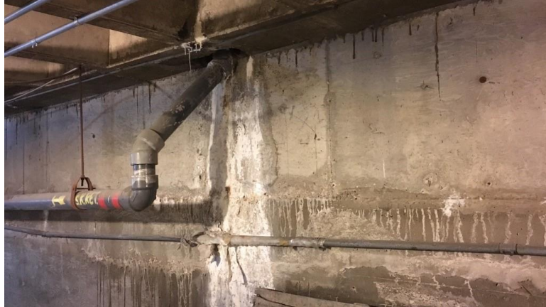
Photograph 3.2.2.1-6: Efflorescence at crack in pool tank wall.
