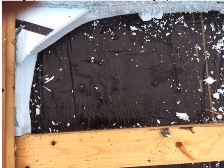
Photograph 3.3.3.1-2: View water on existing vapor barrier.
