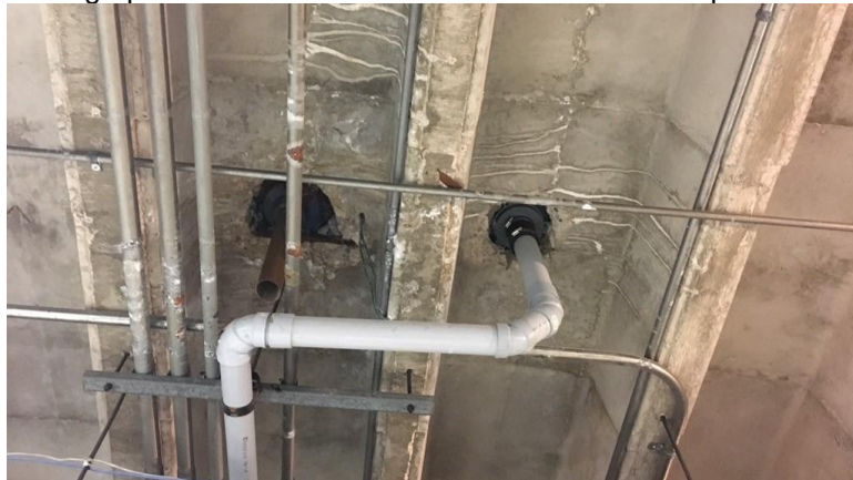
Photograph 3.2.2.1-7: Localized leaks below the east pool deck at a mechanical line.
