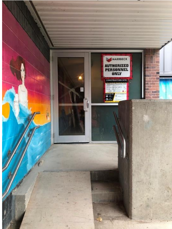
Photograph 3.3.2.2-2: North elevation entrance showing glazed aluminum door and aluminum curtain wall framed exterior glazed sidelight.
