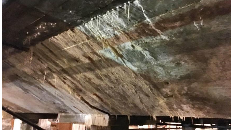
Photograph 3.2.2.1-3: Leakage and efflorescence along construction joint in pool tank.
