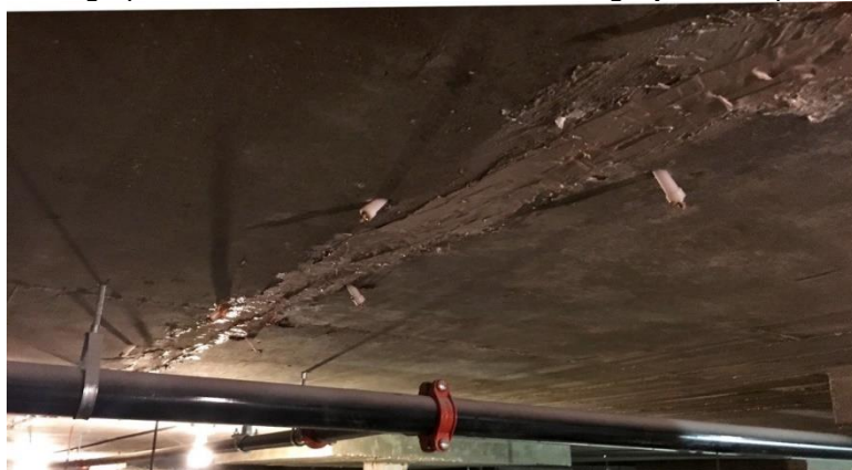
Photograph 3.2.2.1-2: Soffit delamination along injection repair.
