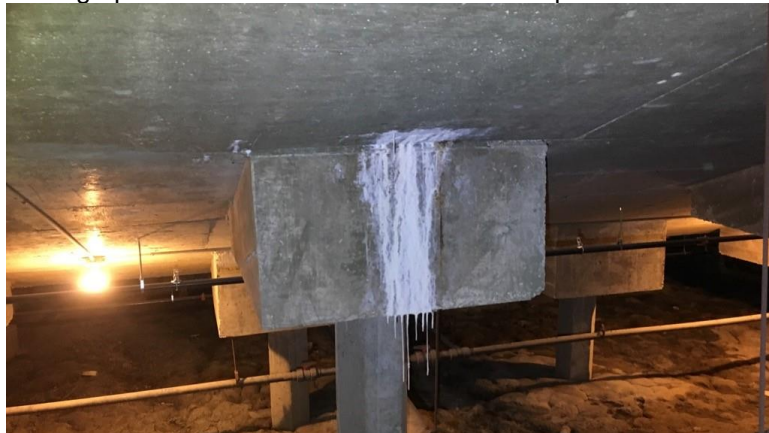
Photograph 3.2.2.1-5: Efflorescence at leak in pool tank.
