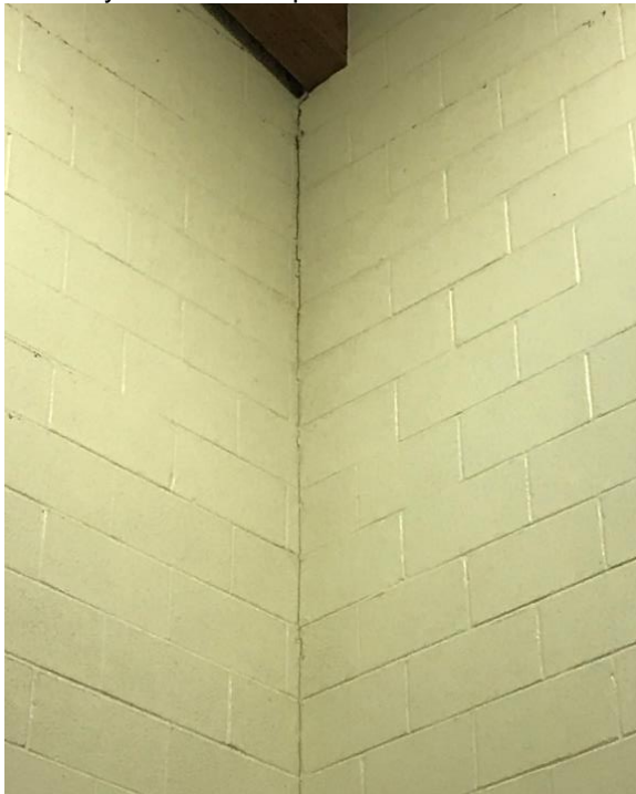
Photograph 3.3.1.4-8: Corner cracking observed at the interior face of the existing masonry block back-up.
