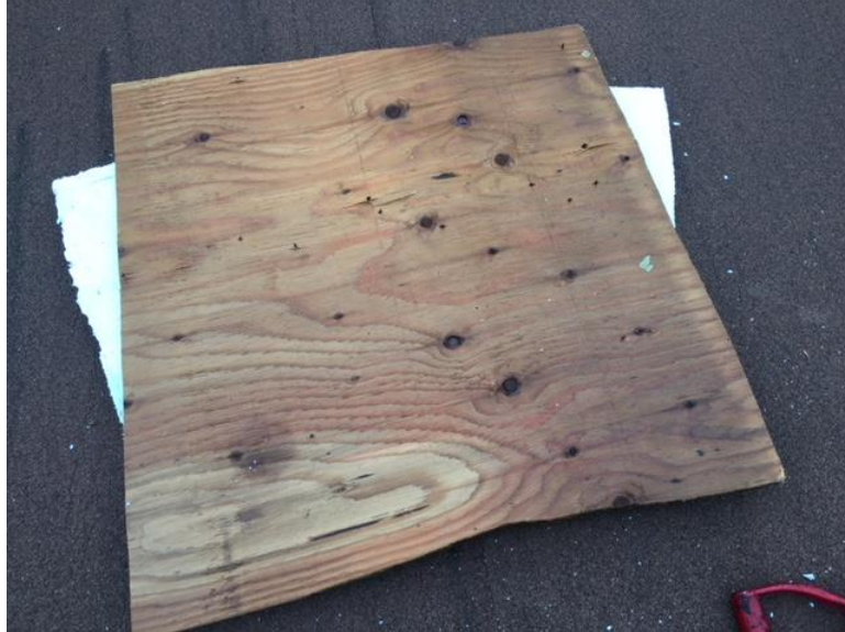
Photograph 3.3.3.1-3: Showing saturated plywood support panel.
