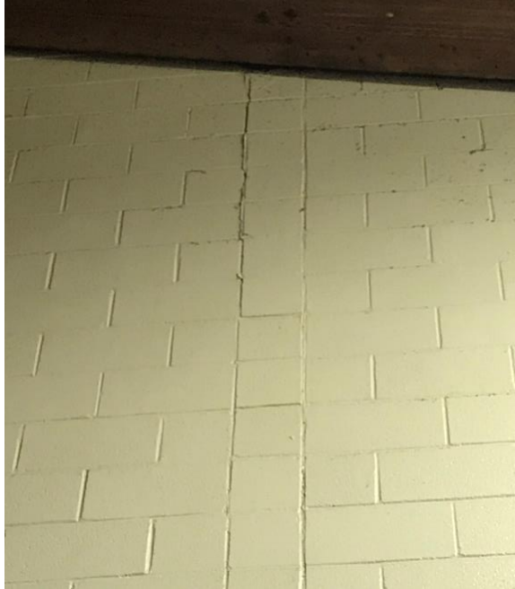
Photograph 3.3.1.4-8: Corner cracking observed at the interior face of the existing masonry block back-up.
