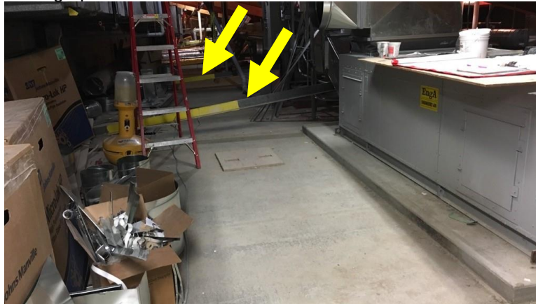
Photograph 3.2.4.2-2: Glulam tension tie connection to floor structure.
