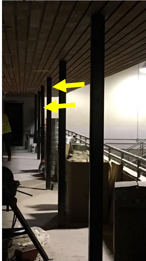
Photograph 3.2.4.2-3: Lateral deflection of HSS columns.
