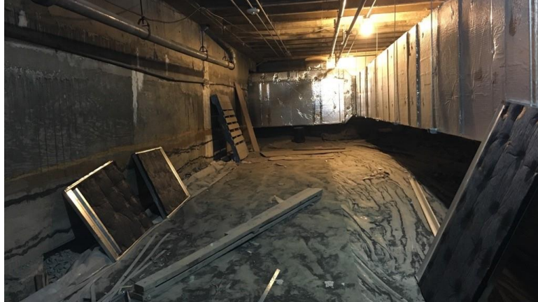
Photograph 3.2.1.1-3: Partial view of crawlspace below the west pool deck.
