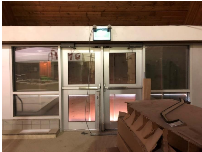
Photograph 3.3.2.2-2: North elevation entrance showing glazed aluminum door and aluminum curtain wall framed exterior glazed sidelight.
