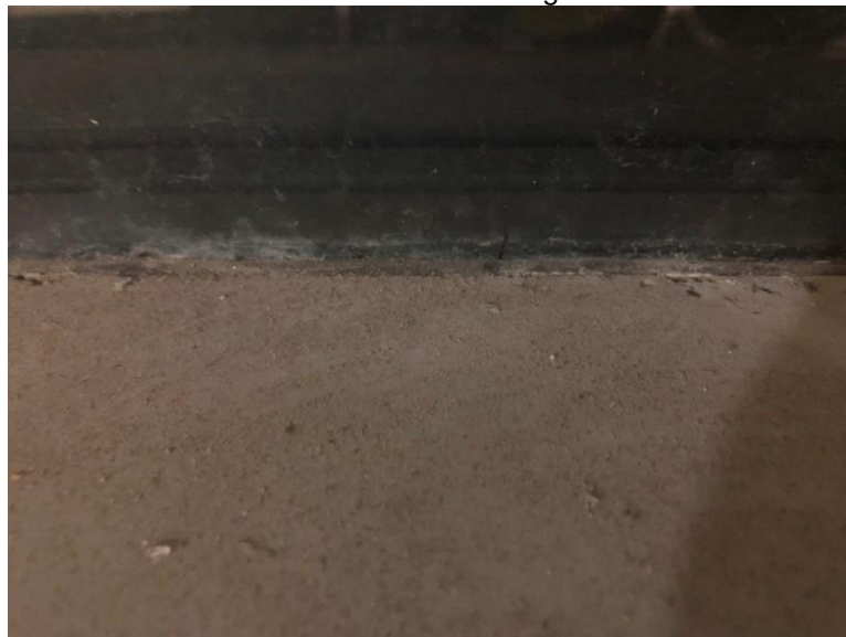
Photograph 3.3.2.1-2: Typical example of dry and stiff interior gasket and desiccant residue on interior surface of lite indicating sealed unit failure
