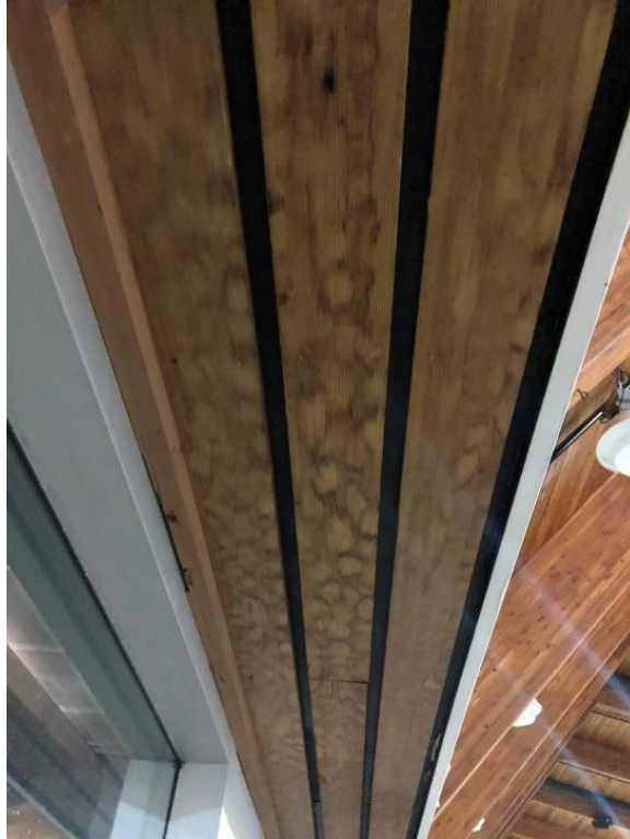
Photograph 3.3.2.1-4: Typical example of condensation and water staining on the aluminum frames and surrounding surfaces.
