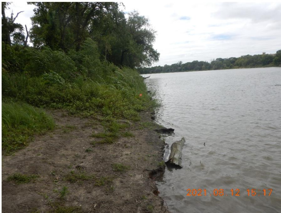
The west side of the riverbank is approximately 10 m high with a bench at approximate the normal summer water level (El. 222.5 m). The slope of the riverbank above to the bench was at a slope of approximately 4H:1V and the lower slope to the channel was approximately 5H:1V. The riverbank slope flattens
