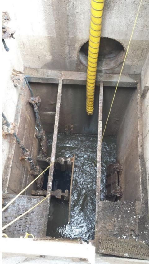
**Figure 5 – Upstream (east) siphon chamber. Note photo predates tie in to newly installed 1800 interceptor.**
