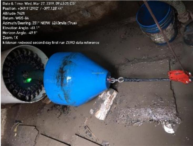
Figure 12. Chimera with trailing pig loaded into the pipe in the East Chamber.
