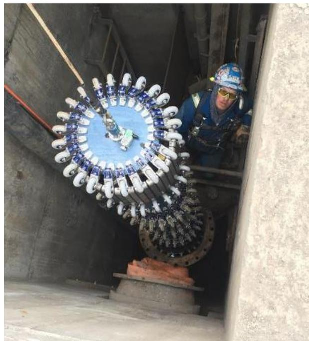
Figure 6. Chimera tool being lowered into the chamber on the west side of the river crossing
