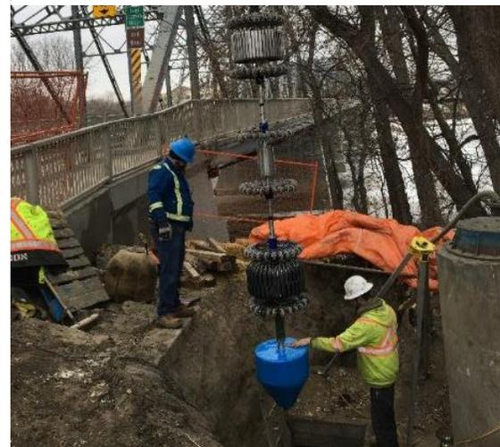
Figure 11. Chimera tool being lowered into East Chamber to inspect the horizontal portion of the Feeder Main.
