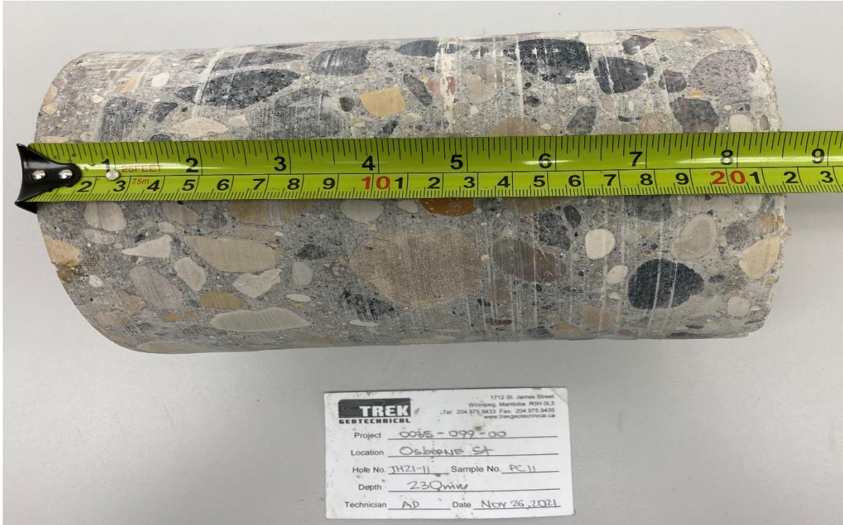
Photo 11: Pavement Core Sample at Test Hole TH21-11
