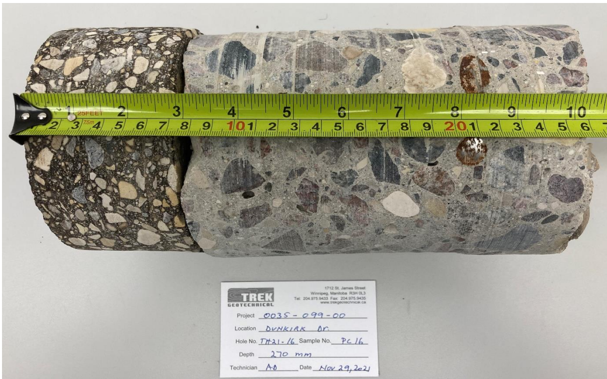
Photo 16: Pavement Core Sample at Test Hole TH21-16
