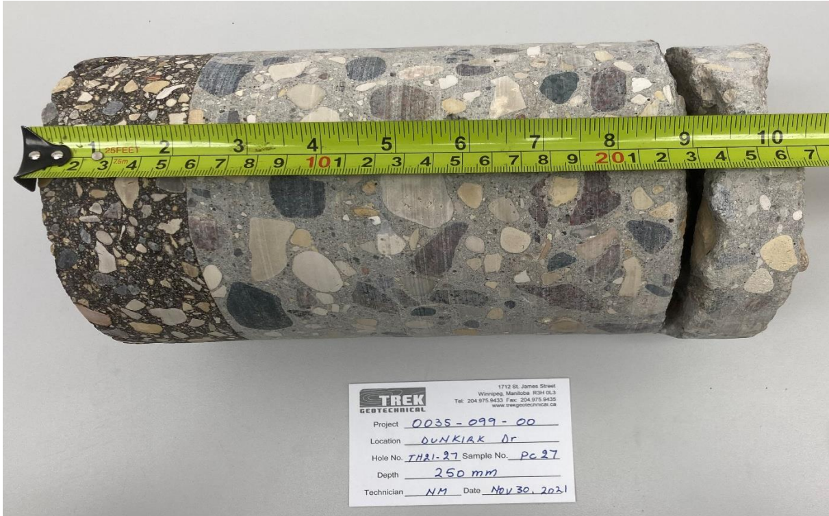
Photo 27: Pavement Core Sample at Test Hole TH21-27
