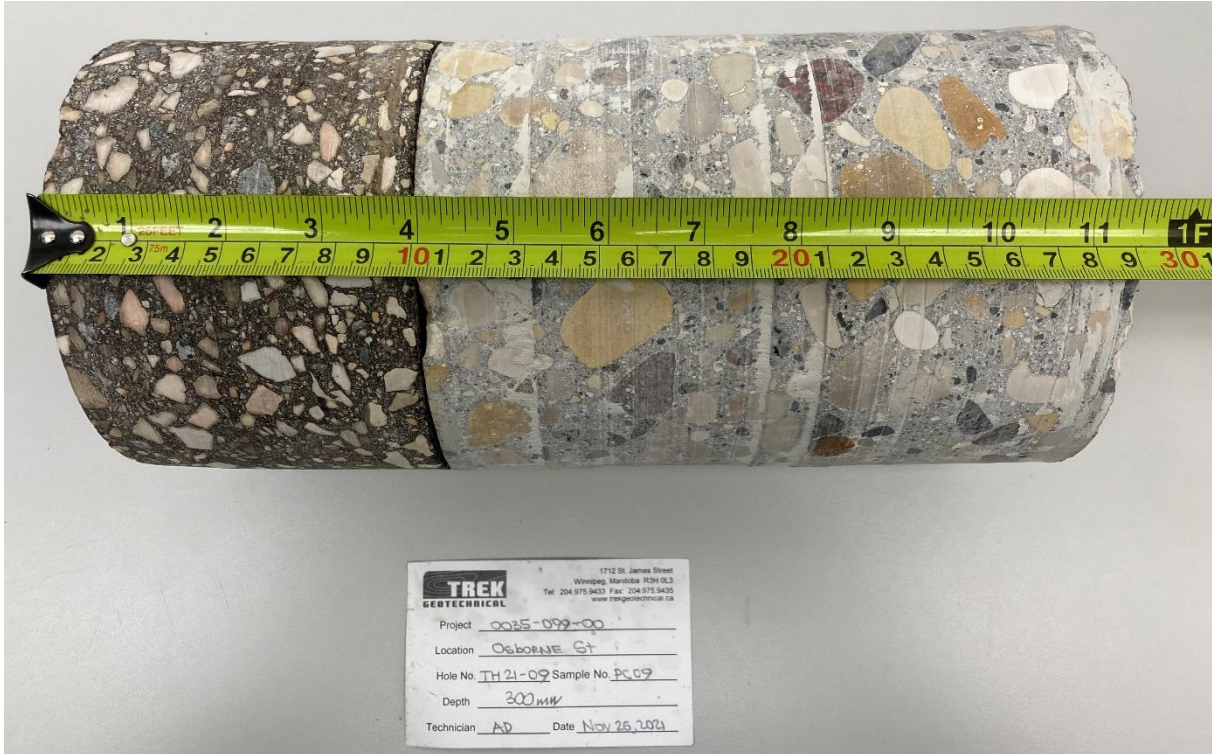
Photo 9: Pavement Core Sample at Test Hole TH21-09
