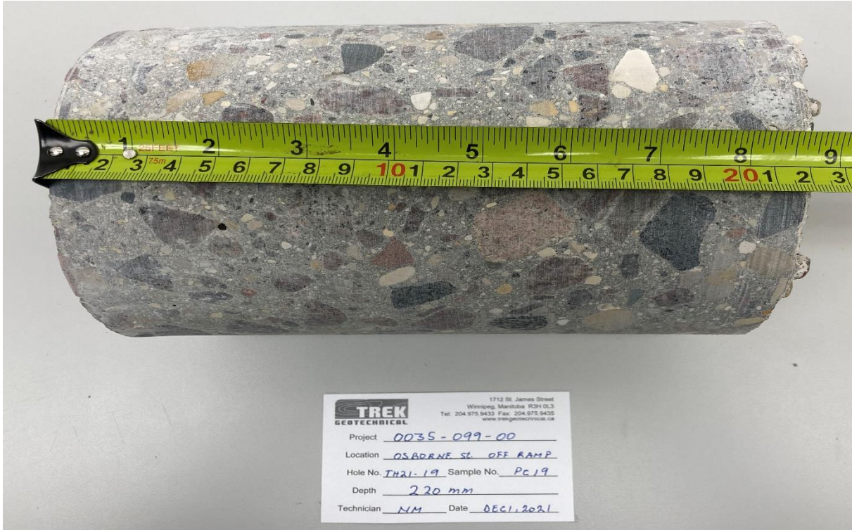
Photo 19: Pavement Core Sample at Test Hole TH21-19
