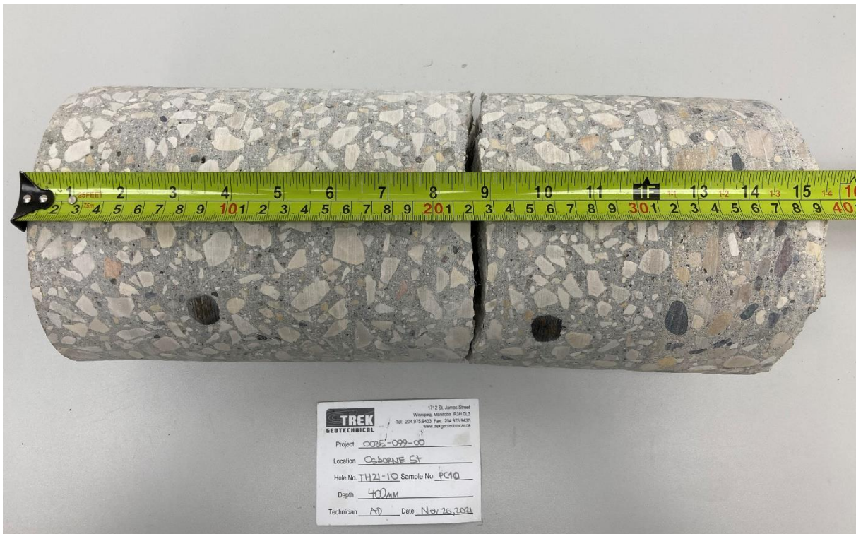
Photo 10: Pavement Core Sample at Test Hole TH21-10
