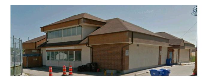
**Figure 1: North Elevation:**Remove & replace all T&G siding. Save trough & down-pipe for re-installation.
