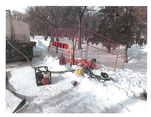
Photo 3 - Preparing to begin filling pipe at upstream valve chamber in Fraser's Grove Park
