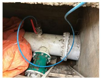
Photo 1 - McDougall's hose connected to 75 mm blow-off in east chamber
