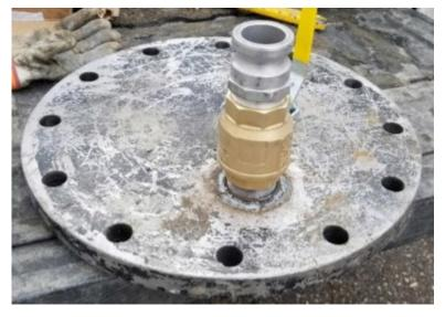
Photo 1 - Blind flanges with ball valves already installed on both ends of force main
