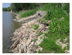
Figure 12 – Rip rap erosion protection at river bank toe.
