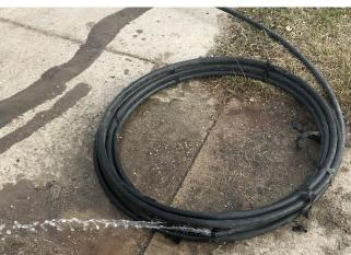
Photo 2 - Water observed flowing from hose connected to 75 mm blow-off in east chamber after flushing air (prior to connecting to pressure testing trailer)
