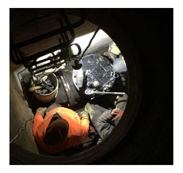
Figure 23: Newton Ave Force Main – Rotated Tee to Facilitate Inspection
