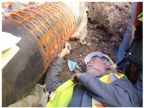
Figure A 18 - UT Inspection of 400mm Iron Pipe.
