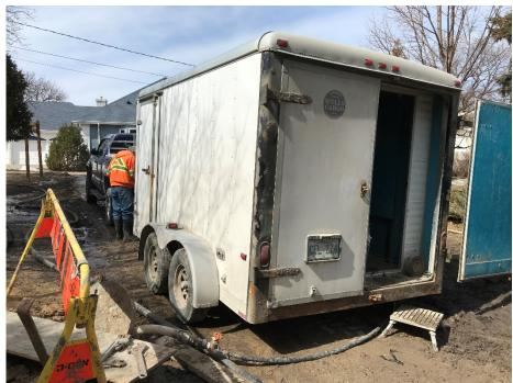
Photo 1 - McDougall's pressure testing trailer connected to 50 mm blow-off in south chamber
