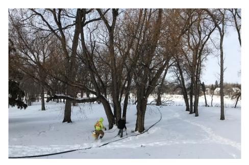
Photo 2 - Setting up water pump and thawing hoses
