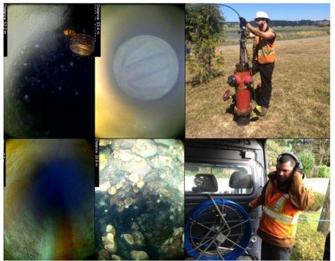
Figure A 14 - Investigator Leak Detection System (courtesy of GAME).
