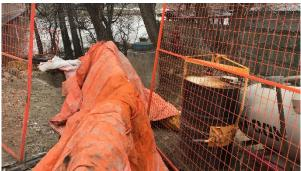
Photo 2 - Hoarded hoses connecting McDougall pressure testing trailer to 75 mm blow-off on east chamber cross piece
