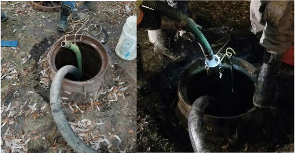
Figure 3: The standpipe configuration with 4" reducer after switching hoses.
