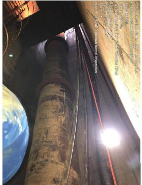
Figure 10. Looking up vertical shaft from tunnel. Image shows the vertical steel pipe portion of the Kildonan-Redwood Feeder Main.
