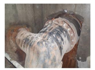
Figure 3: Site 1 - Side Outlet 90 Deg Elbow (West Tunnel Shaft)
