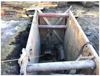
Figure 7. Tagline being pulled up at north excavation to pull south side winchline through the Feeder Main.
