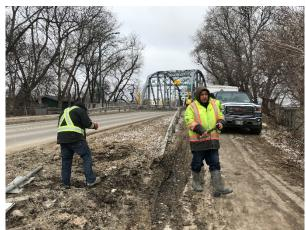
Photo 1 - McDougall operating new 300 mm valve to charge pipe to city pressure
