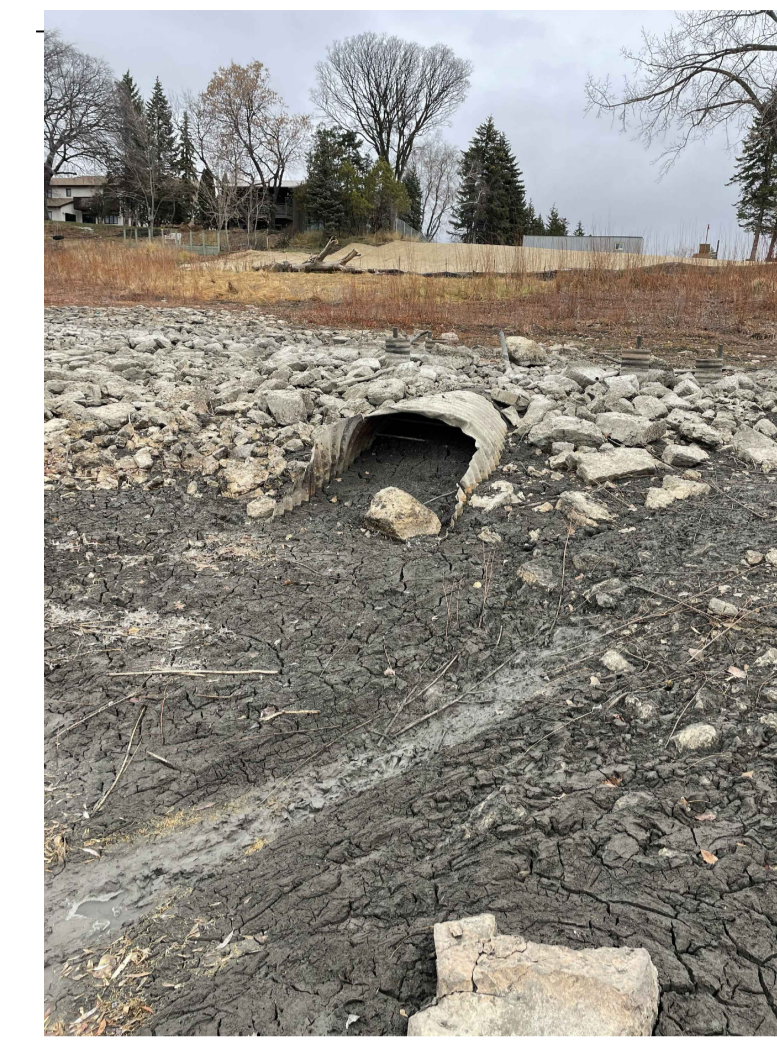
PIPE OUTLET DATE: 2022-11
