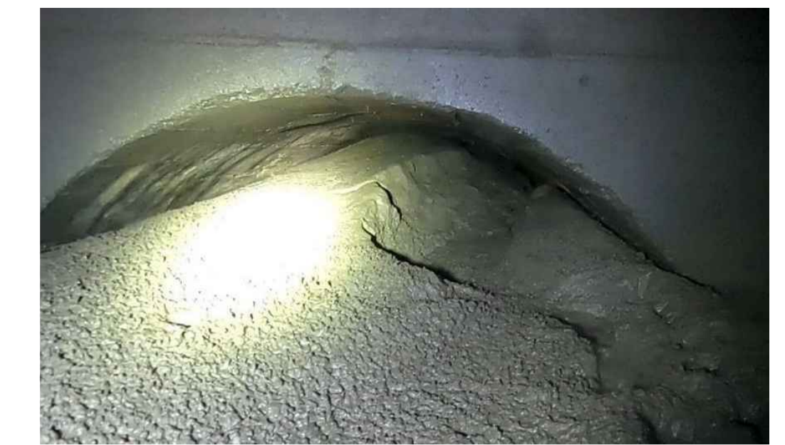
INSIDE CHAMBER LOOKING DOWNSTREAM INTO OUTFALL DATE: 2022-11
