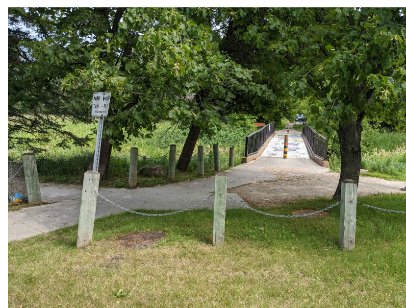
LOOKING NORTH DATE: 2022-07
