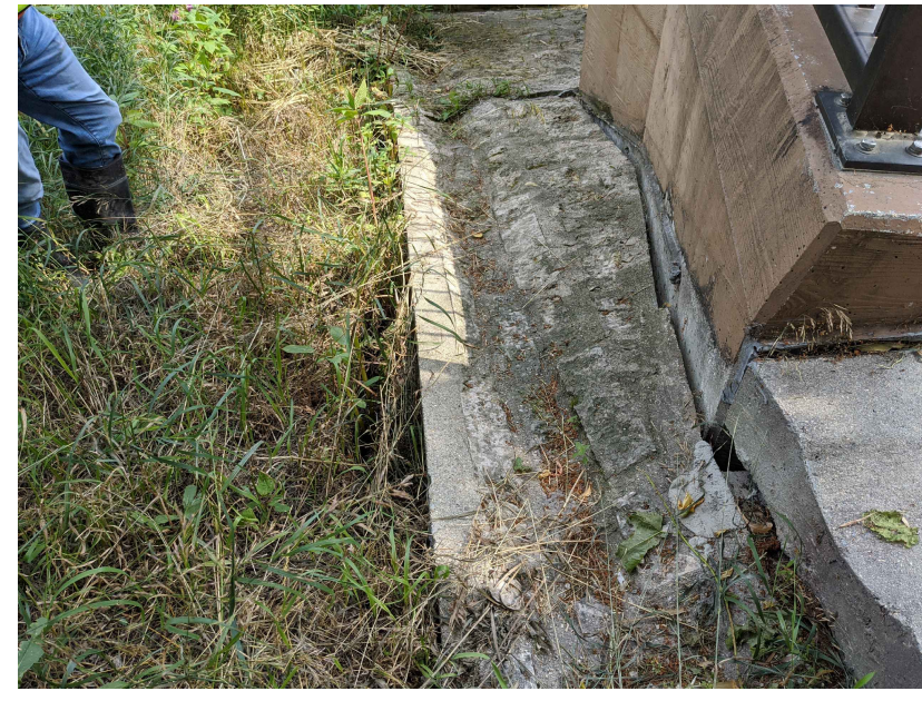
SW BRIDGE CORNER DATE: 2022-07
