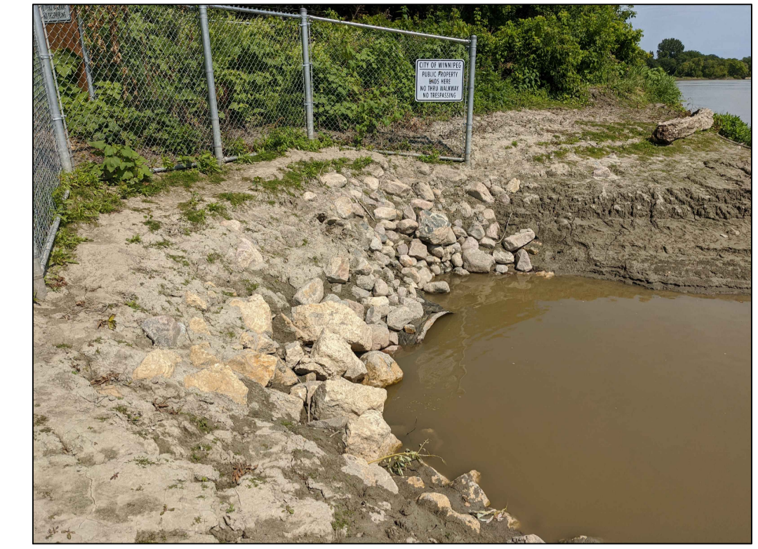
PIPE OUTLET DATE: 2022-07
