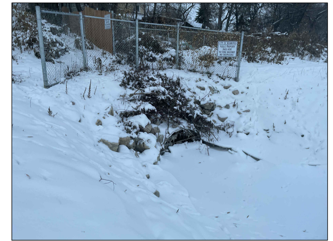
PIPE OUTLET DATE: 2022-11
