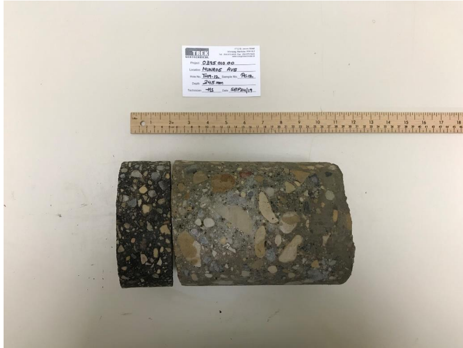
Photo 12: Pavement Core Sample at Test Hole TH19-12
