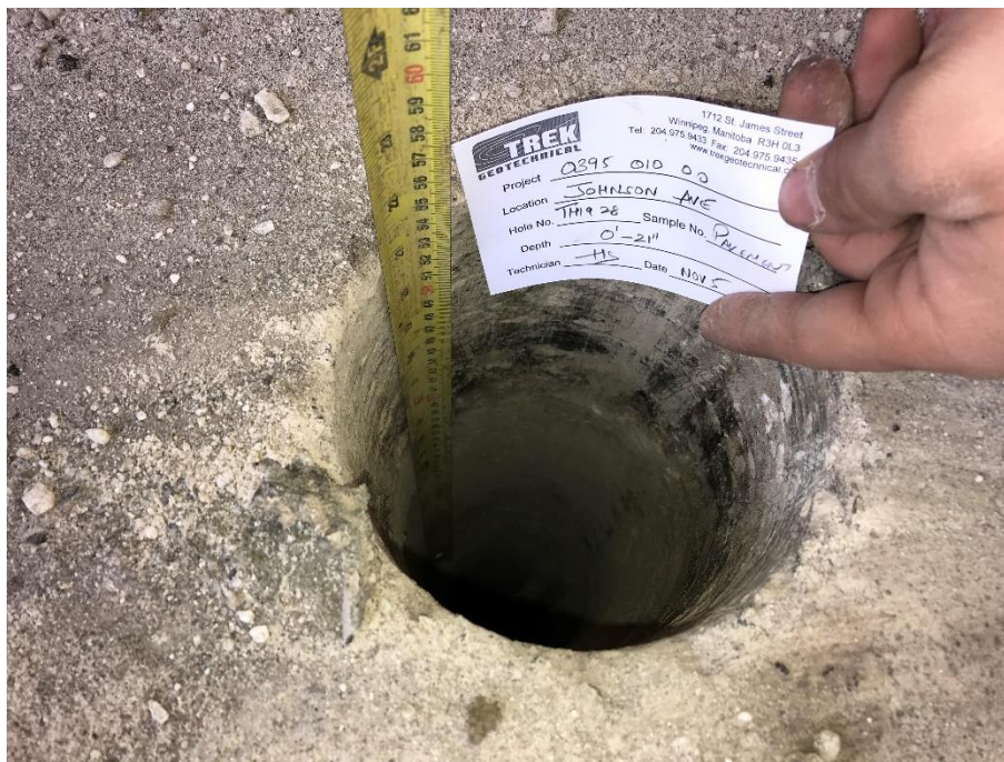
Photo 28: Pavement Core Measurement at Test Hole TH19-28
