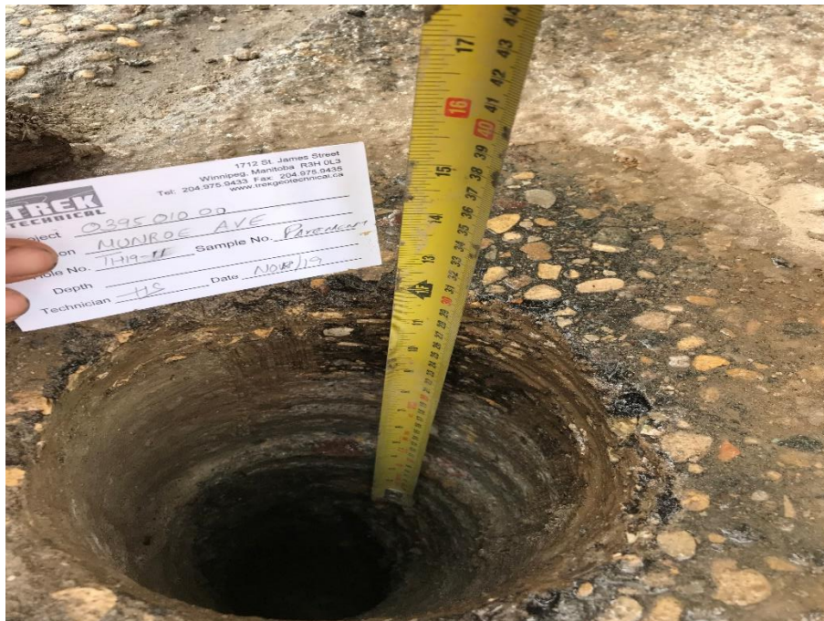
Photo 11: Pavement Core Measurement at Test Hole TH19-11
