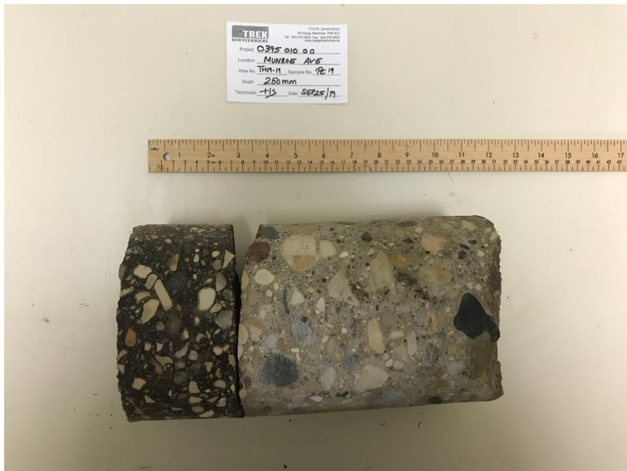
Photo 19: Pavement Core Sample at Test Hole TH19-19
