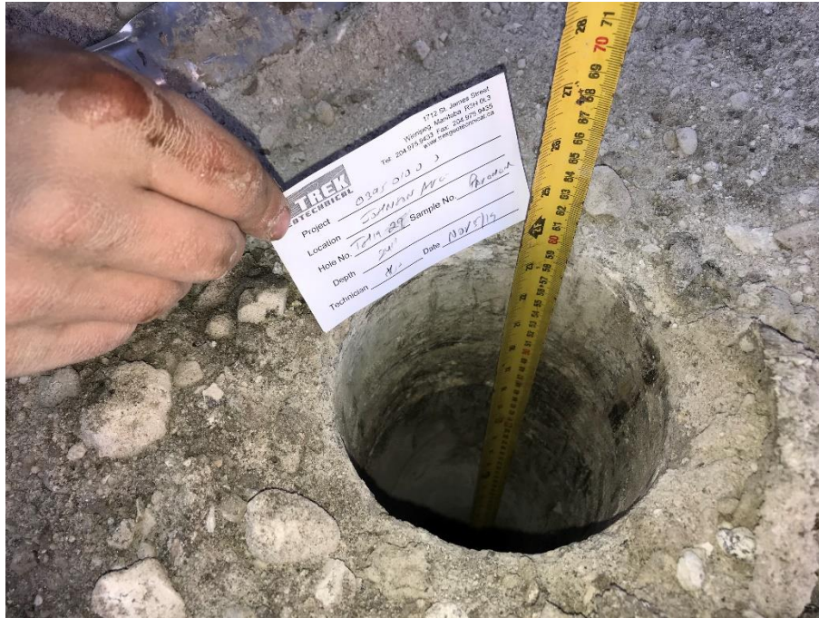
Photo 29: Pavement Core Measurement at Test Hole TH19-29
