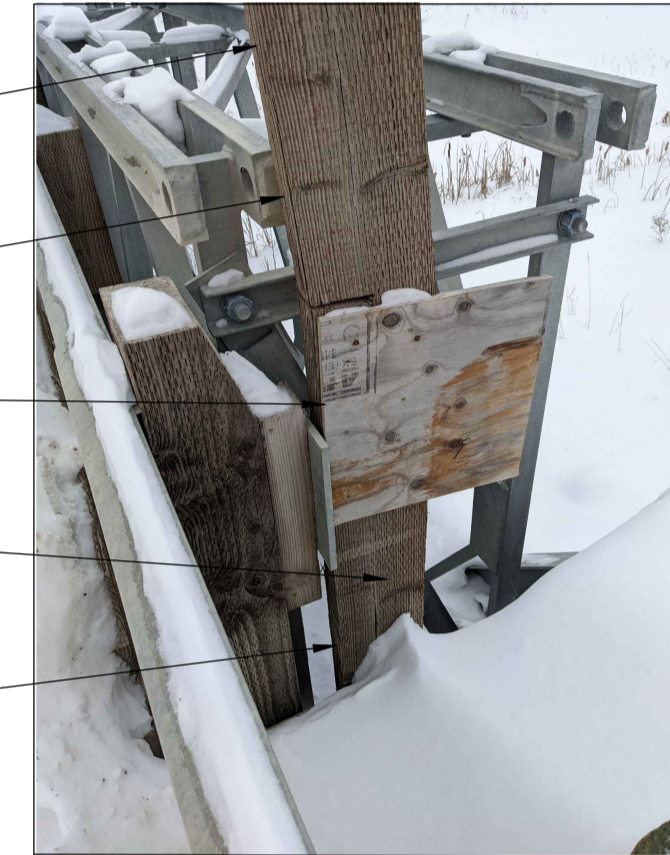
HAZARD MARKER INSTALLATION
