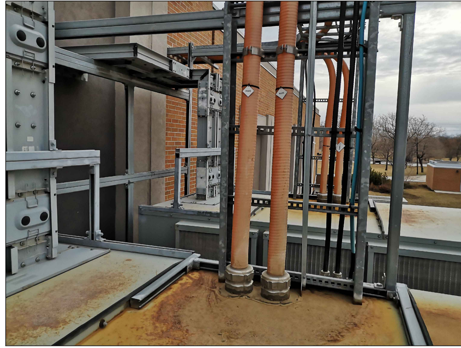
UVT-3 (FOREGROUND) AND UVT-2 (BACKGROUND) EXISTING ROOF
