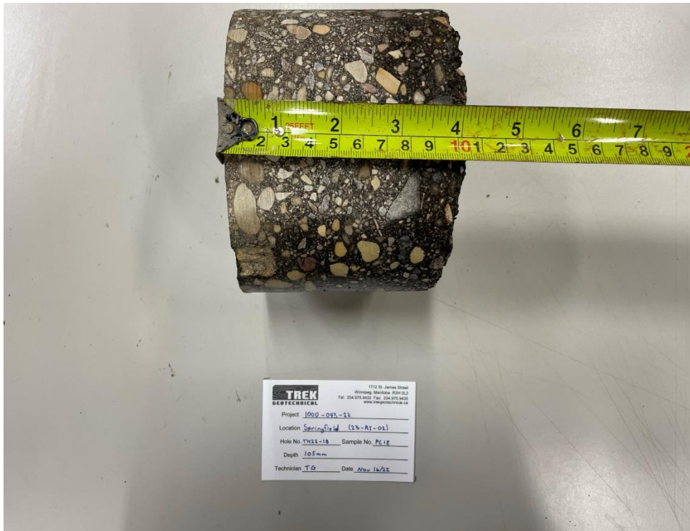
Photo 2: Pavement Core Sample at TH22-18
