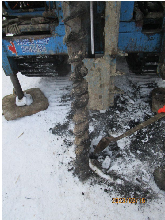
TH23-07 Photo 1: 0 ft to 5 ft (0 m to 1.52 m)
