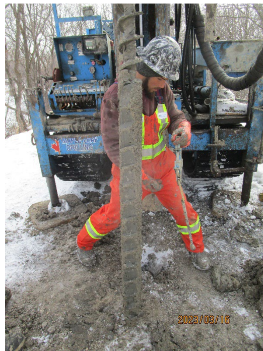
TH23-07 Photo 12: 55 ft to 60 ft (16.76 m to 18.29 m)
