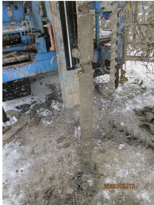
TH23-07 Photo 11: 50 ft to 55 ft (15.24 m to 16.76 m)
