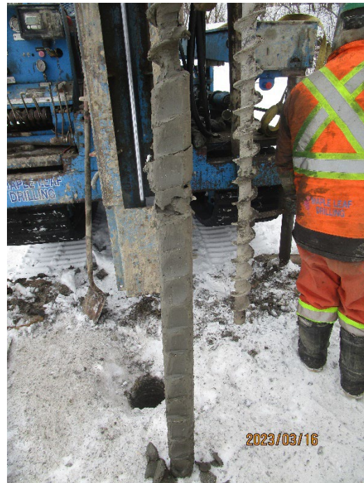
TH23-08 Photo 10: 45 ft to 50 ft (13.72 m to 15.24 m)
