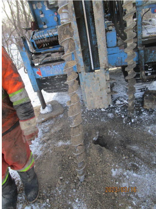
TH23-07 Photo 5: 20 ft to 25 ft (6.1 m to 7.62 m)
