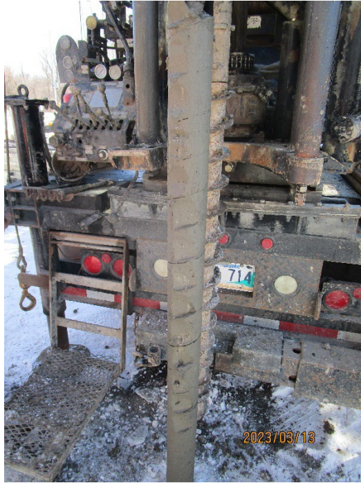
TH23-02 Photo 11: 50 ft to 55 ft (15.24 m to 16.76 m)
