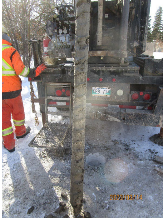
TH23-03 Photo 13: 61 ft to 66 ft (18.60 m to 20.12 m)
