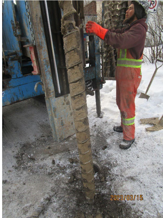
TH23-05 Photo 3: 10 ft to 15 ft (3.05 m to 4.57 m)
