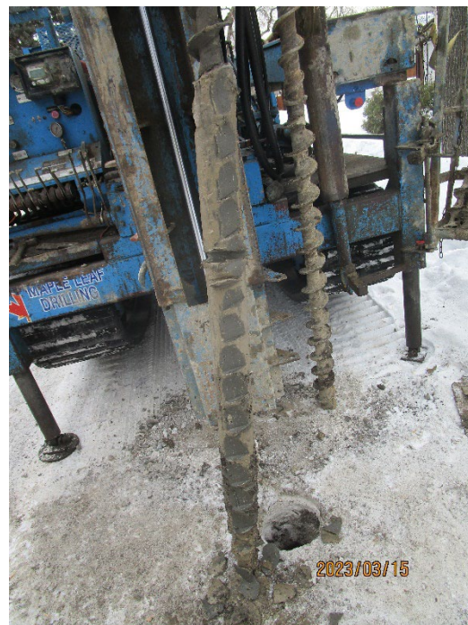
TH23-05 Photo 8: 35 ft to 40 ft (9.14 m to 12.19 m)
