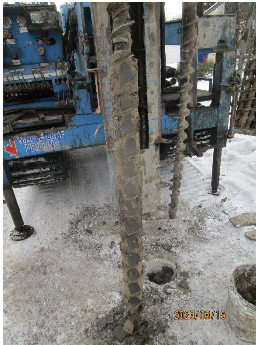
TH23-05 Photo 6: 25 ft to 30 ft (7.62 m to 9.14 m)
