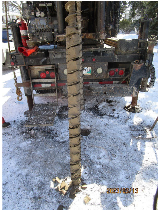
TH23-02 Photo 5: 20 ft to 25 ft (6.1 m to 7.62 m)
