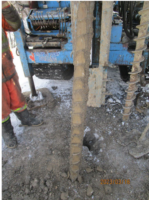
TH23-07 Photo 9: 40 ft to 45 ft (12.19 m to 13.72 m)
