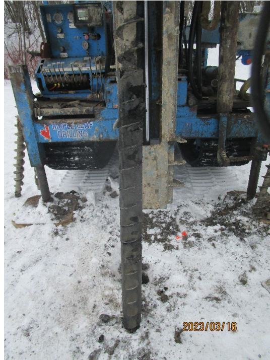
TH23-08 Photo 3: 10 ft to 15 ft (3.05 m to 4.57 m)
