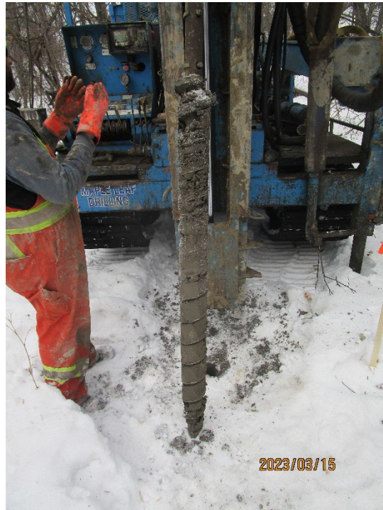
TH23-06 Photo 1: 0 ft to 5 ft (0 m to 1.52 m)
