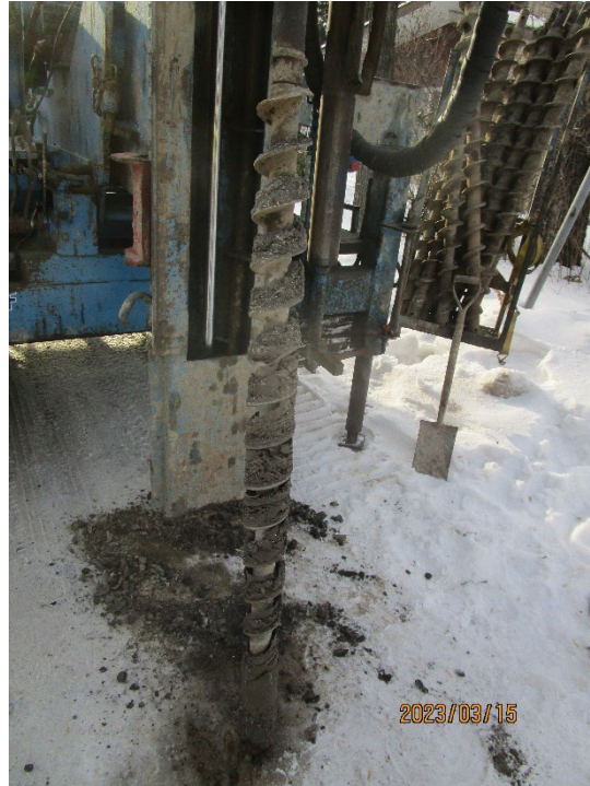
TH23-05 Photo 1: 0 ft to 5 ft (0 m to 1.52 m)
