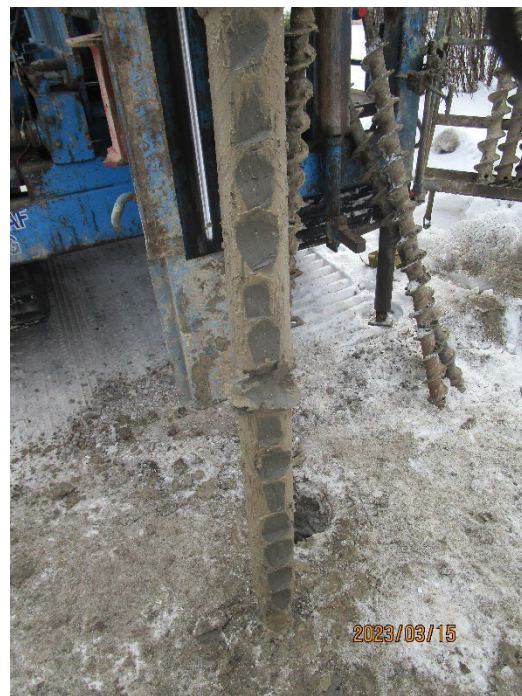
TH23-05 Photo 12: 55 ft to 60 ft (16.76 m to 18.29 m)
