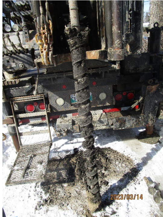
TH23-04 Photo 1: 0 ft to 5 ft (0 m to 1.52 m)
