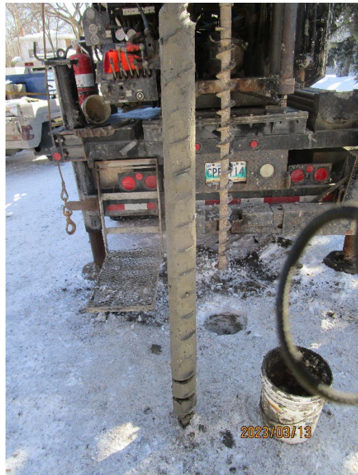
TH23-02 Photo 12: 55 ft to 60 ft (16.76 m to 18.29 m)
