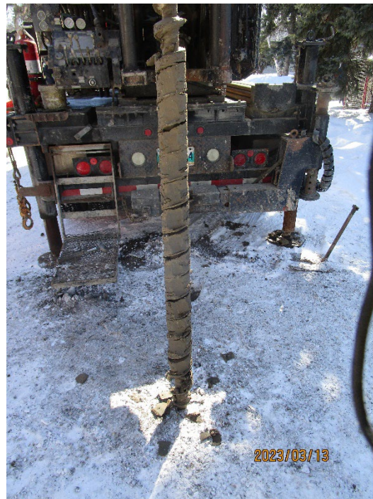
TH23-02 Photo 6: 25 ft to 30 ft (7.62 m to 9.14 m)
