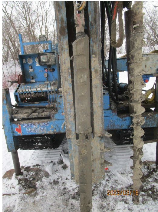
TH23-08 Photo 7: 30 ft to 35 ft (9.14 m to 10.67 m)
