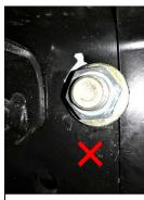
Not acceptable bolt/nut assembly, on seam
