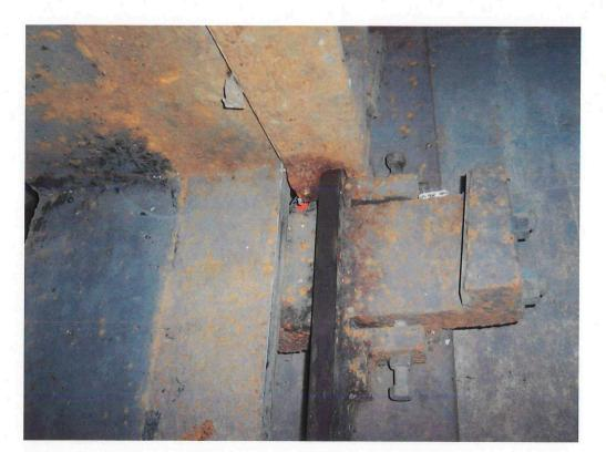
WET WELL ROOF - SPALLING WITH EXPOSED REBAR
