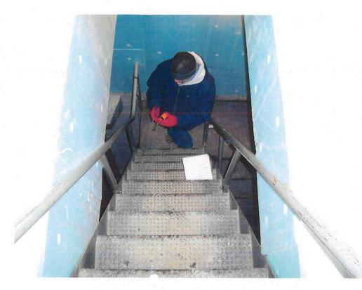
DRY WELL ACCESS STAIR - STEEP AND MISSING MID-RAILS
