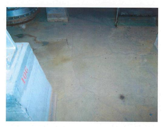
DRY WELL WALLS - WHITE DEPOSITS (EFFLORESCENCE) FROM HAIRLINE CRACKS AT CONCRETE INFILLS
