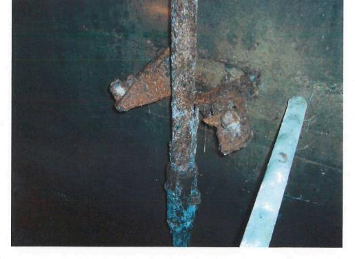
**SLIDE GATE SHAFTS AND GUIDES - CORRODED**
