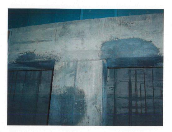
INTERMEDIATE BEAMS AND COLUMNS (DRY WELL) - MULTIPLE PATCHED LOCATIONS
