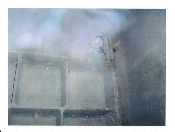
FLAP GATE - MINOR CORROSION
