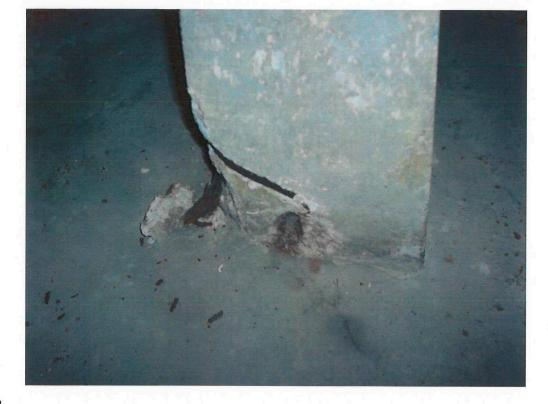
PUMP BASE - BOTTOM CORNER SPALLED OFF AND EXPOSED REINFORCING STEEL (CORRODED - SECTION LOSS)
