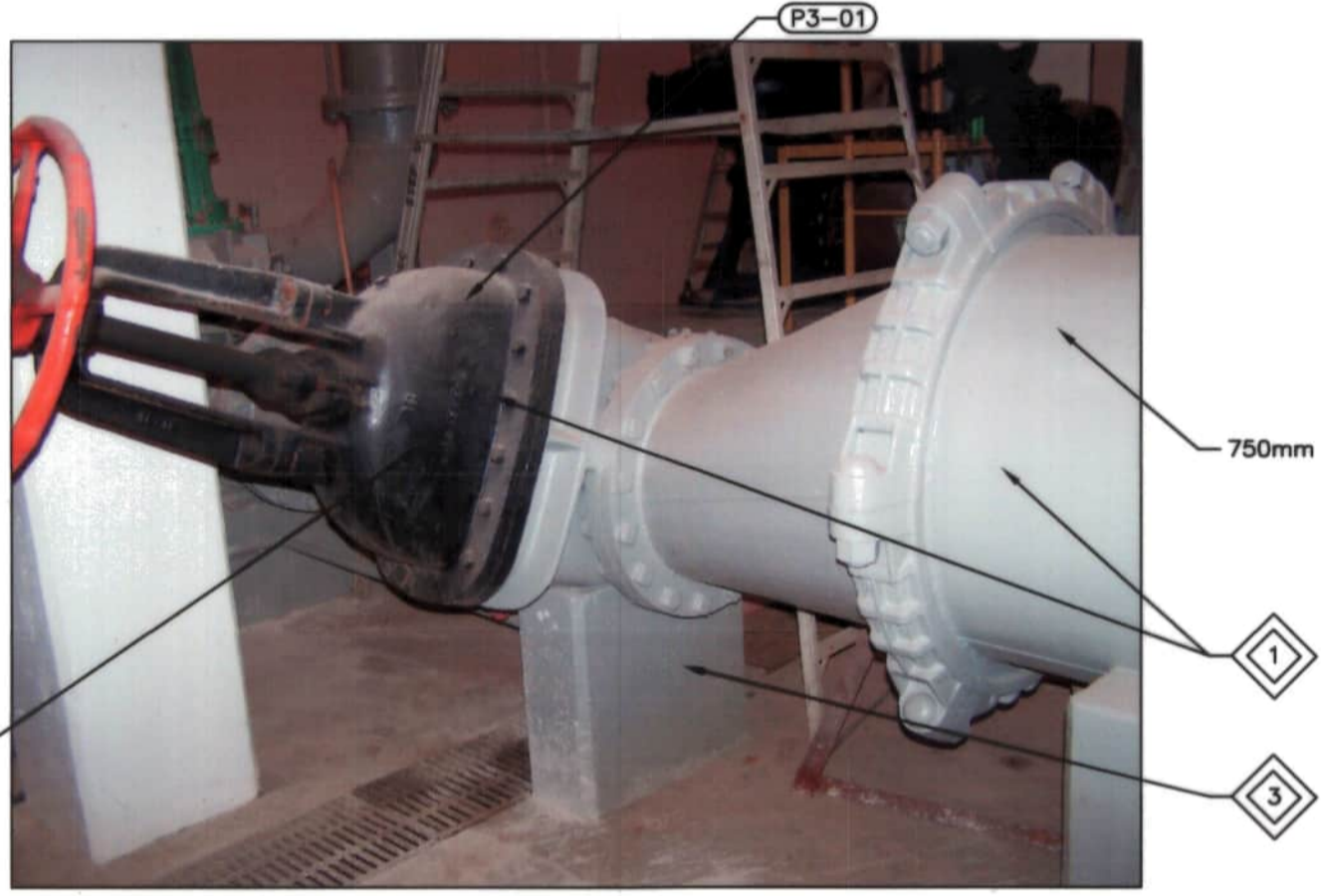
4 P3 SUCTION PIPING - LEVEL 100 M1
