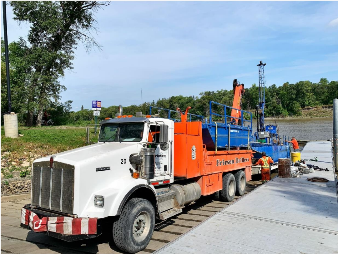
TH24-03 Barge Demobilization
