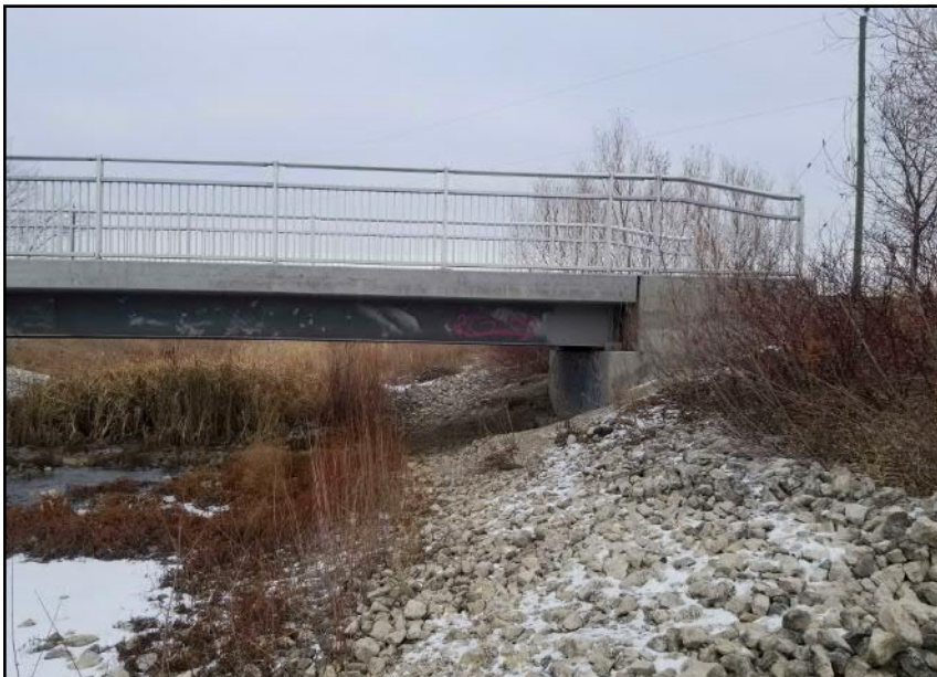
Site 9 - Eastern Bank | Rip-rap at bridge abutment north of the crossing (facing NE)
