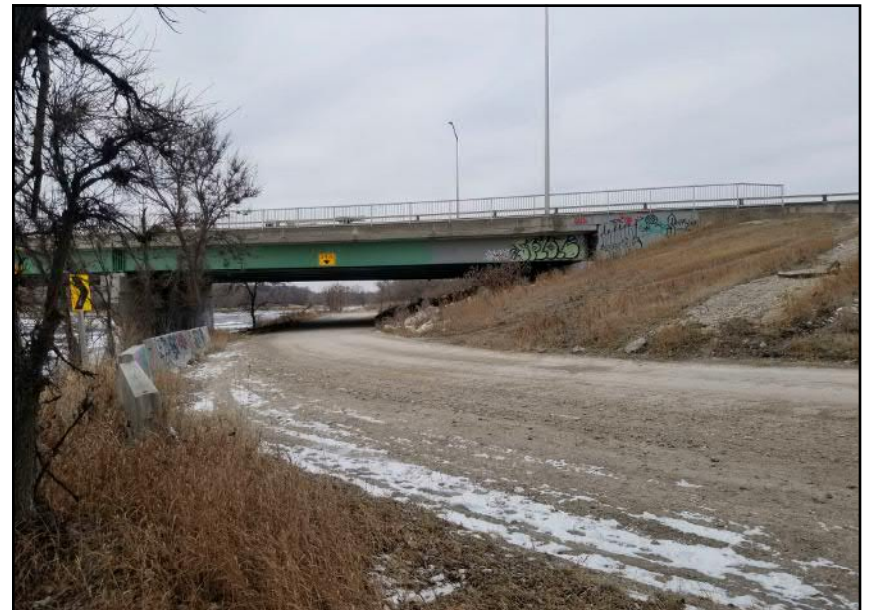
Site 5 - Northern Riverbank | Granular road along riverbank crest below bridge, jersey barriers, traffic signs (facing W)
