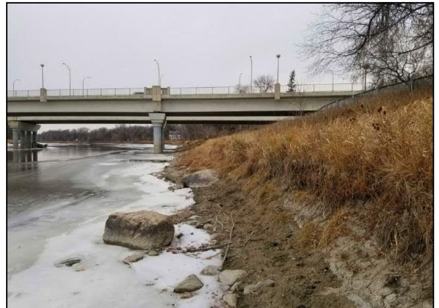
Site 10 - Northern Riverbank | Scarp near river edge observed along full length of bank toe within study area (facing W)
