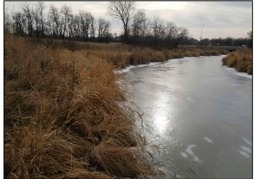
Site 6B - Eastern Bank Minor erosion observed at localized areas along bank toe (facing S)
