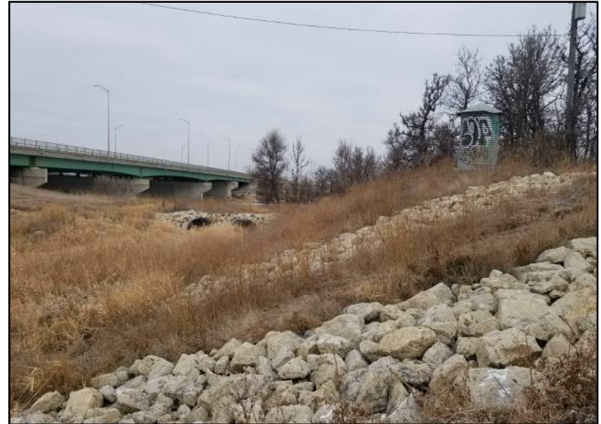
Site 5 - Southern Riverbank | Rock drains installed within steeper slopes of rip-rap lined drainage channel (facing N)
