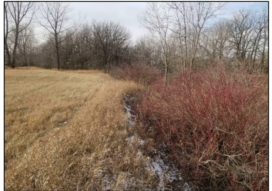
Site 6A - Southern Bank | Progressive slope instabilities have progressed towards the bank crest (facing W)
