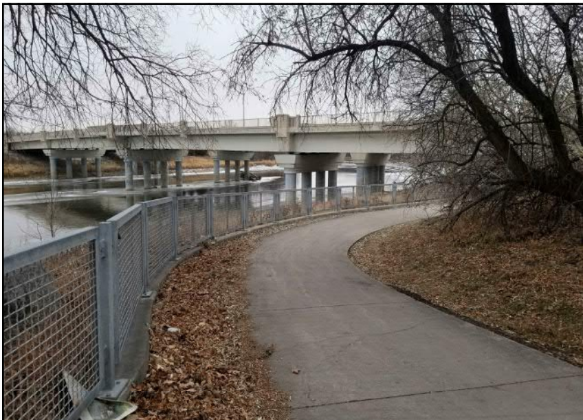
Site 10 - Northern Riverbank | Pedestrian pathway with minor cracking and railing along bank slope (facing SW)
