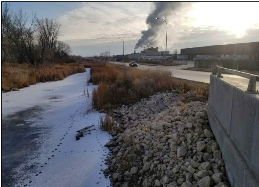
Site 8 - Western Bank | Regraded and rip-rap armoured slope within crossing alignment (facing S)
