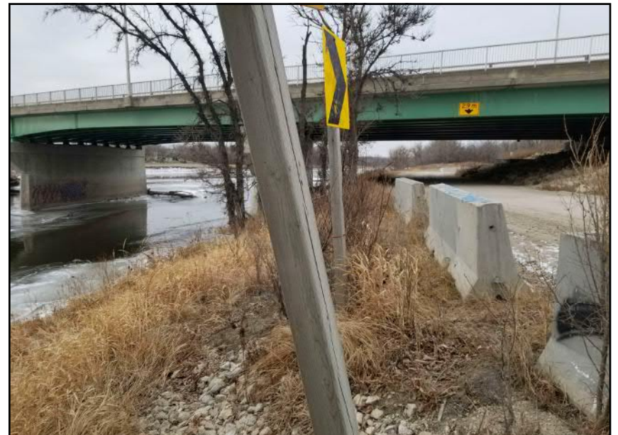
Site 5 - Northern Riverbank Traffic signs located along bank crest near crossing alignment. One leaning, one straight (facing W)
