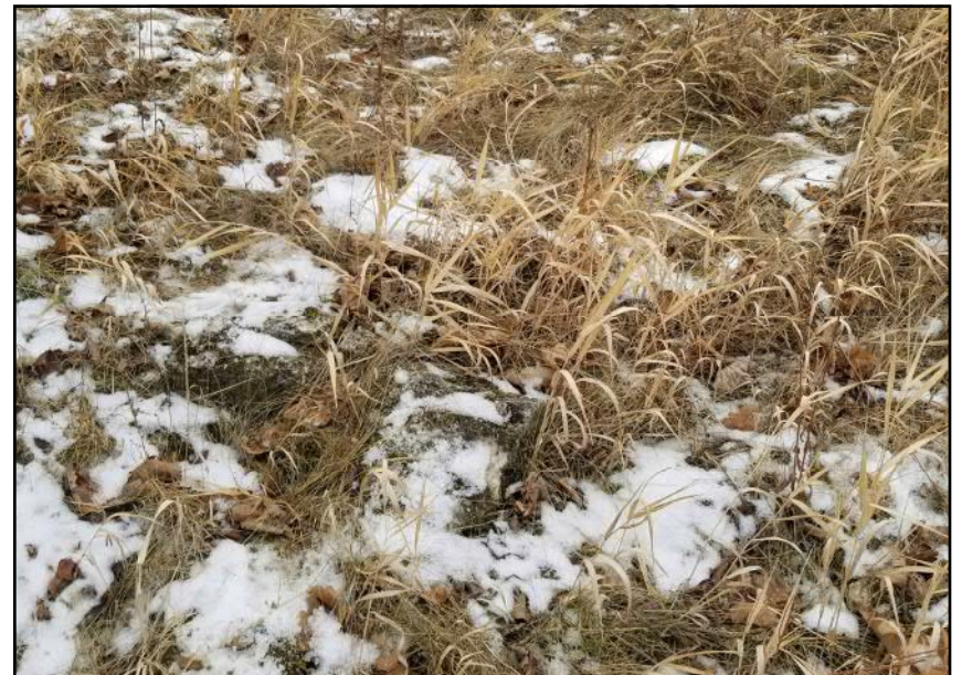
Site 10 - Southern Riverbank Small scarp and crack observed along flat portion of bank crest near crossing alignment (facing S)
