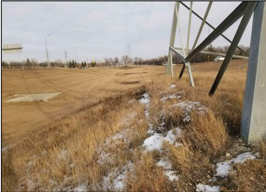
Site 4 - Eastern Riverbank Steeper slopes around hydro tower showed signs of slope instability and animal burrows (facing E)
