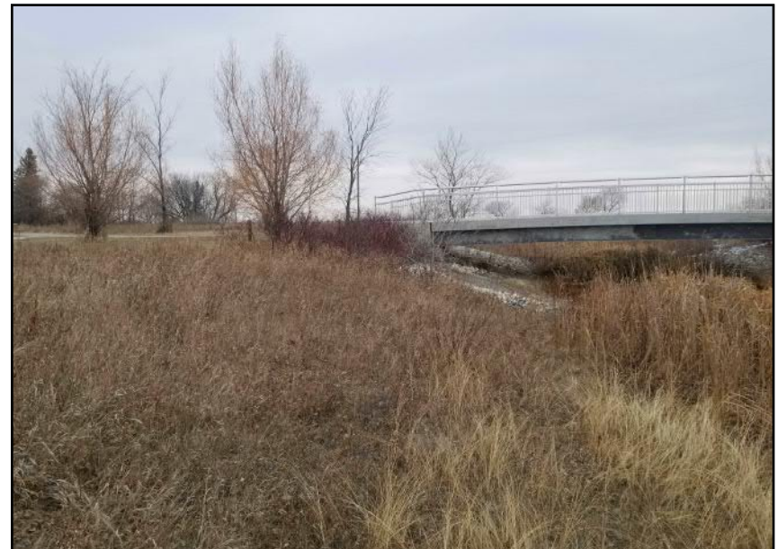
Site 9 - Western Bank Moderate to dense brush vegetation along bank slope, groundwater well near bridge (facing N)
