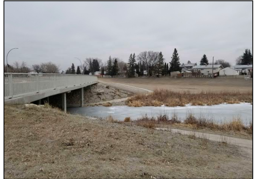
Site 7 - Western Bank | View from the west bank facing the east bank along the approximate crossing alignment (facing E)
