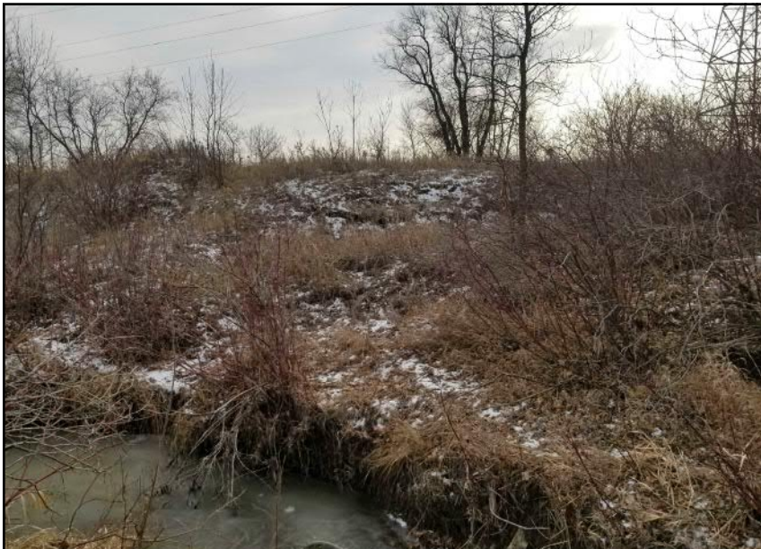
Site 6A - Southern Bank Progressive slope instabilities along bank slope near crossing alignment (facing SE)
