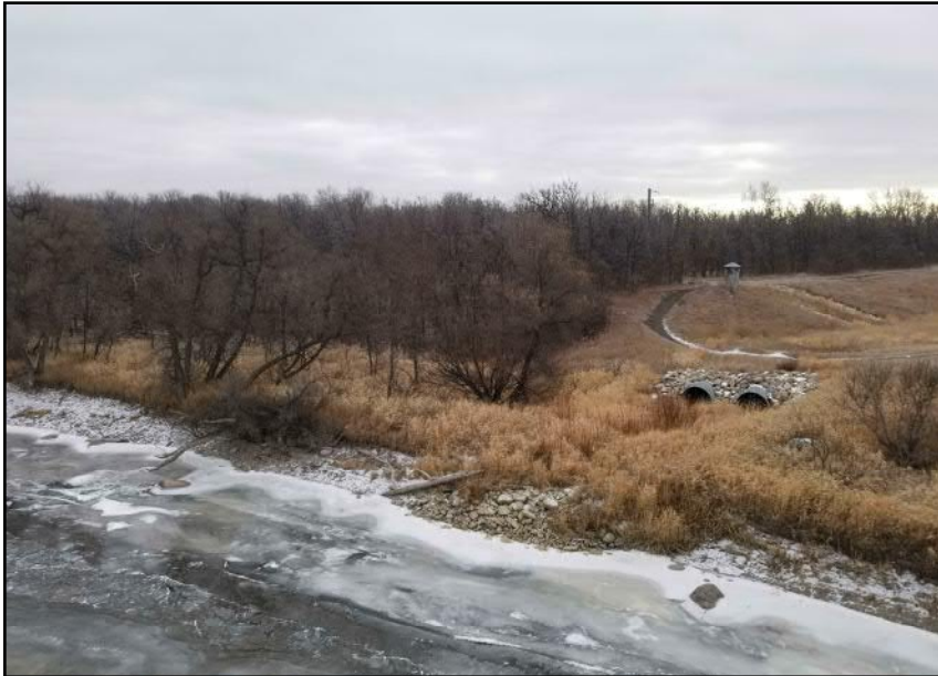
Site 5 - Southern Riverbank | View of southern bank from top of bridge (facing SE)
