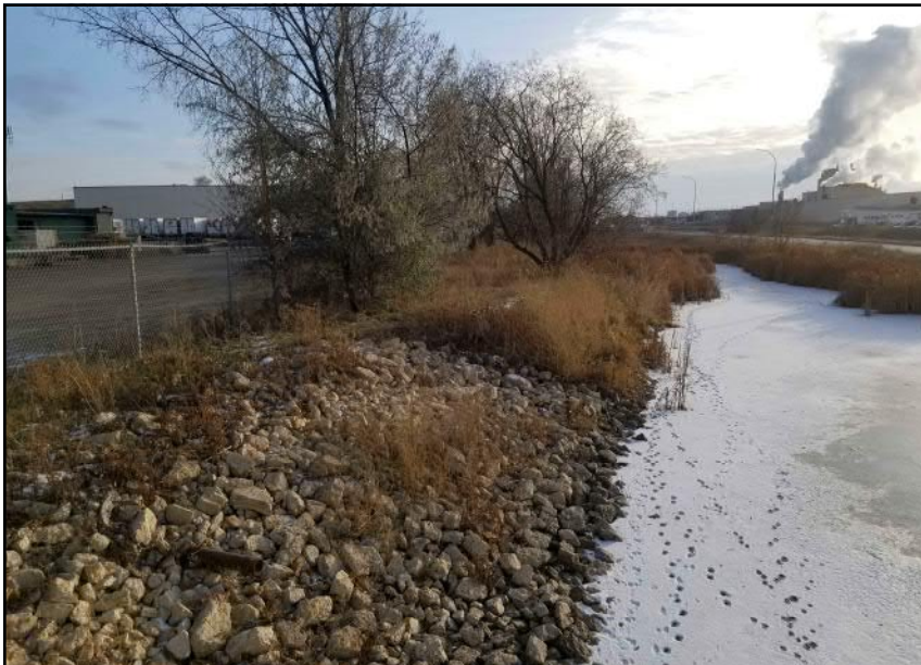
Site 8 - Eastern Bank | Regraded and rip-rap armored slope within crossing alignment (facing S)
