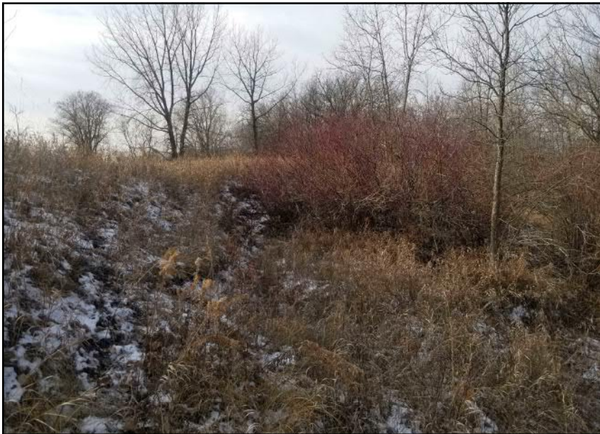
Site 6A - Southern Bank | Progressive slope instabilities observed in close proximity to crossing alignment (facing W)
