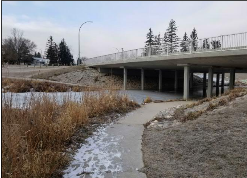
Site 7 - Eastern Bank Steeper slopes to the east of pedestrian pathway, gradual slope to the west of it (facing NW)
