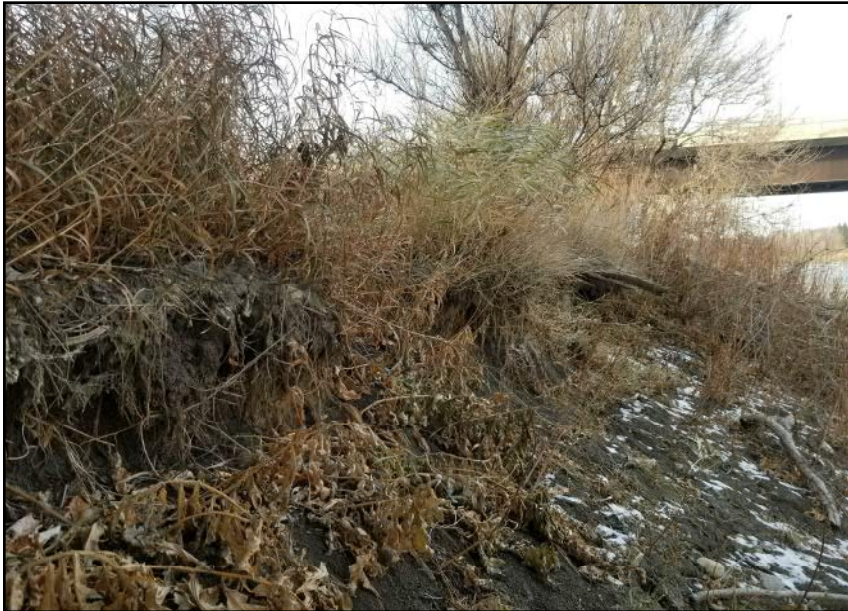
Site 4 - Western Riverbank | Observed scarp near oversteepened riverbank crest in adjacent to crossing alignment (facing N)
