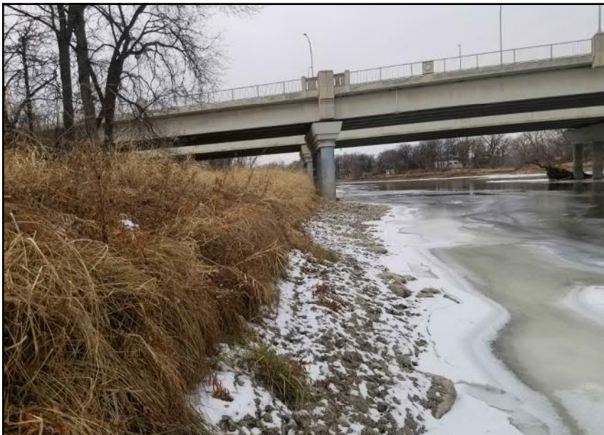
Site 10 - Southern Riverbank Scarp near river edge observed within western portion of study area (facing W)
