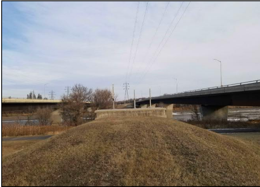
Site 4 - Western Riverbank | Steepened slopes around siphons inlet chamber structure (facing E)
