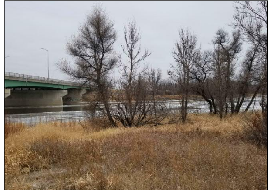
Site 5 - Southern Riverbank View from riverbank crest along approximate crossing alignment (facing N)
