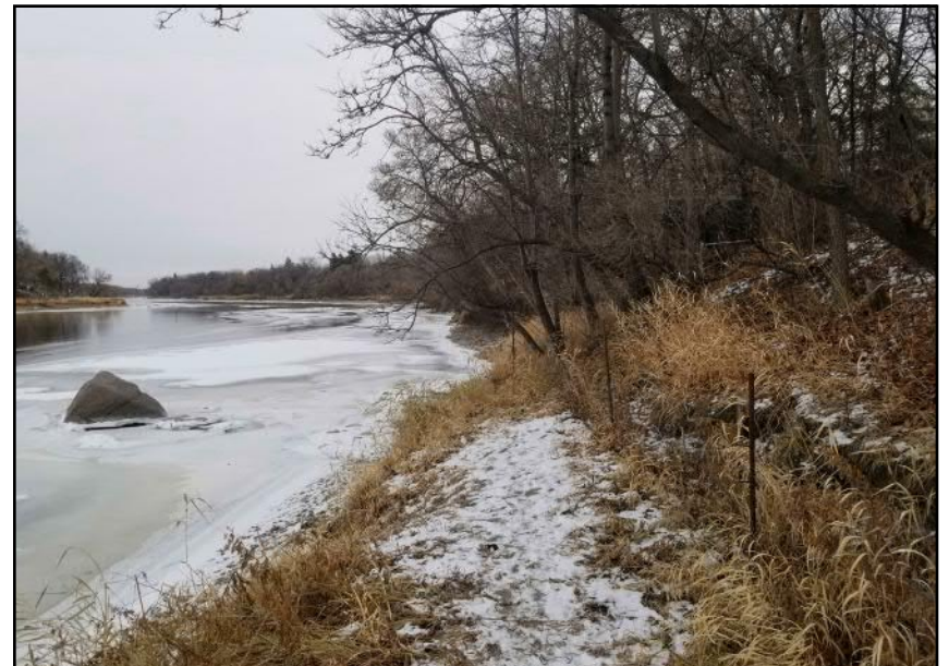
Site 10 - Southern Riverbank | Oversteepened banks and instabilities observed within eastern portion of study area (facing E)
