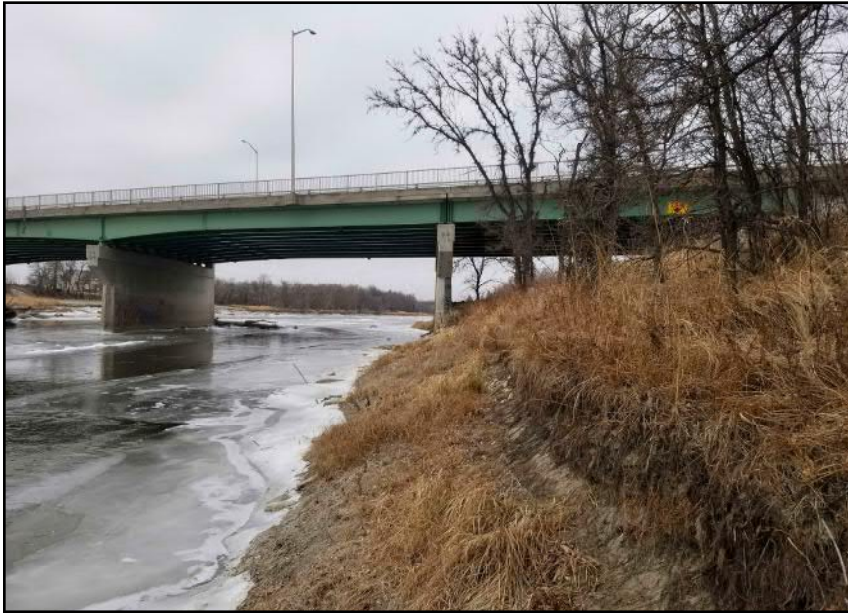
Site 5 - Northern Riverbank Erosion scarp observed near bank toe within western portion of study area (facing W)
