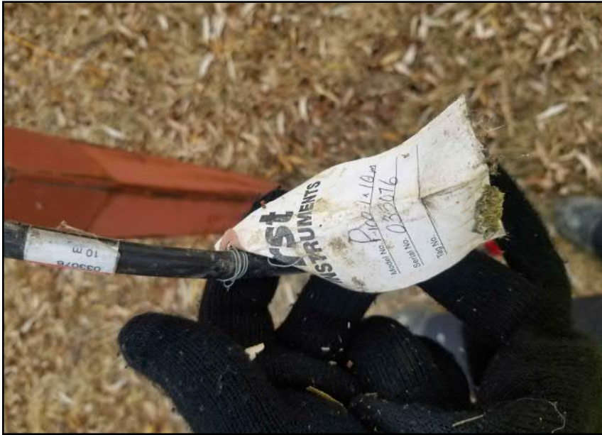
Site 9 - Western Bank Groundwater well near west bridge abutment containing pneumatic piezometer
