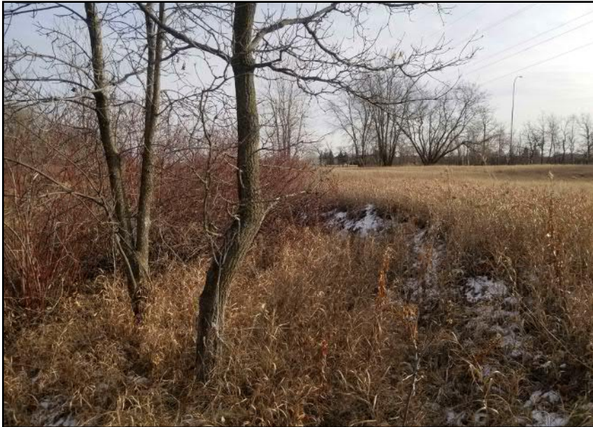
Site 6A - Southern Bank Progressive slope instabilities have progressed towards the bank crest (facing E)
