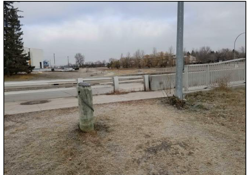
Site 7 - Western Bank | Western bridge abutment near bank crest (facing N)
