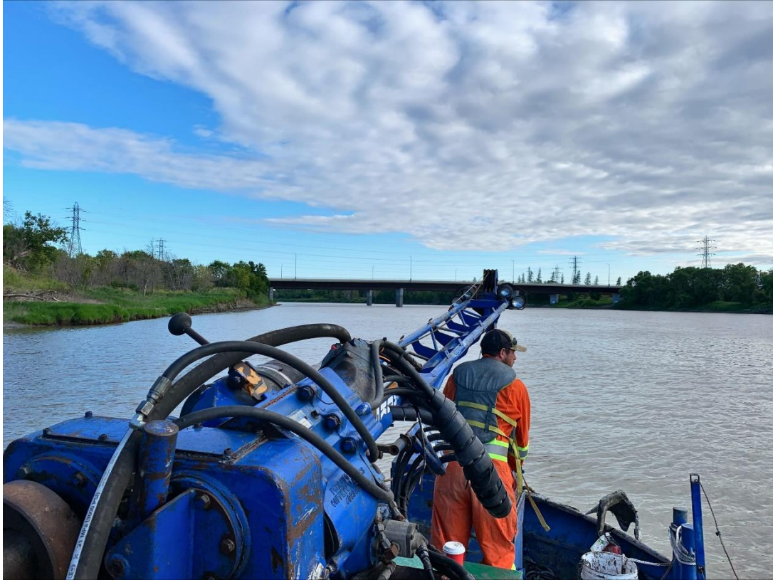
TH24-03 Barge Launch
