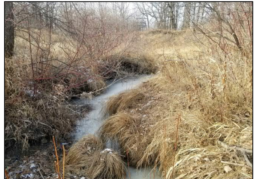
Site 6A - Northern Bank Erosion scarp observed along drain edges, varying in height (facing W)
