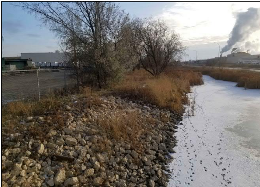
Site 8 - Eastern Bank Regraded and rip-rap armoured slope within crossing alignment (facing S)
