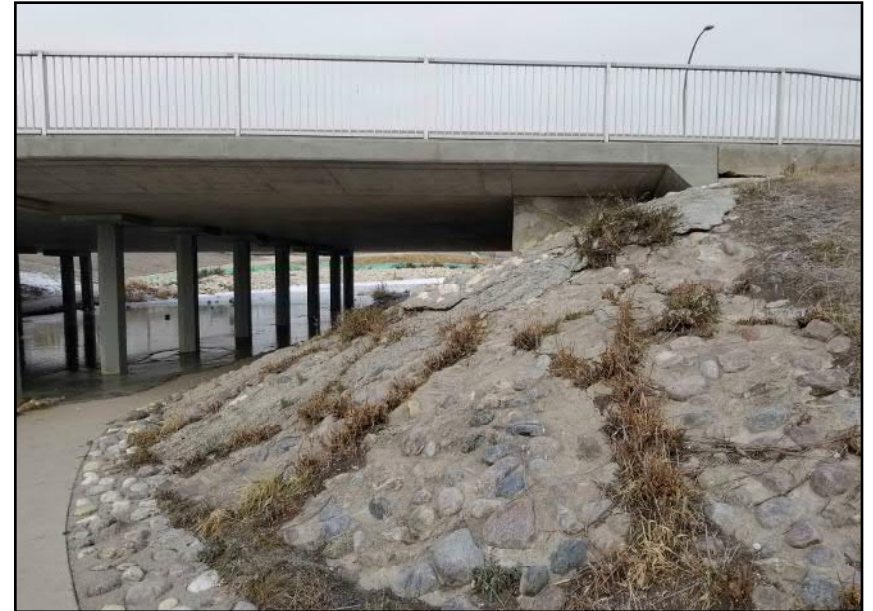
Site 7 - Eastern Bank Grouted rip-rap armouring along steeper banks in close proximity to bridge abutment (facing N)
