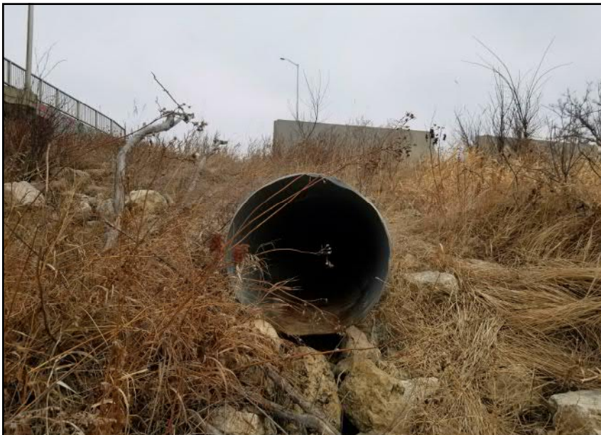
Site 5 - Northern Riverbank CSP outfall daylighting along bank slope, some erosion of bank material between rip-rap (facing N)
