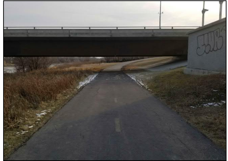
Site 4 - Western Riverbank Asphalt paved pedestrian pathway. Minor cracking observed parallel to bank crest (facing S)
