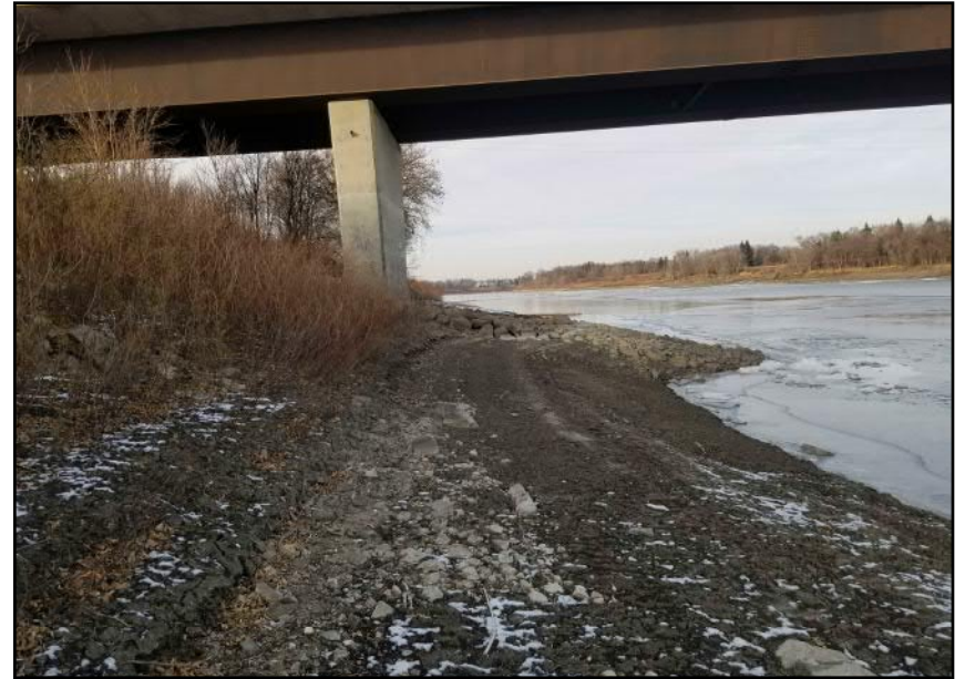
Site 4 - Western Riverbank Short erosion scarps, localized rip-rap, gradual toe slope within crossing alignment (facing N)
