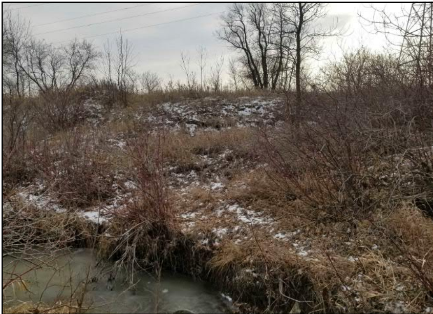
Site 6A - Southern Bank Progressive slope instabilities along bank slope near crossing alignment (facing SE)
