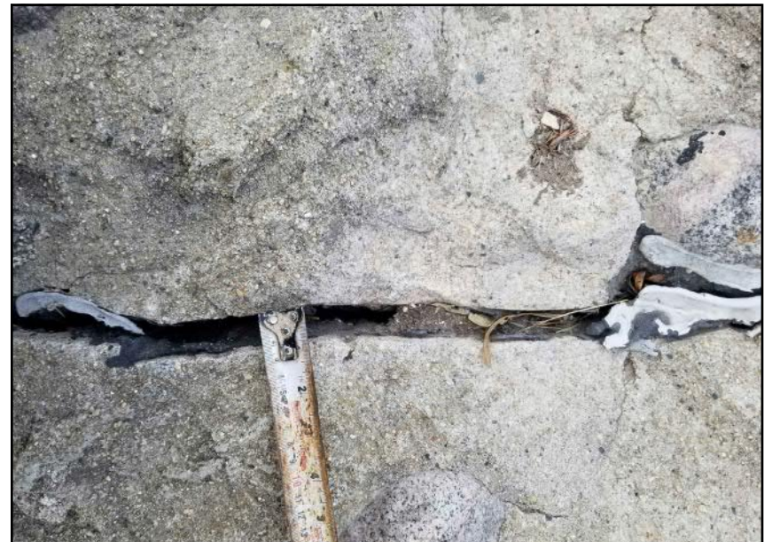
Site 7 - Western Bank Cracks observed within grouted rip-rap armorings at various orientations
