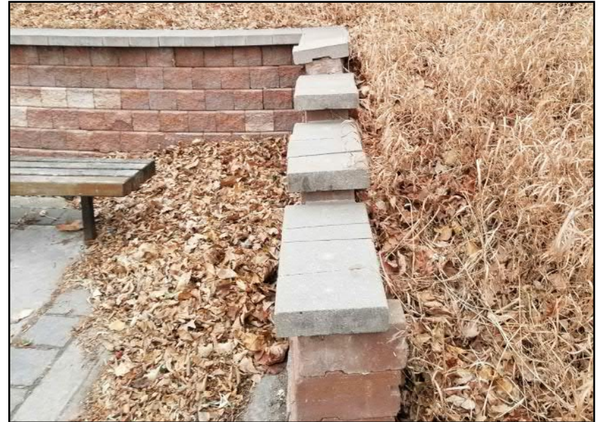
Site 10 - Northern Riverbank Masonry retaining wall structure near pedestrian pathway shows small signs of movement (facing W)
