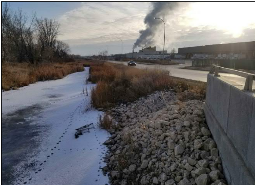
Site 8 - Western Bank Regraded and rip-rap armoured slope within crossing alignment (facing S)
