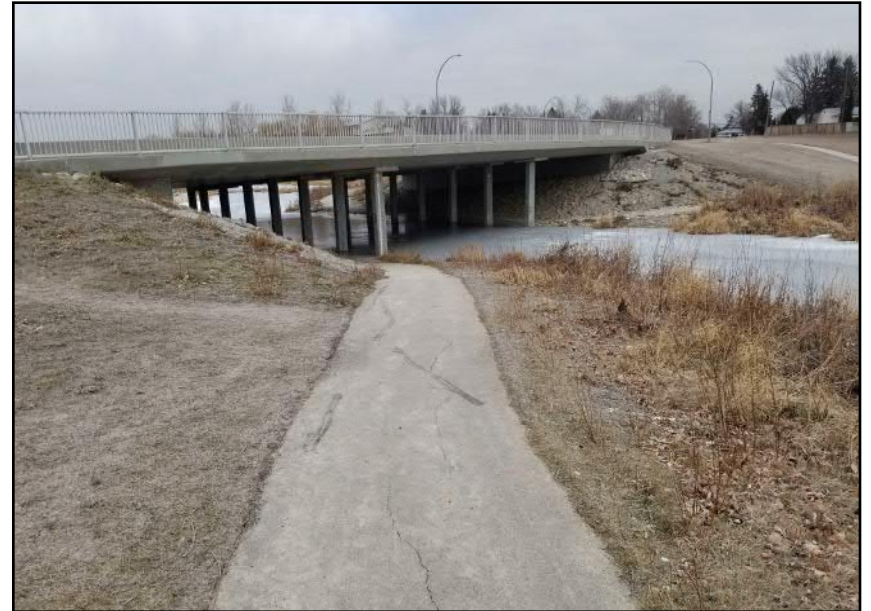
Site 7 - Western Bank Steeper slope around bridge abutment and minor cracking along pedestrian pathway (facing NE)
