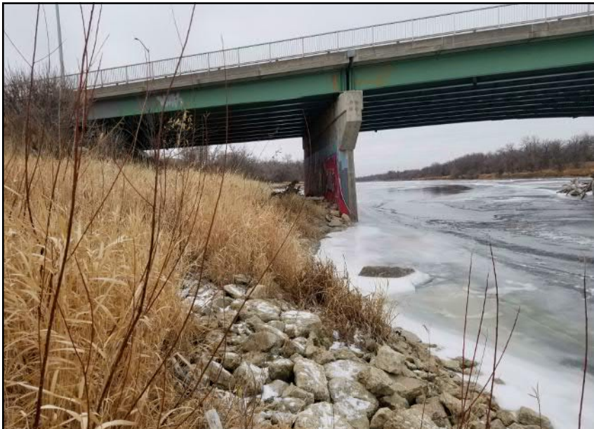
Site 5 - Southern Riverbank | Rip-rap armouring along bank slope between CSP culverts and river edge (facing W)
