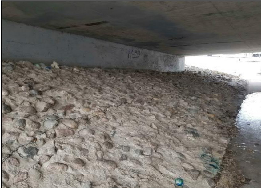
Site 7 - Western Bank Grouted rip-rap along abutment head slope below bridge structure (facing NW)
