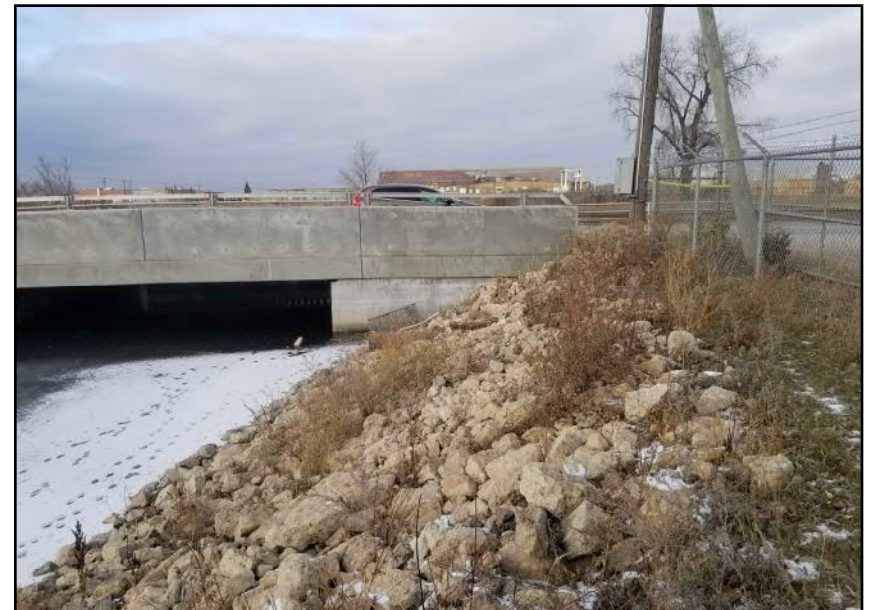
Site 8 - Eastern Bank Regraded and rip-rap armoured slope near bridge structure (facing N)
