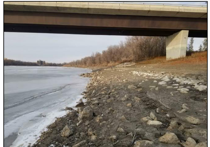
Site 4 - Eastern Riverbank | Rip-rap armouring along entire lower portion of riverbank between bridges (facing N)
