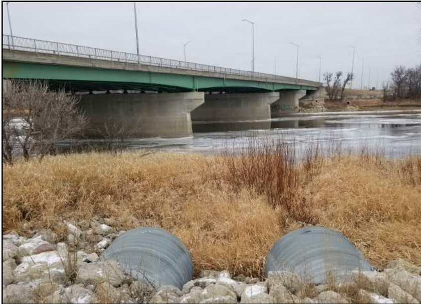
Site 5 - Southern Riverbank | Discharge path of CSP culverts west of crossing alignment, gradual bank slopes (facing NW)
