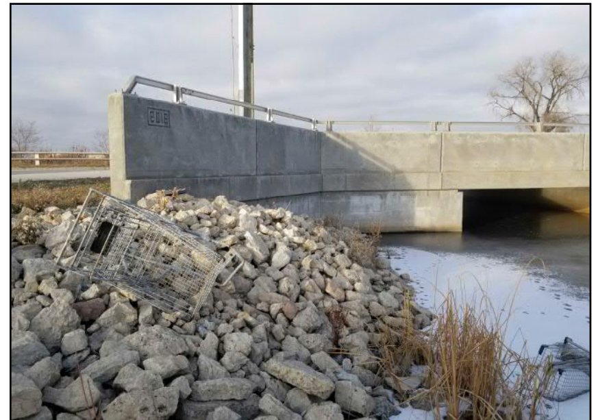
Site 8 - Western Bank Regraded and rip-rap armoured slope near bridge structure. Steeper slope near abutment (facing N)
