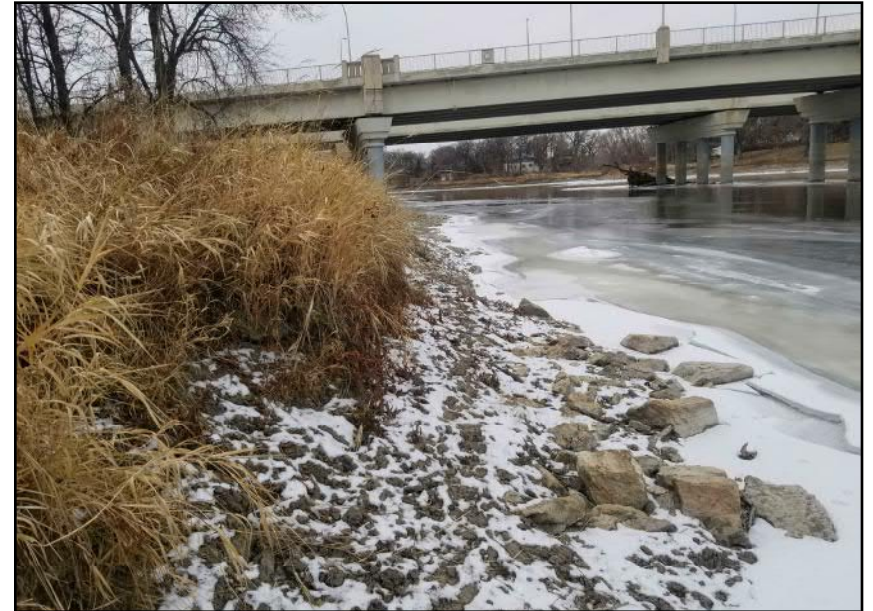
Site 10 - Southern Riverbank Local rip-rap observed along the bank toe near the crossing alignment (facing W)
