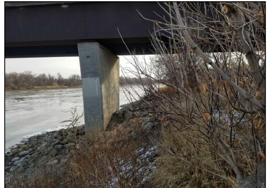
Site 4 - Western Riverbank South bridge pier near river edge surrounded in rip-rap armouring (facing S)
