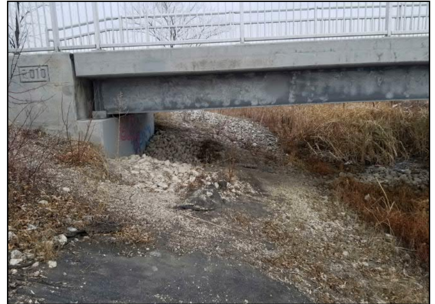
Site 9 - Western Bank Displaced rip-rap and exposed geotextile at bridge abutment north of the crossing (facing NW)
