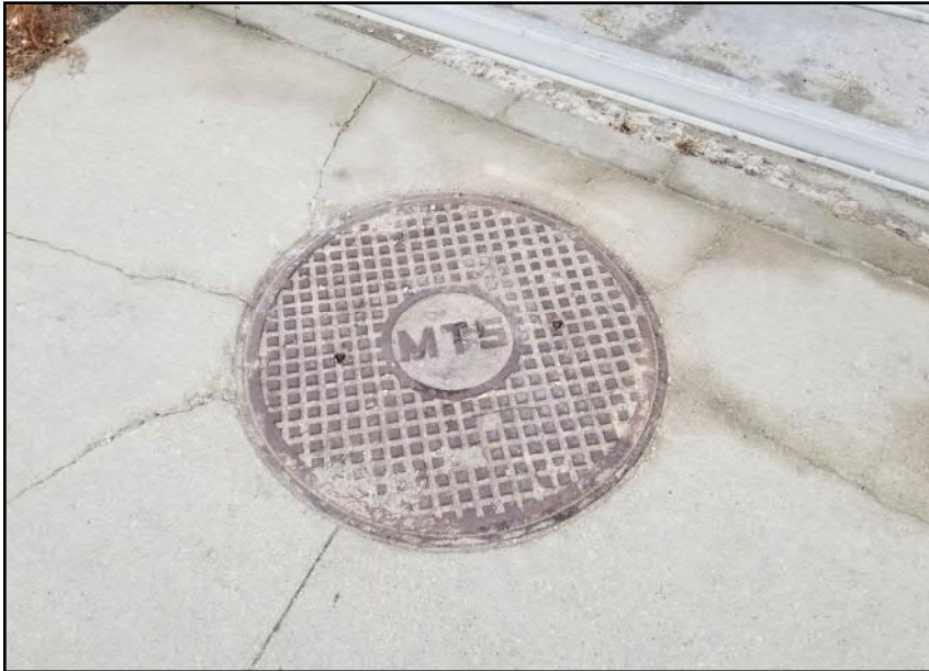
Site 7 - Western Bank Cracks around MTS manhole located in paved bridge sidewalk near abutment
