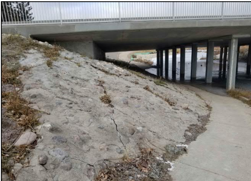
Site 7 - Western Bank Grouted rip-rap armouring along steeper banks in close proximity to bridge abutment (facing N)
