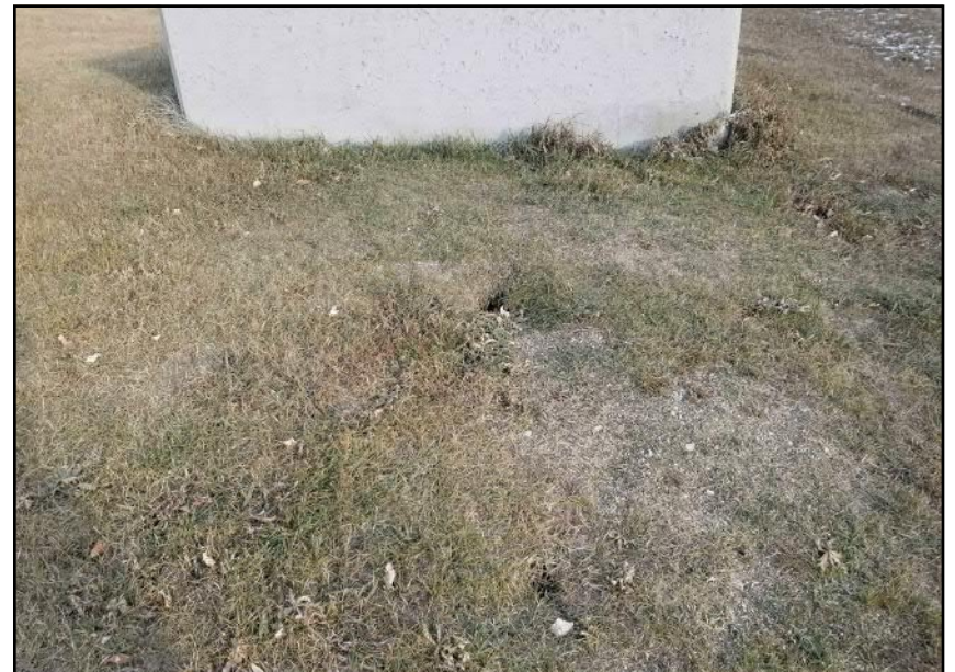
Site 4 - Eastern Riverbank Animal burrows observed in front of siphons inlet chamber structure (facing W)
