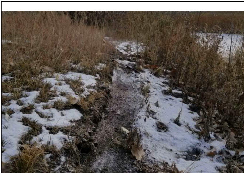
Site 8 - Eastern Bank Scarp ridge observed near bank crest at oversteepened bank south of rip-rap area (facing S)
