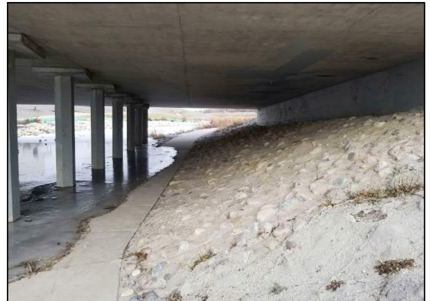
Site 7 - Eastern Bank Grouted rip-rap along abutment head slope below bridge structure (facing N)
