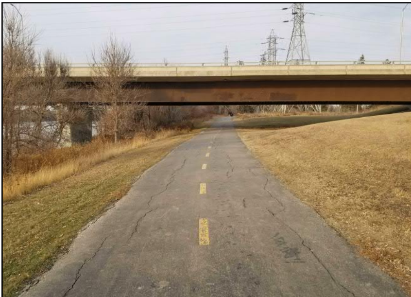
Site 4 - Eastern Riverbank Asphalt paved pedestrian pathway. Minor cracking observed parallel to bank crest (facing N)
