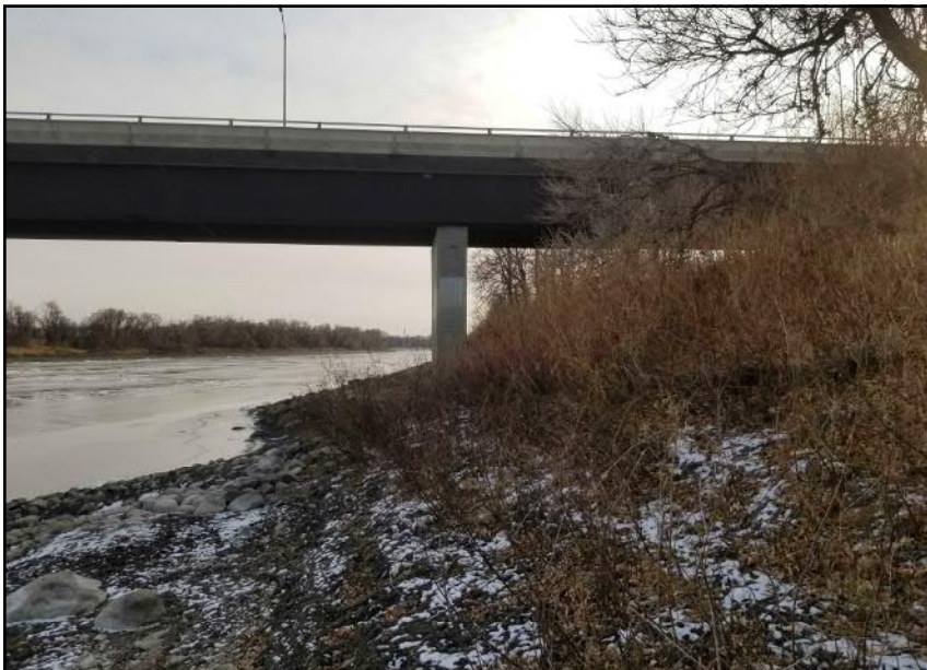
Site 4 - Western Riverbank Short erosion scarps, localized rip-rap, gradual toe slope adjacent to crossing alignment (facing S)
