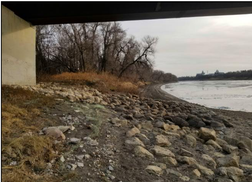
Site 4 - Eastern Riverbank Rip-rap armouring around south bridge pier and along gradually sloping bank toe (facing S)
