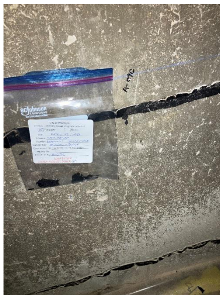
Photograph 9: Sample Group A-09 – Example of Black Mastic on Basement Tunnel Wall, Asbestos Not Detected
