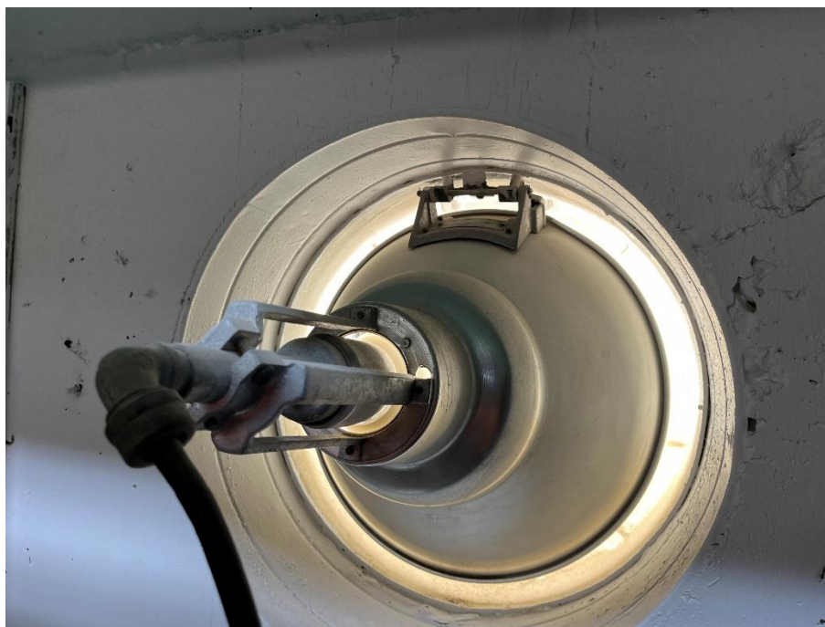
Photograph 15: Light Fixture in Pool with Suspect Mercury-Containing Bulb
