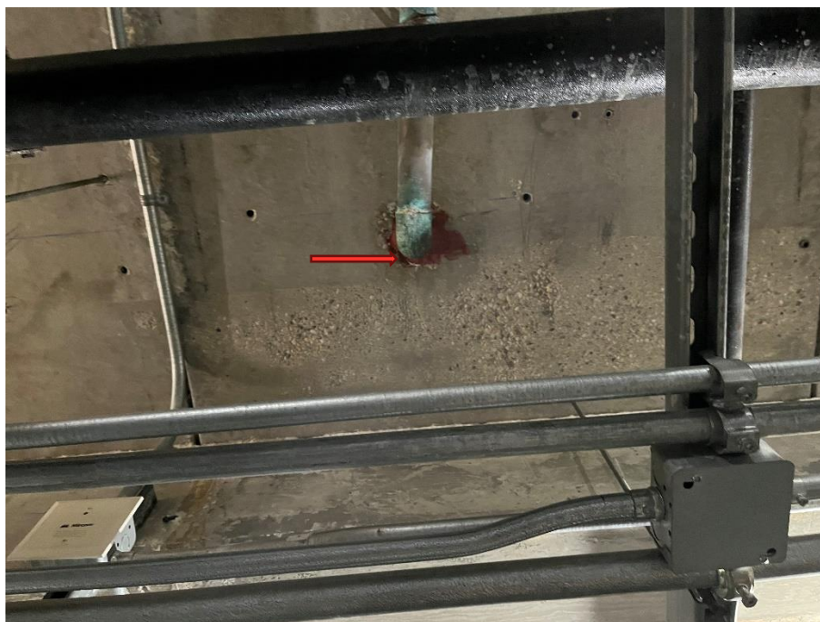
Photograph 10: Example of Red Fire Stopping at Pipe Penetrations, Presumed to Contain Asbestos
