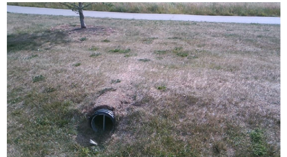
*Photo of Existing Culvert to Retention Pond
