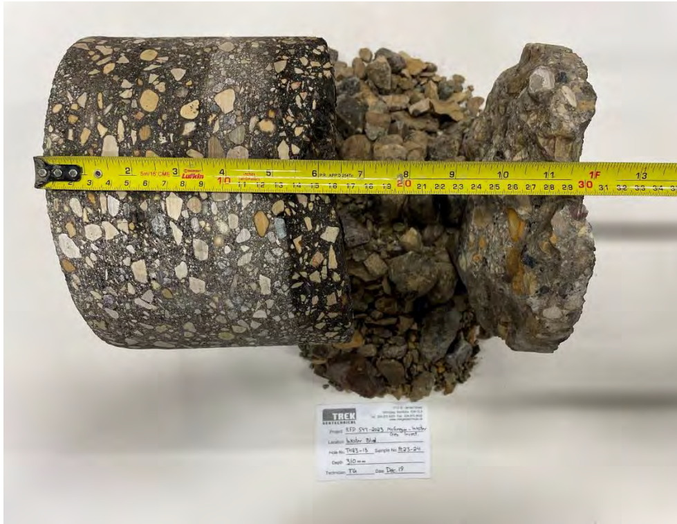
Photo 3: Pavement Core Sample at Test Hole TH23-13
