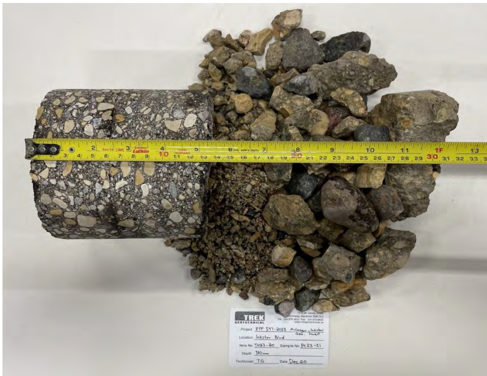
Photo 10: Pavement Core Sample at Test Hole TH23-20
