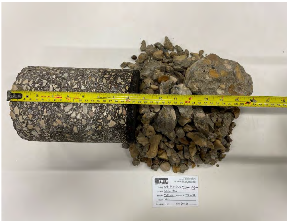
Photo 8: Pavement Core Sample at Test Hole TH23-18
