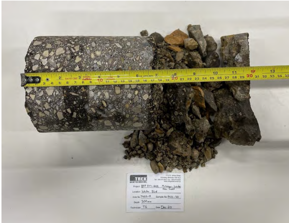
Photo 9: Pavement Core Sample at Test Hole TH23-19
