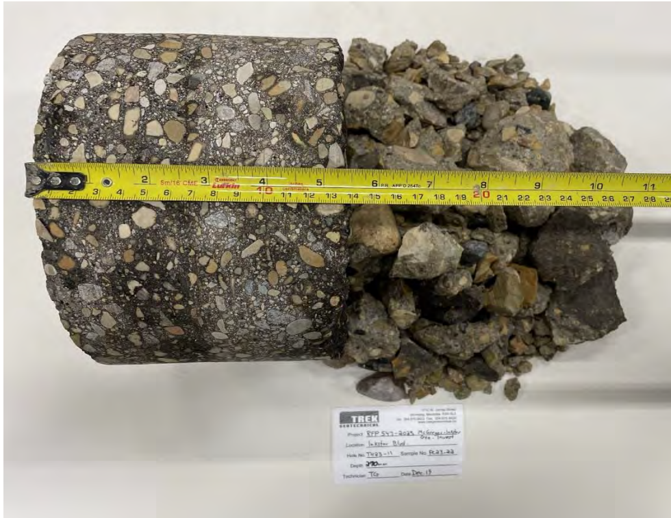
Photo 1: Pavement Core Sample at Test Hole TH23-11
