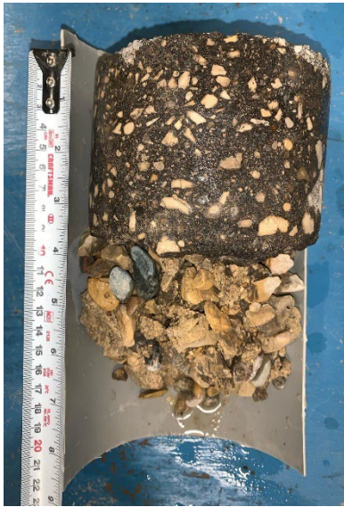
Figure 9 – Core No. 48 (Gordon Ave)
