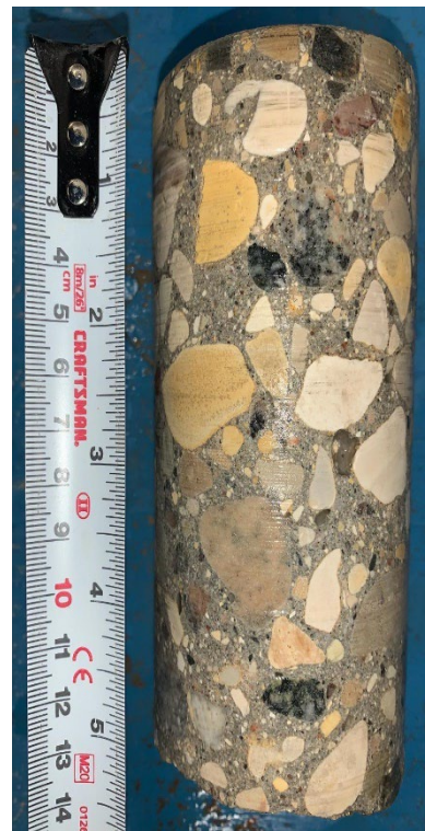
Figure 16 – Core No. 55 (Hood Ave)
