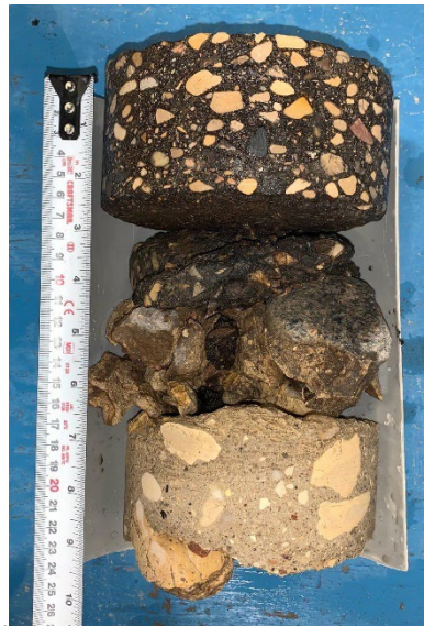
Figure 7 – Core No. 46 (Gordon Ave)
