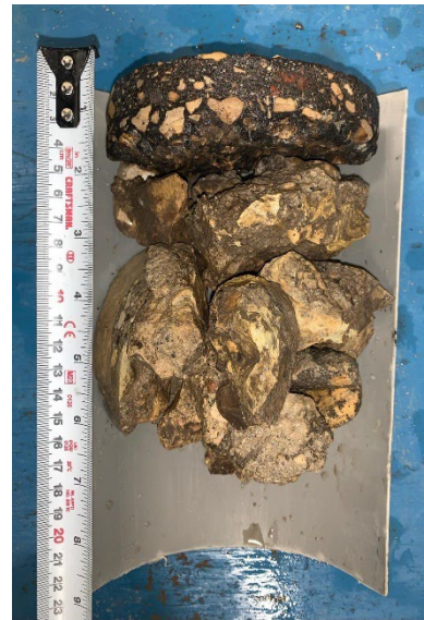
Figure 8 – Core No. 47 (Gordon Ave)
