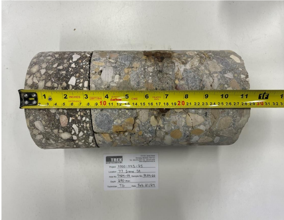
Photo 3: Pavement Core Sample at TH24-03
