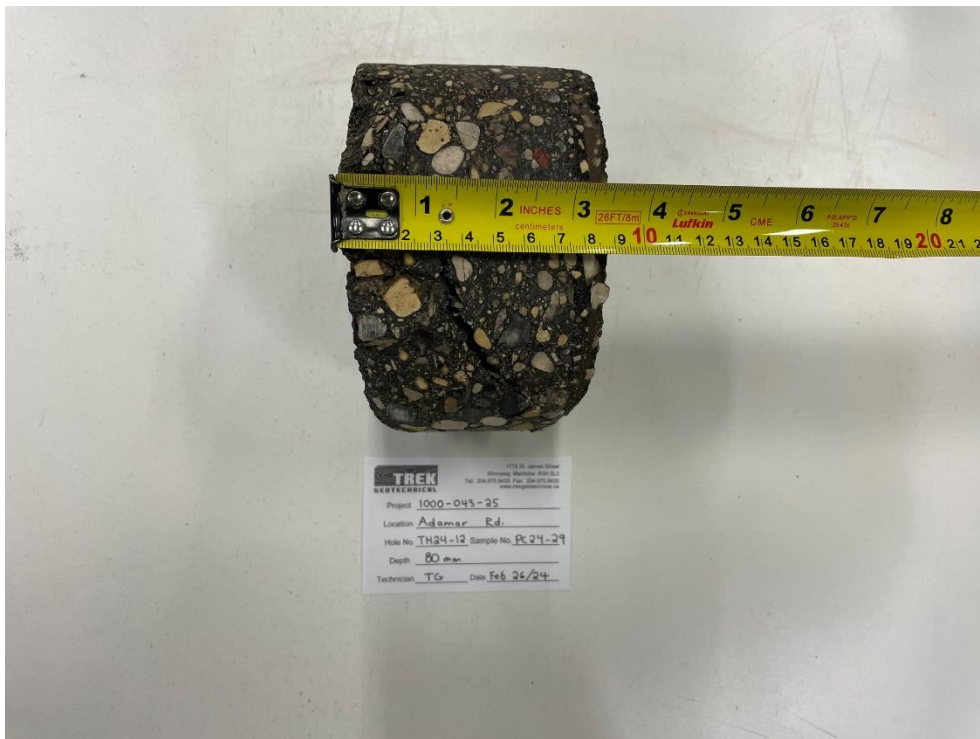
Photo 4: Pavement Core Sample at TH24-12
