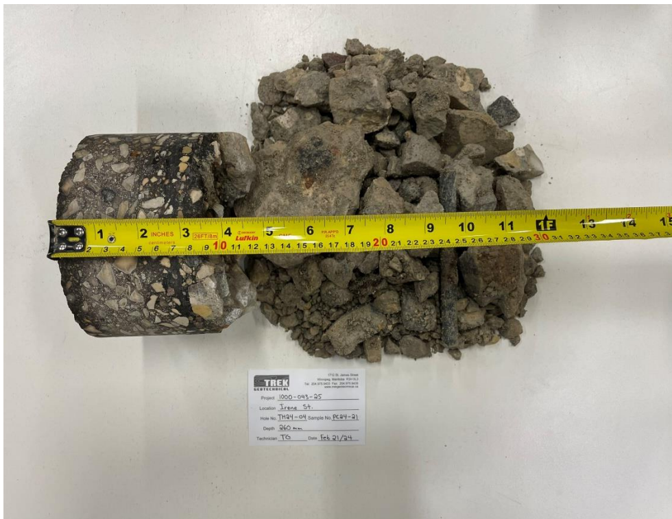
Photo 4: Pavement Core Sample at TH24-04
