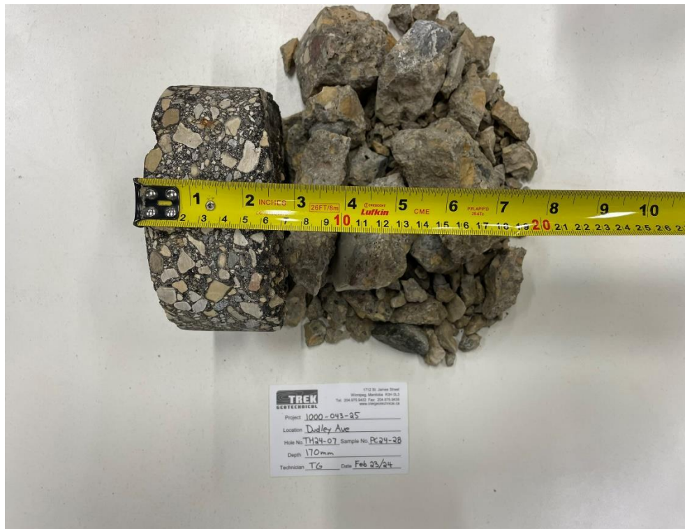
Photo 2: Pavement Core Sample at TH24-07
