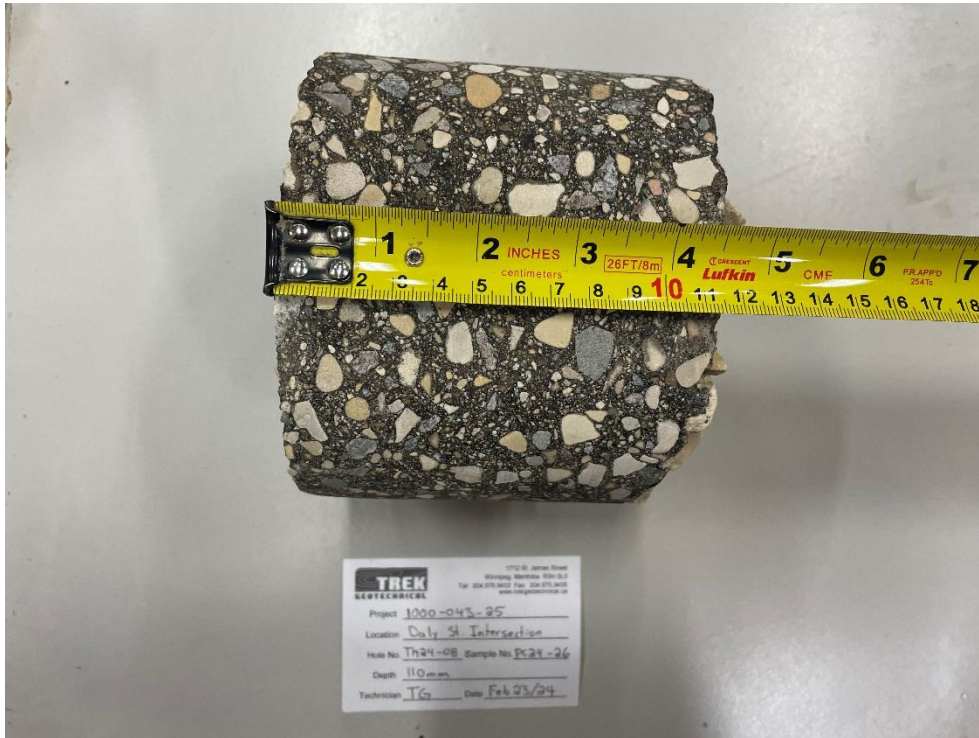
Photo 1: Pavement Core Sample at TH24-08
