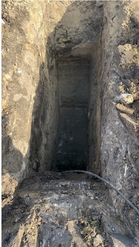
TP24-02 Photo 1: Top of bedrock encountered at 4.6 m
