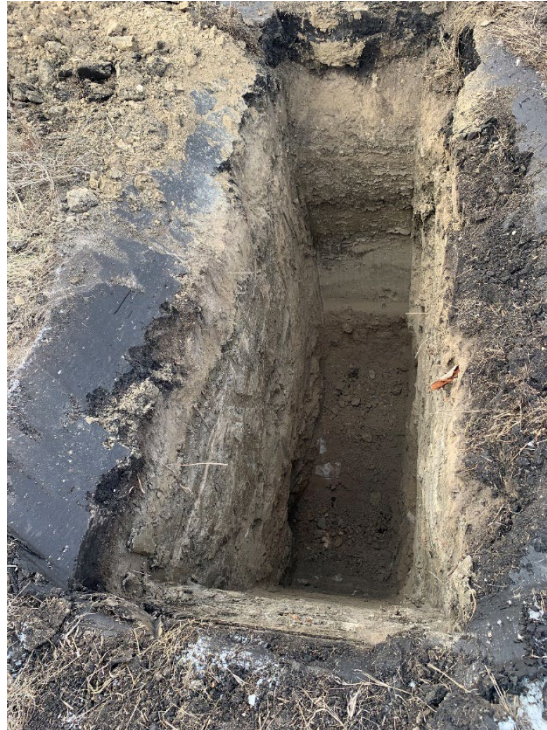
TP24-01 Photo 1: Completed test pit to 5.1 m
