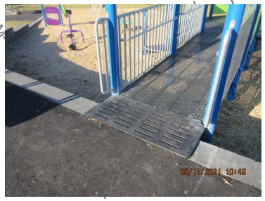
ACCESSIBLE ELEVATED PLATFORM ENTRY
