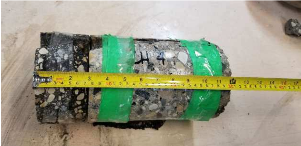
South bound transverse joint, Sta. 1+300
