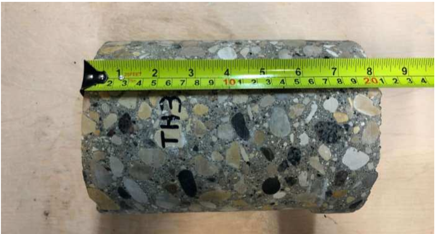
TH 3, south bound Sta. 0+756
