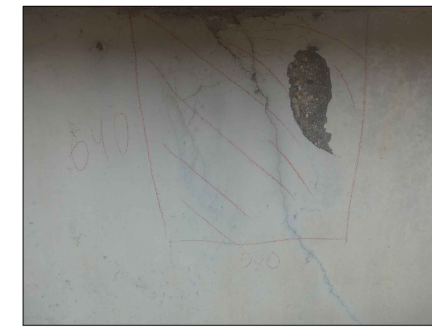
PHOTO 1 DELAMINATION
