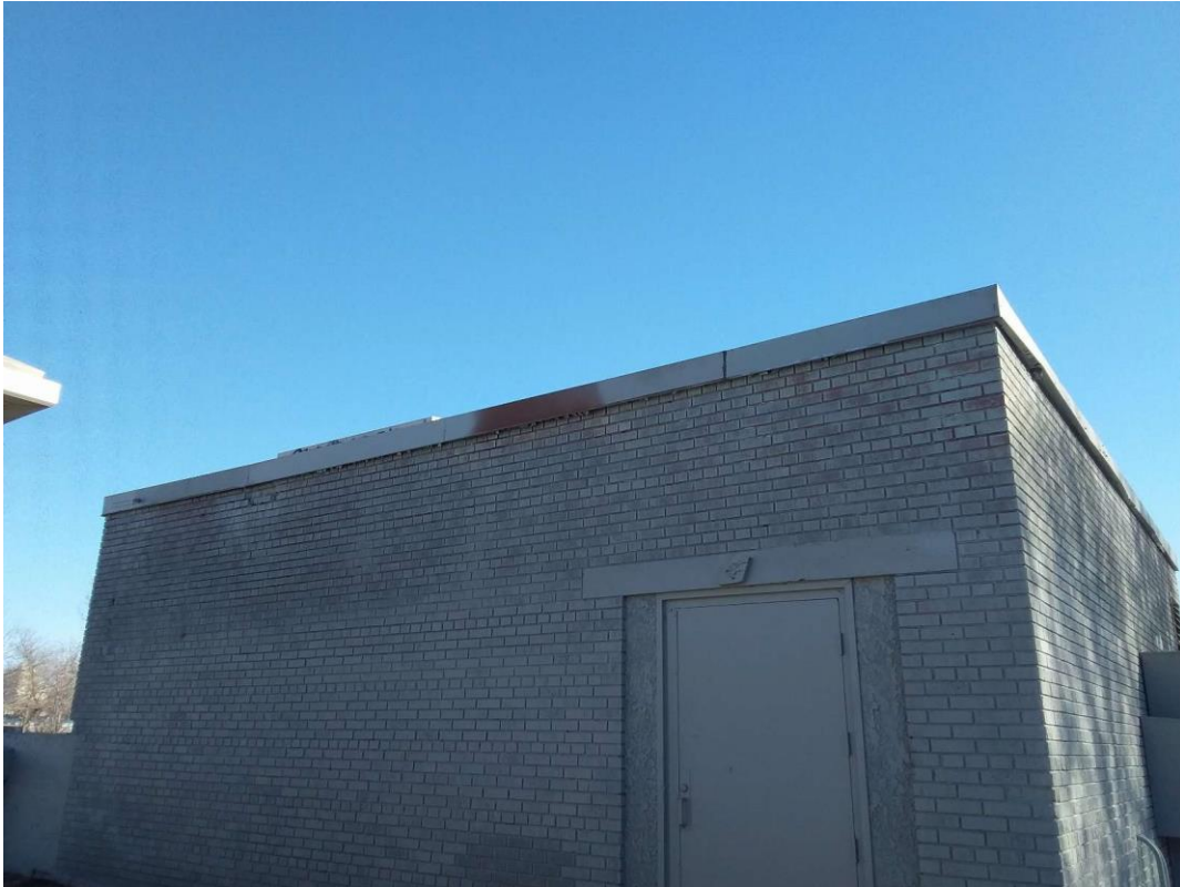
Pb Products, V9000(Yes), ROOF FLASHING, Painted grey, Exterior of Building (Location #: 3)
