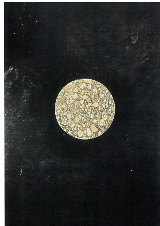
PC-20 Top of Asphalt Pavement Ø = 150 mm
