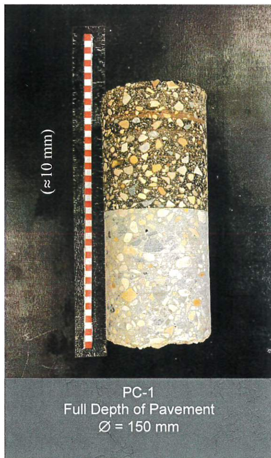
Photograph 1: Specimen from Ellice Avenue, Eastbound Curb Lane
