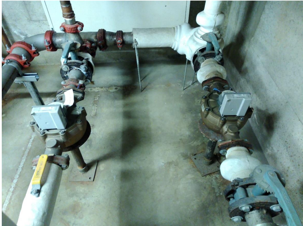
Figure 9: Separate meters for the library and parkade.
