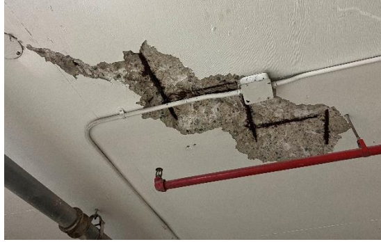
Figure 6: Exposed reinforcement
