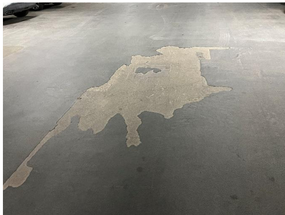
Figure 3: Traffic membrane repair on P1
