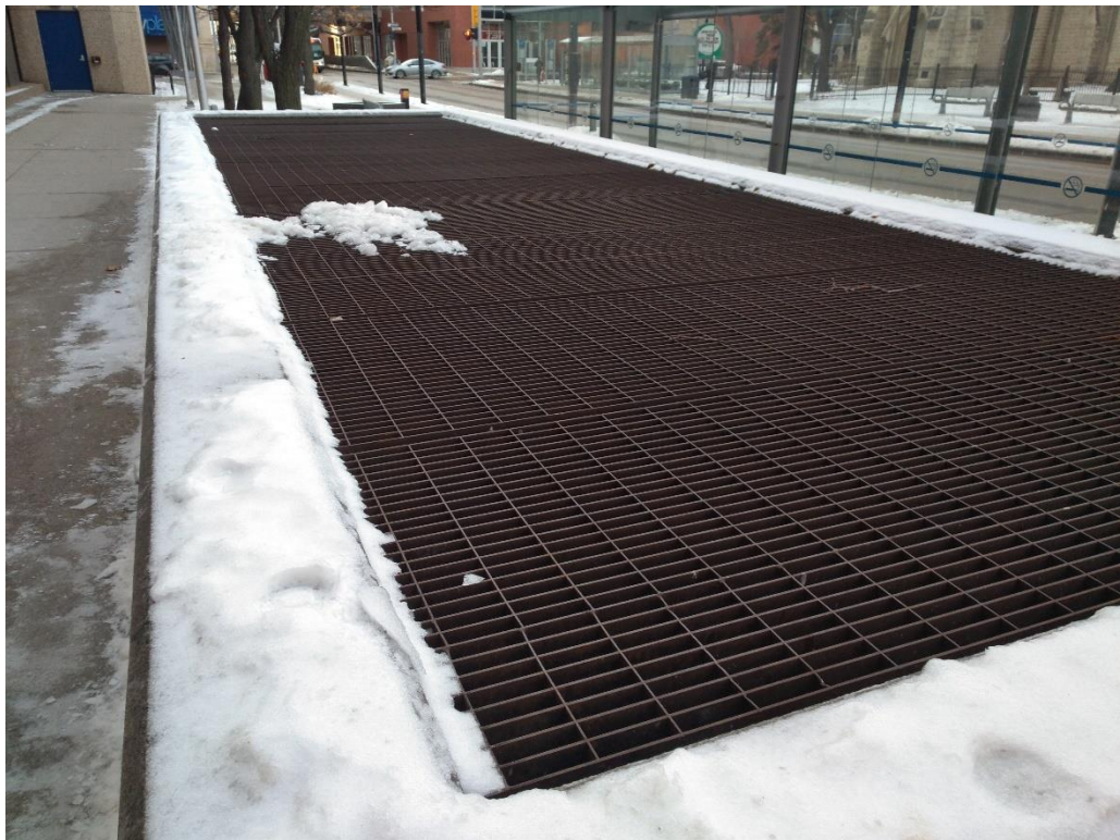
Figure 26: Intake louver for parkade make-up air unit.
