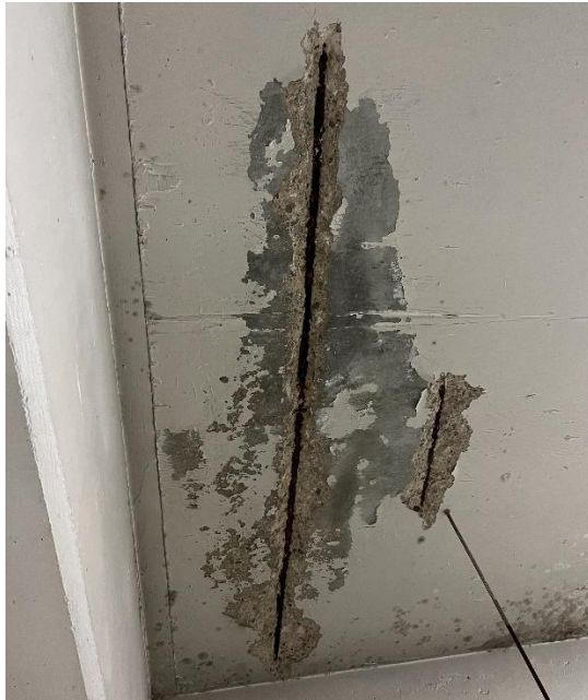
Figure 4: Exposed reinforcement
