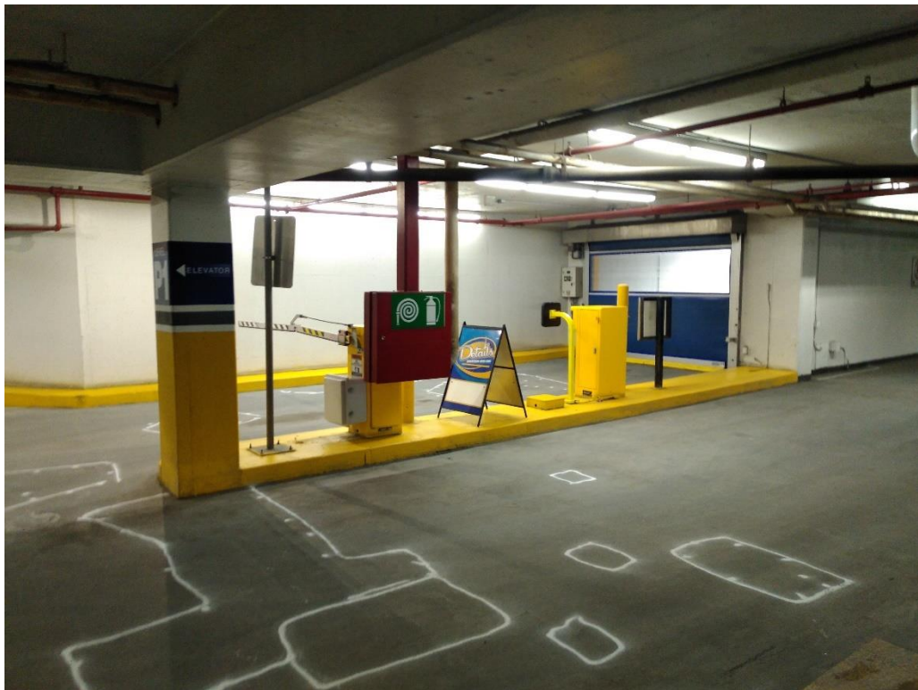
Figure 14: Hose cabinet and fire extinguisher installed as part of renovation project for Library
