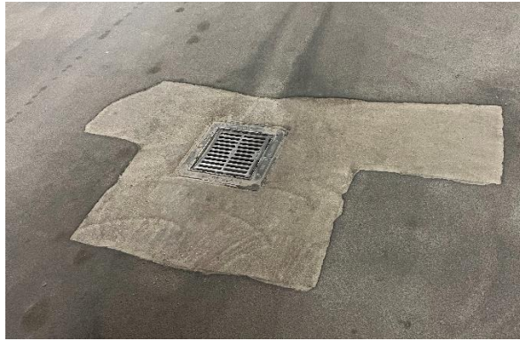
Figure 1: Traffic membrane repair on P1
