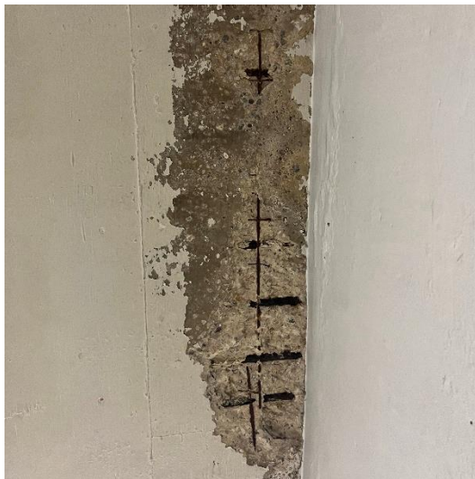
Figure 5: Exposed reinforcement
