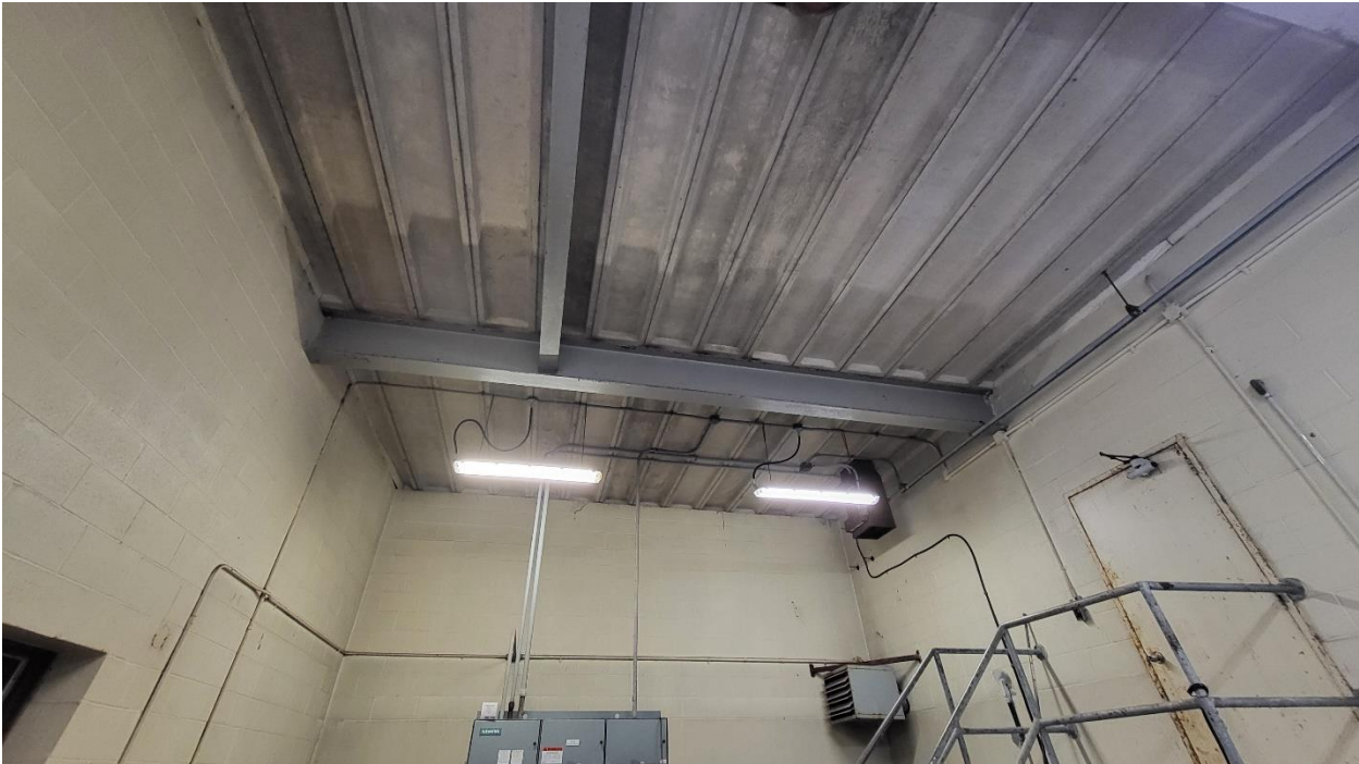
Photograph #9: Valve House Ceiling
