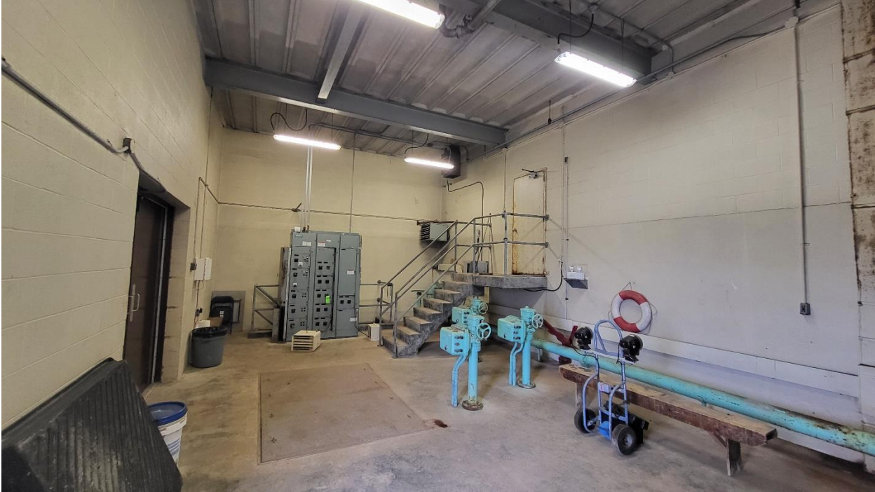
Photograph #15: Valve House
