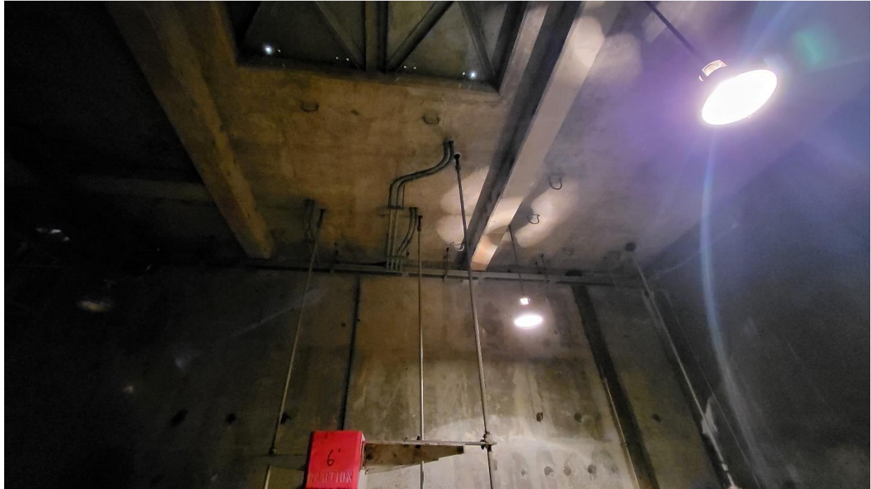
Photograph #10: Valve House Pit
