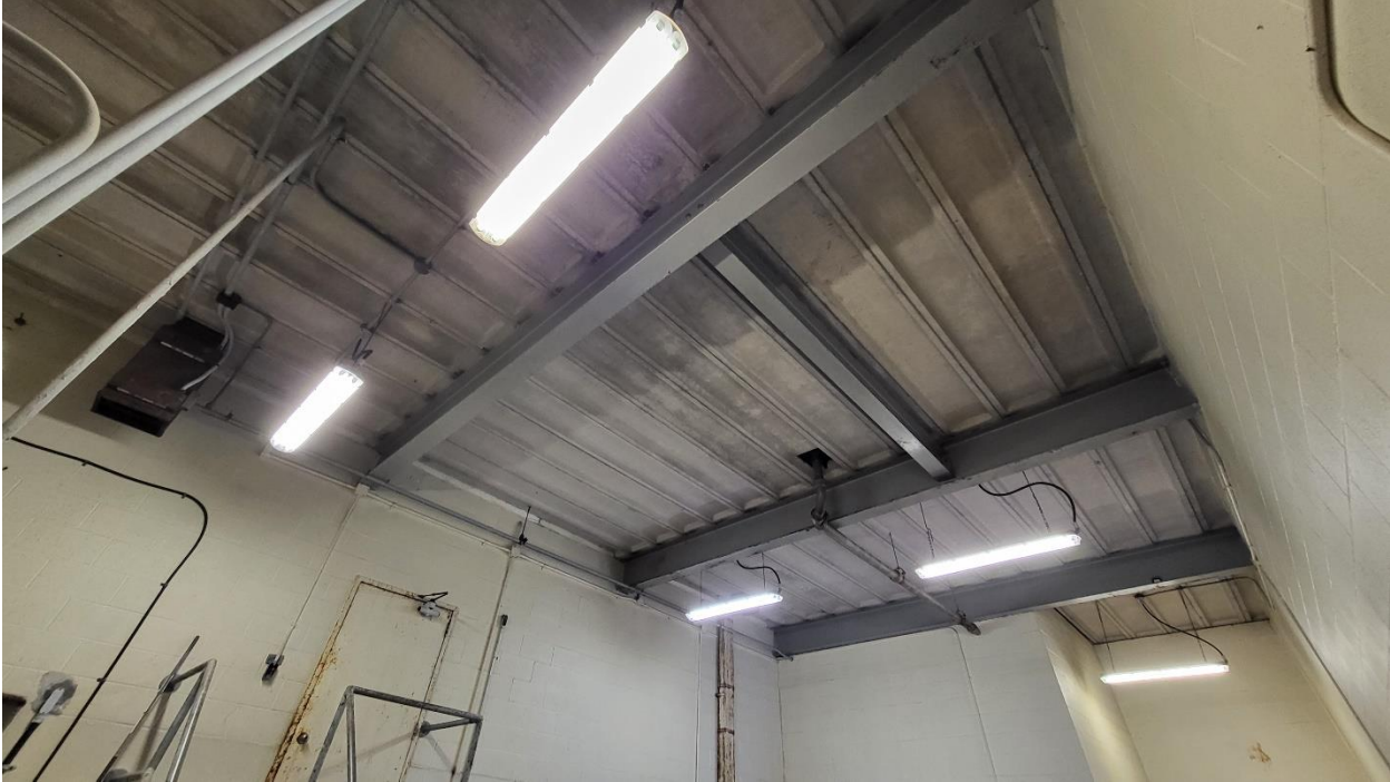
Photograph #8: Valve House Ceiling
