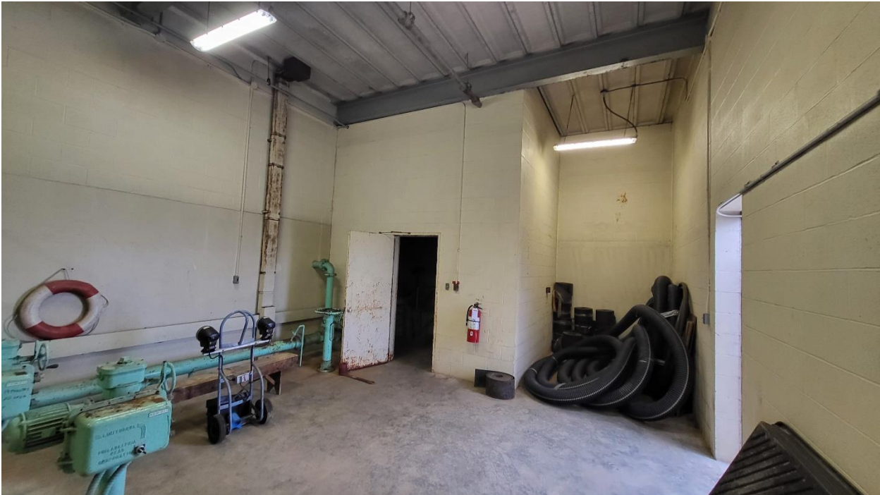
Photograph #16: Valve House
