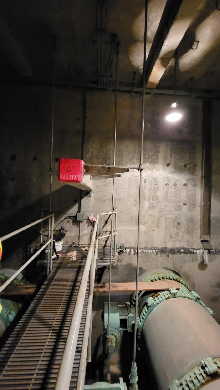
Photograph #12: Valve House Pit
