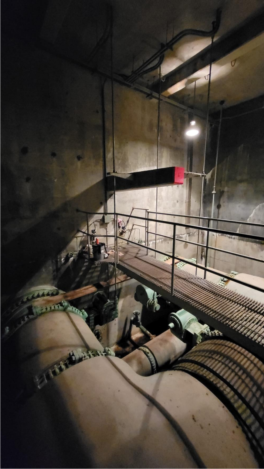
Photograph #13: Valve House Pit
