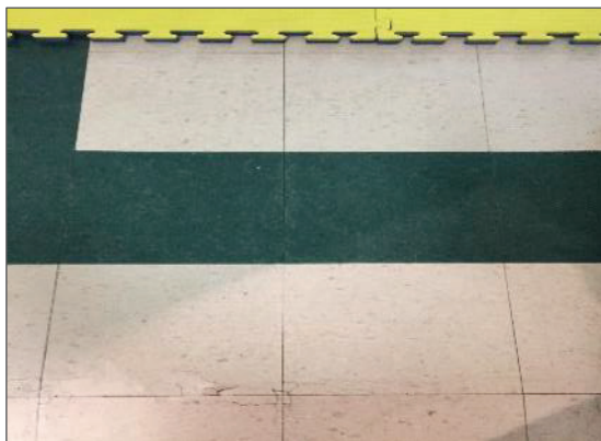
Photograph No.10: Non-asbestos vinyl floor tiles in the basement yoga room Loc. 9 (Samples 0012A-C).
