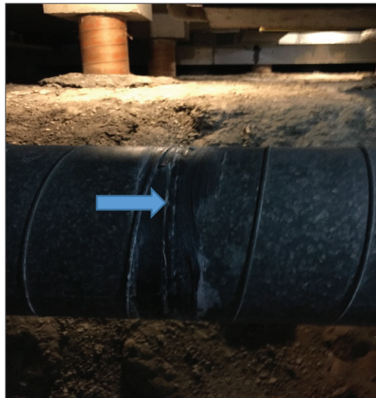
Photograph No. 23: Non-asbestos black/grey mastic present on uninsulated ducting within the south crawlspace and basement (Samples 0005A-C).
