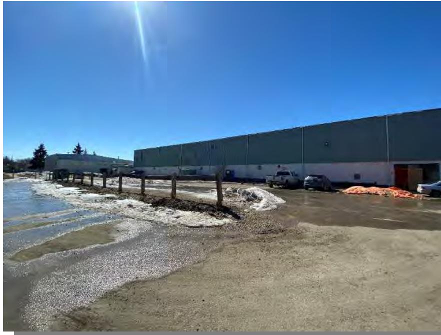
Photograph 11 – Exterior, east site boundary Looking southwest from the northeast elevation.
