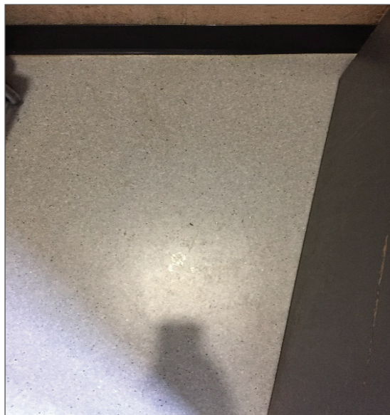
Photograph No. 9: Non-asbestos vinyl sheet flooring within the utility room Loc.53 (Rubber).
