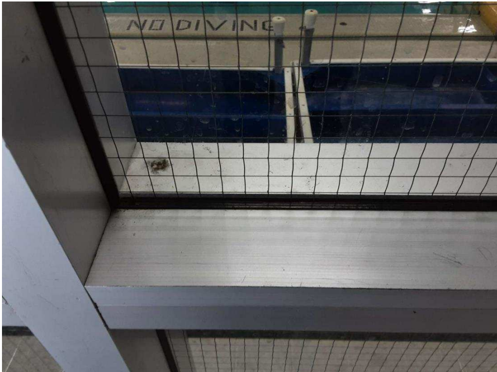
S0008C (None), Other, Window, Butyl Tape, Foyer (Location #: 15)
