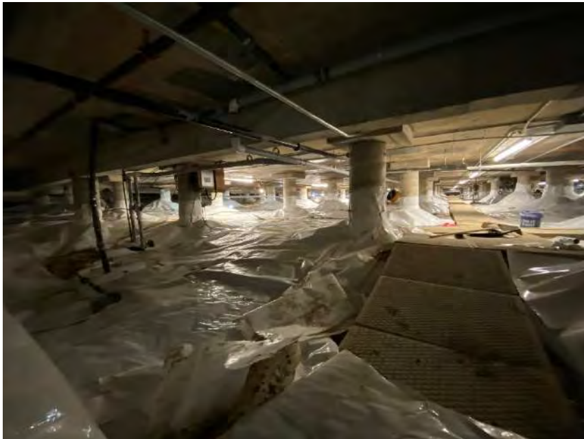
Photograph 32 – Interior, Arena crawlspace
