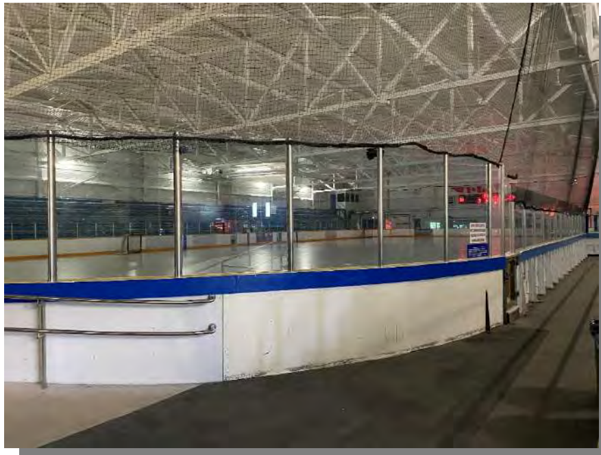
Photograph 14 – Interior, Arena Looking northwest at the Arena rink from the southeast corner.
