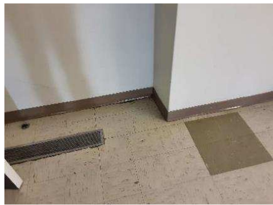
S0001B (None), Wall, Base, Adhesive/mastic, Auditorium (Location #: 1)
