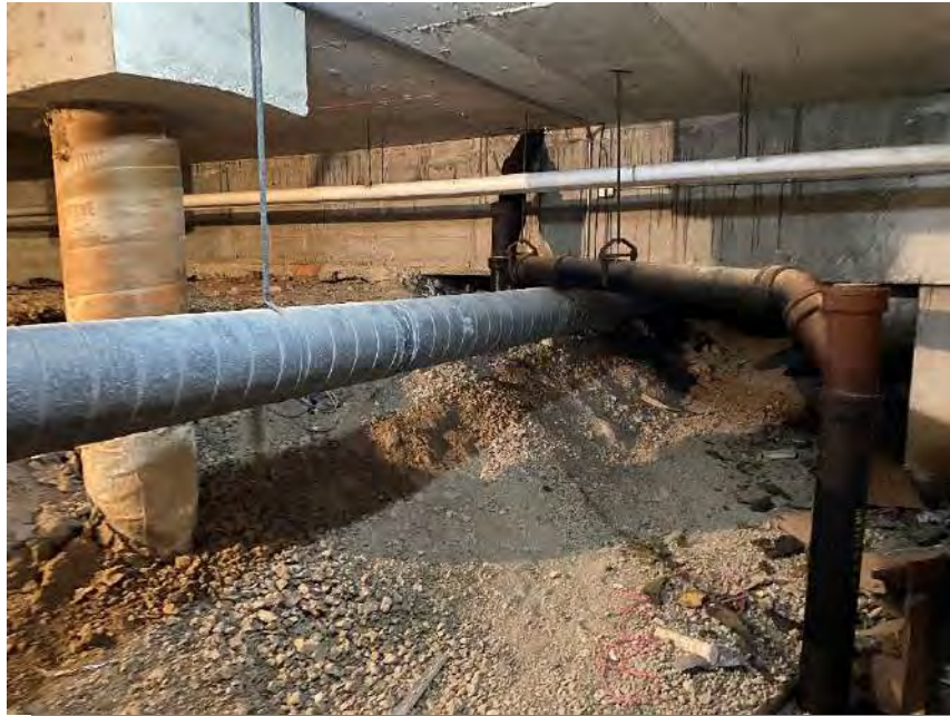
Photograph 33 – Interior, pool crawlspace
