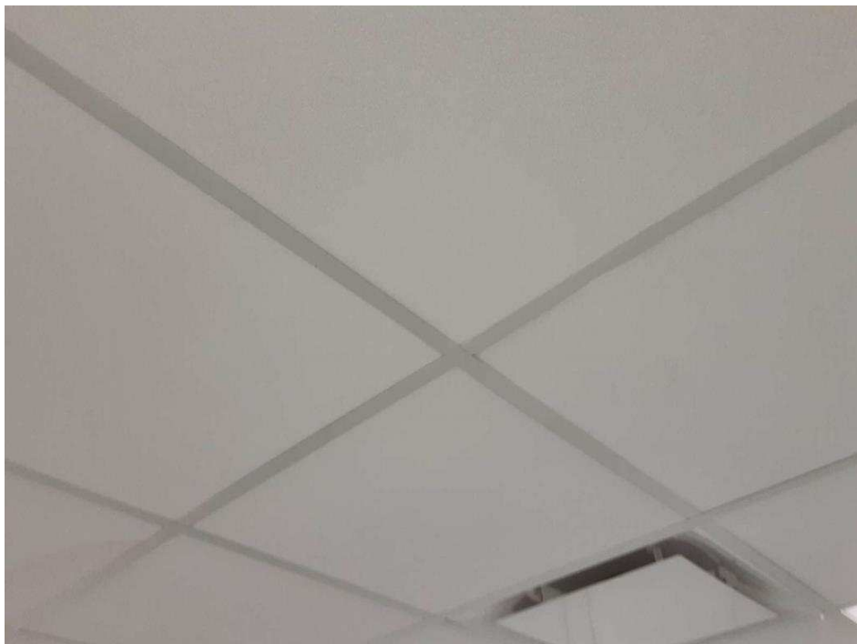
V0000 (None), Ceiling, Ceiling Tiles (lay-in), Classroom (Location #: 14)
