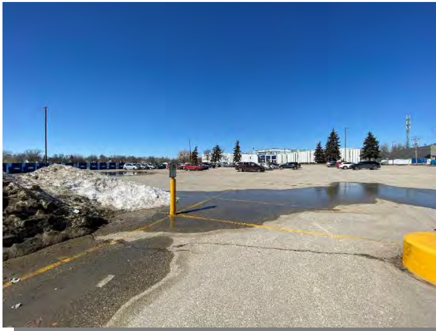
Photograph 10 – Exterior, south site boundary Looking north from the south elevation.
