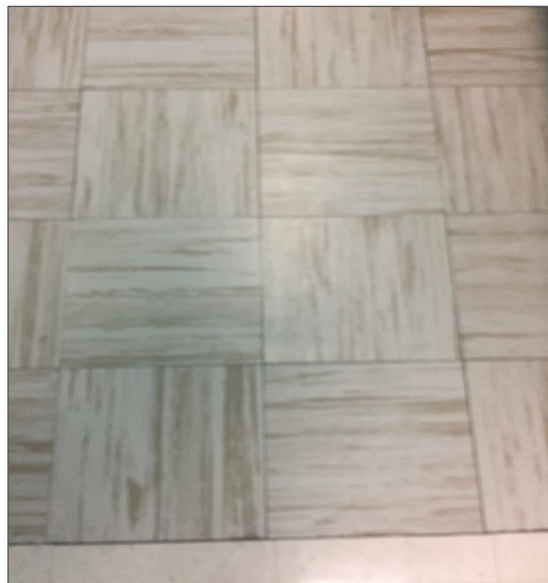
Photograph No. 13: Asbestos-containing vinyl floor tiles within pool corridor and office Loc.'s 38 and 43 (Samples 0033A-C).
