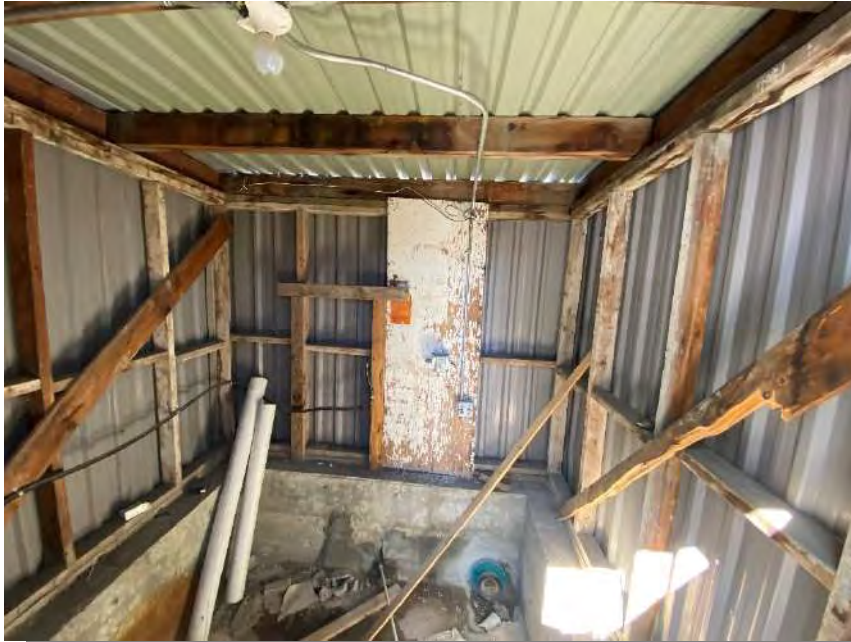
Photograph 31 – Exterior, out-building interior
