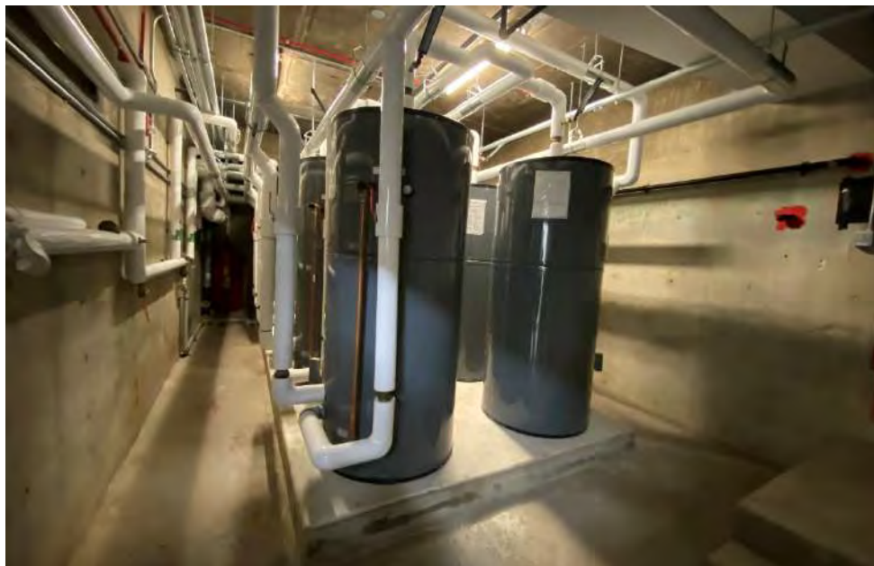
Photograph 24 – Interior, basement boiler room
