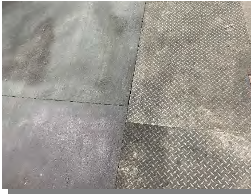
Photograph 34 – Interior, Arena flooring
