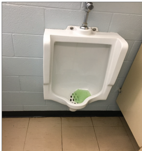
Photograph No. 19: Non-asbestos vinyl floor tiles within the mezzanine washrooms and offices (Samples 0050A-CA-C).
