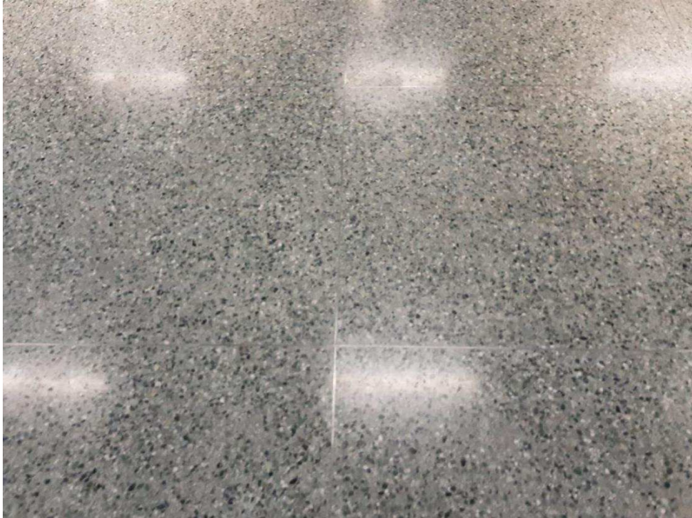
V9500 (Presumed Asbestos), Floor, Terrazzo, Foyer (Location #: 15)
