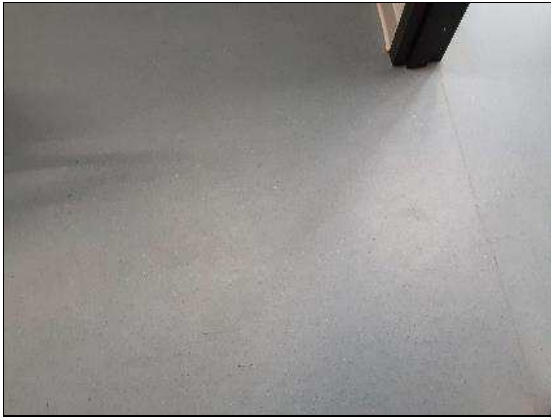
V0000 (None), Floor, Vinyl Sheet Flooring, Stairway To Stage (Location #: 5)
