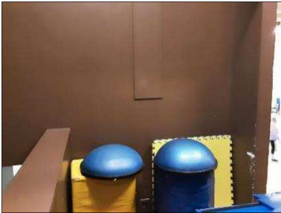
S0002A (None), Wall, Plaster, Stage (Location #: 2)
