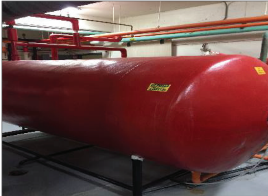
Photograph No. 3: Asbestos-containing parging cement present as insulation on the hot water holding tanks within the pool room Loc.13.
