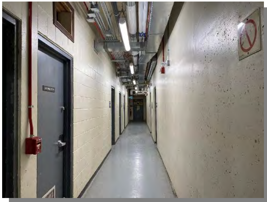
Photograph 22 – Interior, basement Looking east down the basement corridor that is underneath the center portion of the building.
