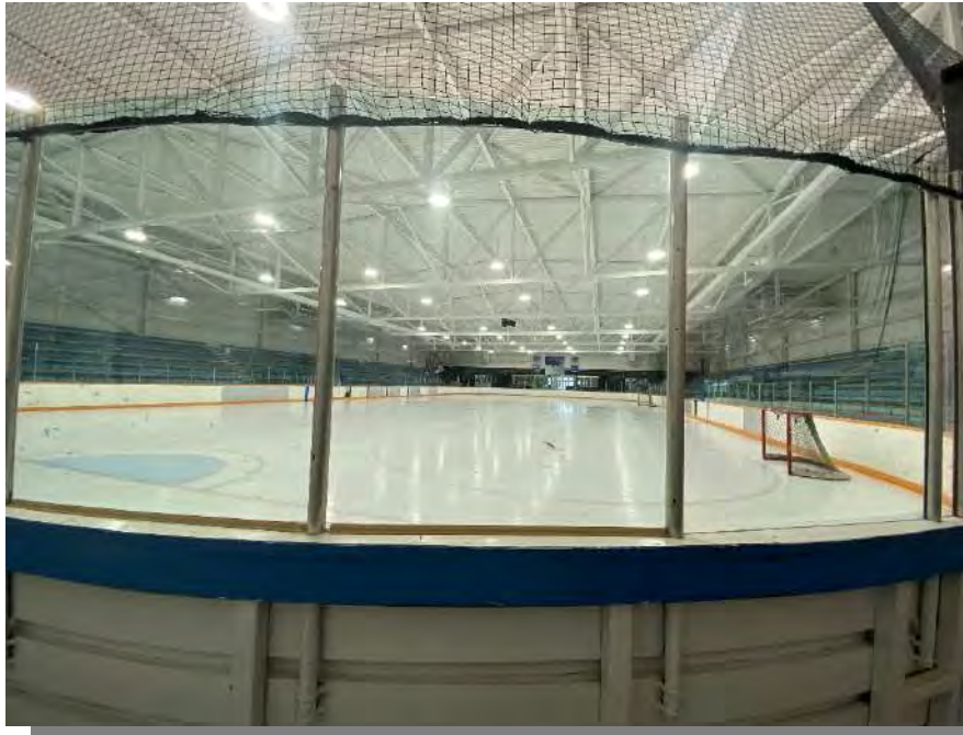
Photograph 15 – Interior, Arena Looking south at the Arena rink from the north side.
