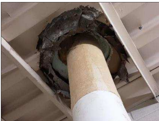
S0003C (None), Other, Tar Paper, Storage Room (Location #: 3)
