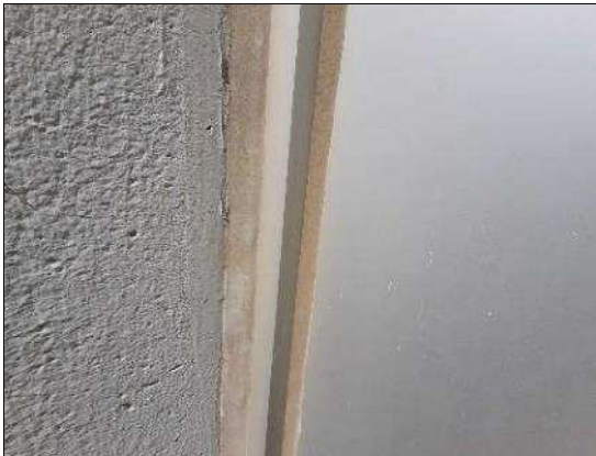
P0001 (PCB), Wall, Grey Caulking, Exterior Of Building (Location #: 19)
