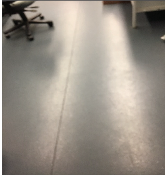
Photograph No. 8: Non-asbestos vinyl sheet flooring within the pool entrance Loc.39 (Rubber).
