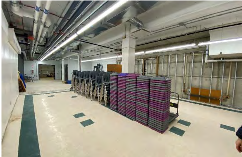
Photograph 23 – Interior, basement storage room
