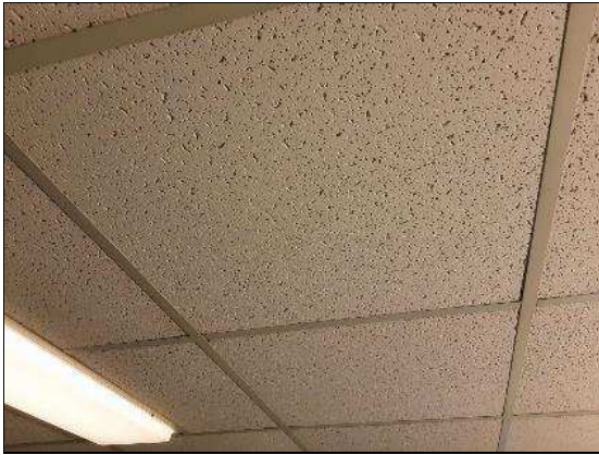
V0000 (None), Ceiling, Ceiling Tiles (lay-in), Men's Washroom (Location #: 10)
