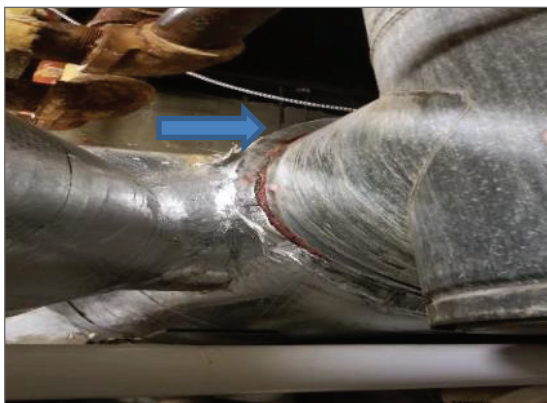
Photograph No. 21: Non-asbestos red/brown mastic on uninsulated ducting within the basement (Samples 0003A-C).
