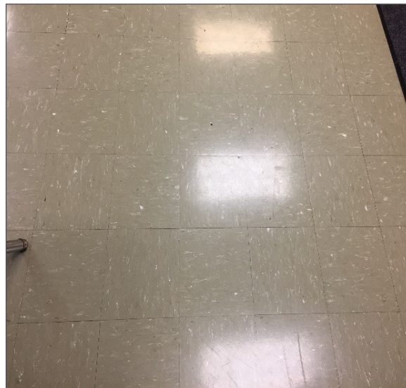
Photograph No. 15: Asbestos-containing vinyl floor tiles within the cloak room Loc.47 (Samples 0038A-C).
