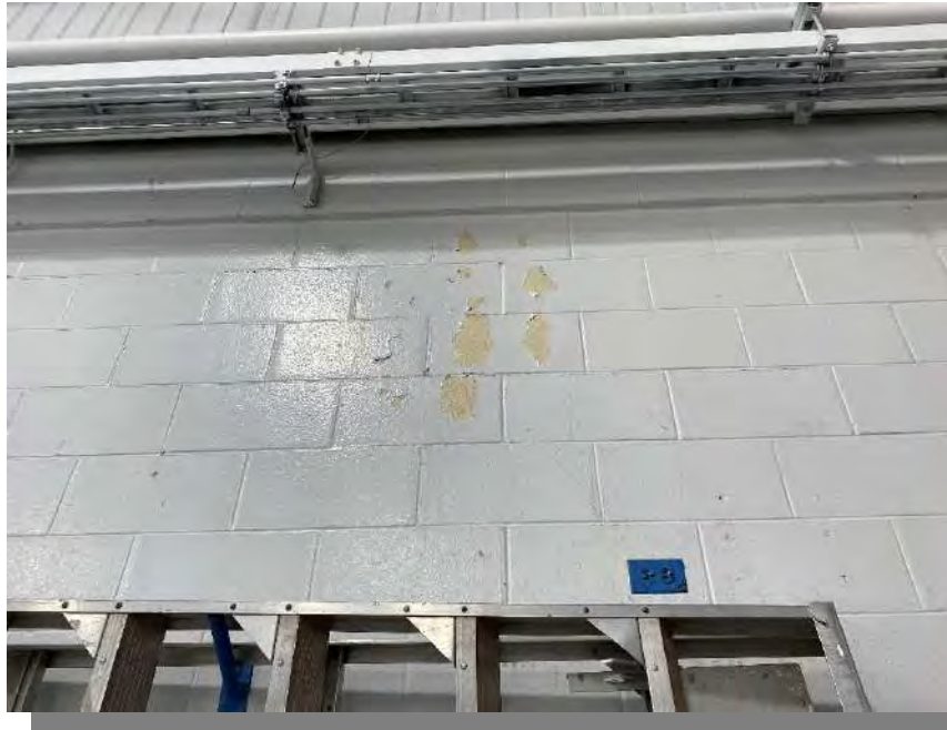
Photograph 35 – Interior, Arena north wall
