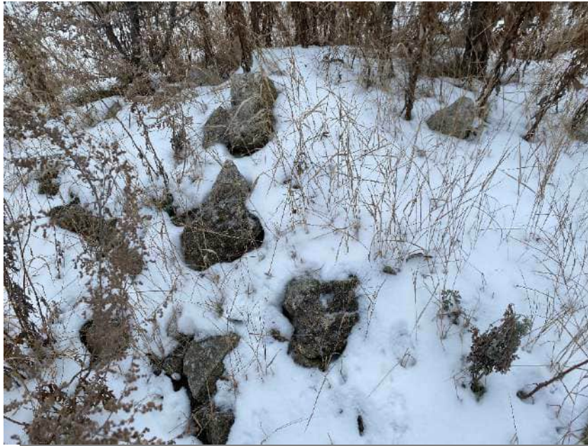
Photograph 19 – View of one of the small stockpiles present within the Study Area Looking at concrete rubble found in the small stockpiles, south of the POI.
