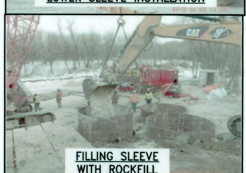
LOWER SLEEVE INSTALLATION
