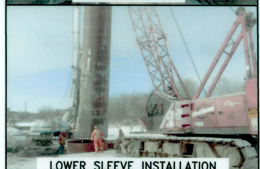
LOWER SLEEVE INSTALLATION
