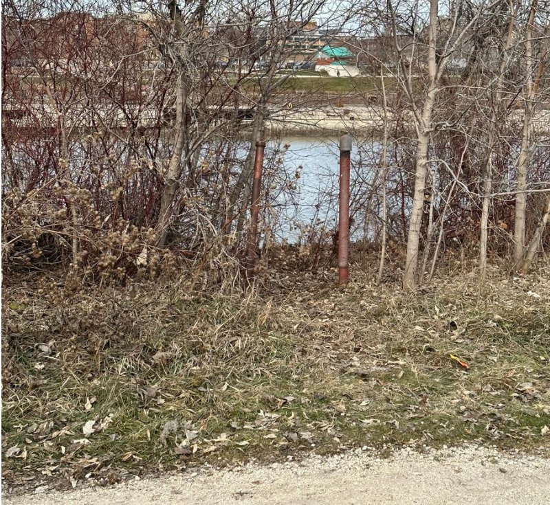
Figure 6 - Avenue Tache Underdrain Outfall – Vent Pipes, looking north.
