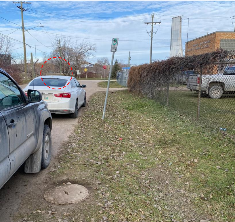
Figure 4 -Avenue Tache UMH110-0001, looking north.
