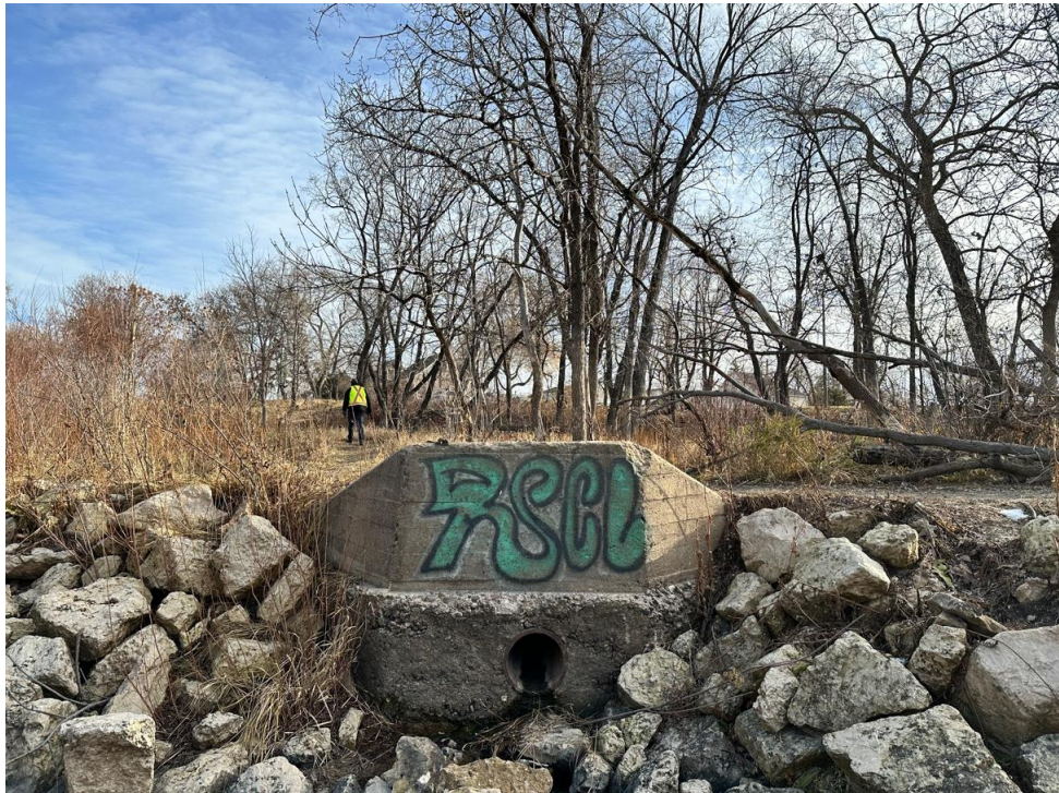
Figure 7 – Rue Notre Dame Underdrain Outfall, looking east.
