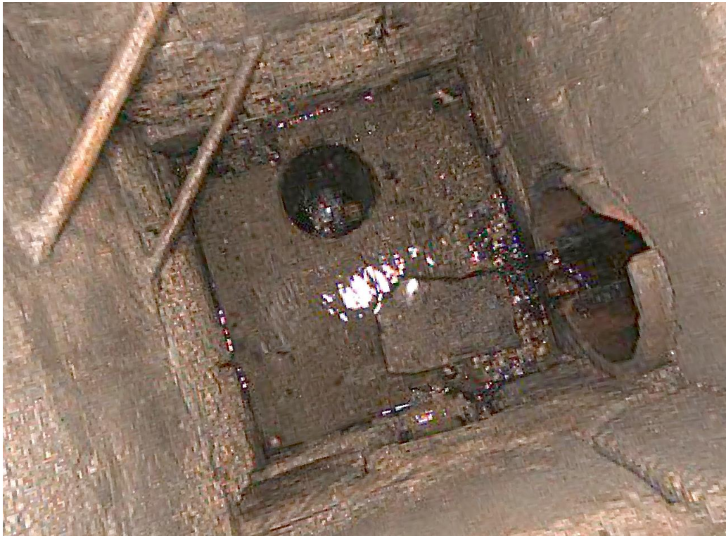
Figure 13 – UMH119-0137 (Dawson Rd) existing connections and floor drain.
