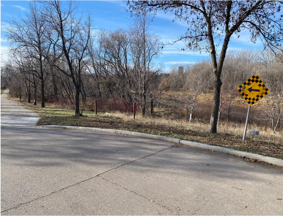
Figure 11 – Rue Notre Dame Underdrain Outfall Site, looking west.
