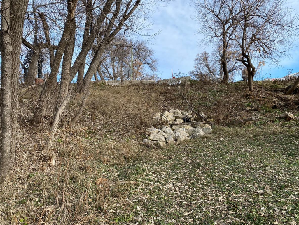
Figure 3 – Rue Plinguet Combined Sewer Outfall, looking east.
