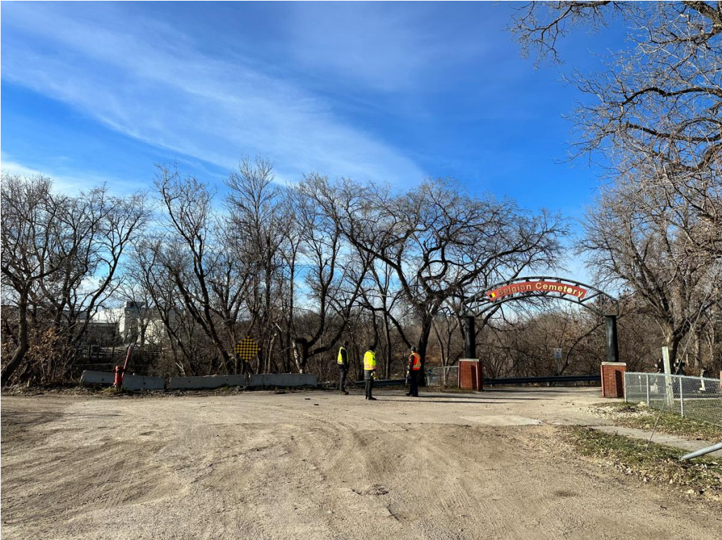
Figure 1 – Rue Plinguet Underdrain Outfall Site, looking west.
