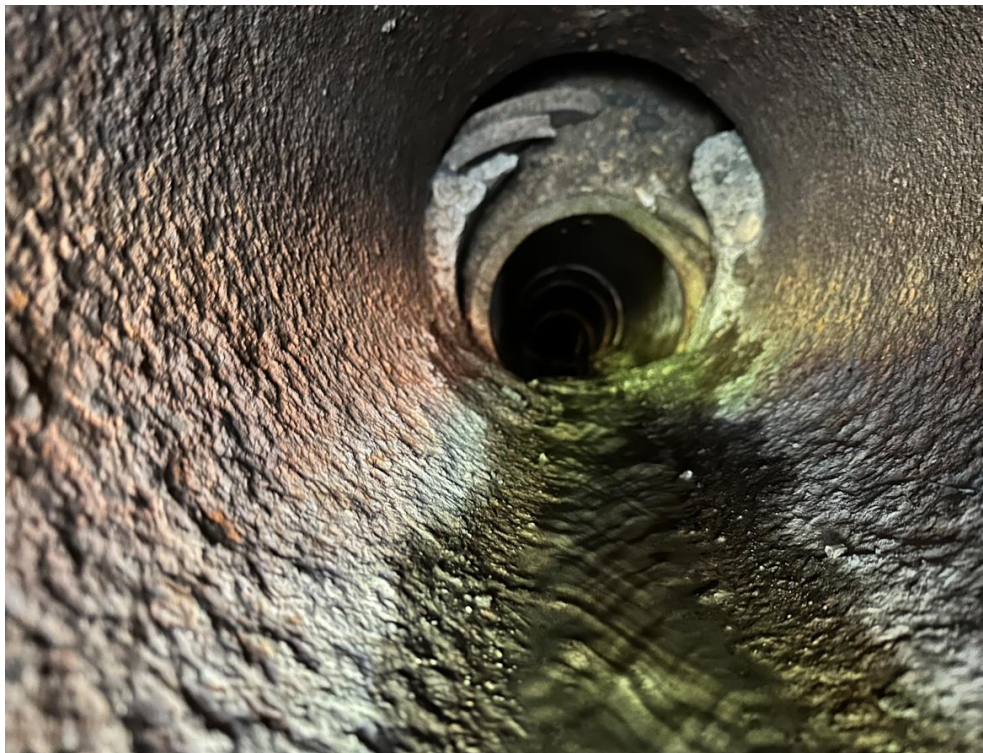
Figure 8 – Rue Notre Dame Underdrain, looking east at headwall.
