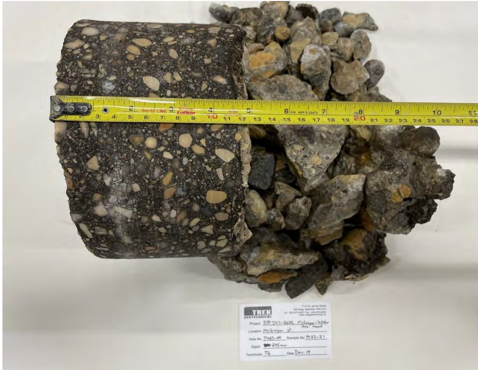
Photo 9: Pavement Core Sample at Test Hole TH23-09
