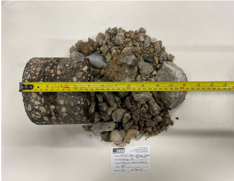
Photo 5: Pavement Core Sample at Test Hole TH23-05
