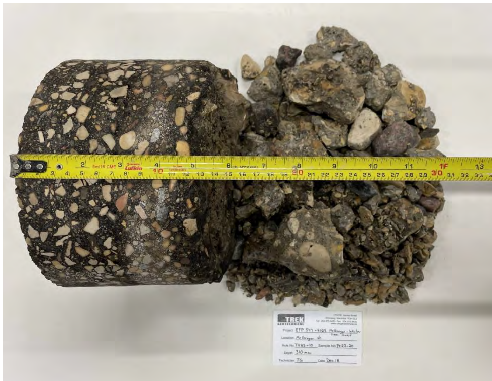
Photo 10: Pavement Core Sample P at Test Hole TH23-10
