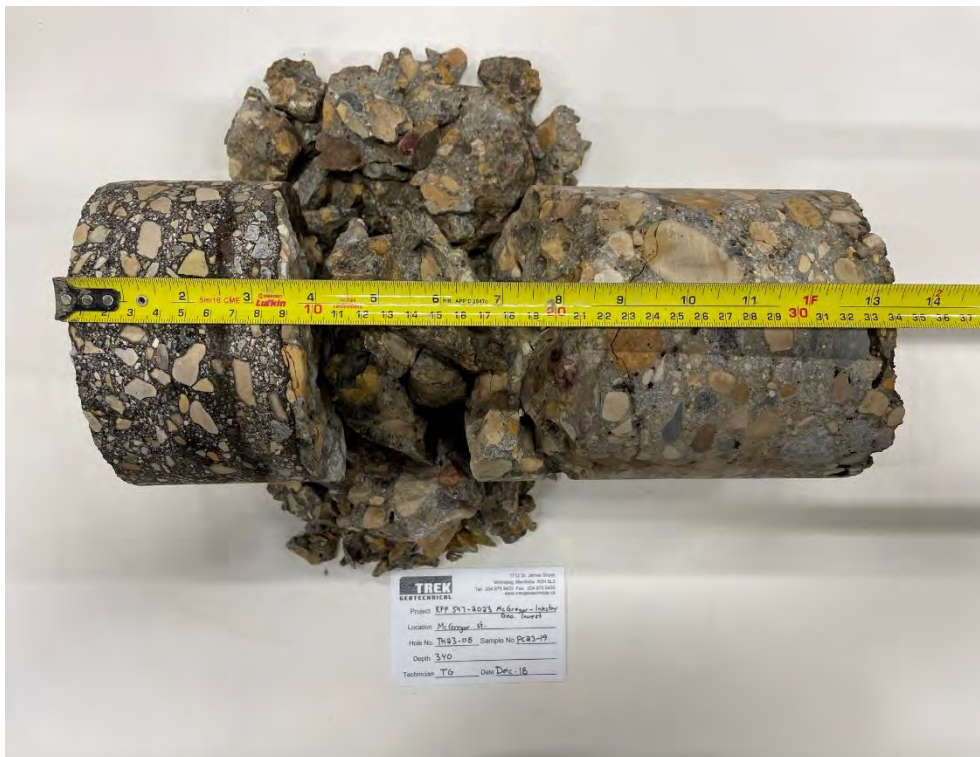
Photo 8: Pavement Core Sample at Test Hole TH23-08
