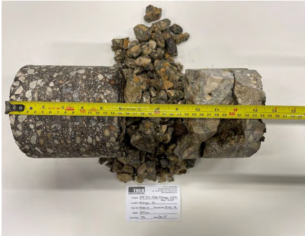
Photo 1: Pavement Core Sample at Test Hole TH23-01
