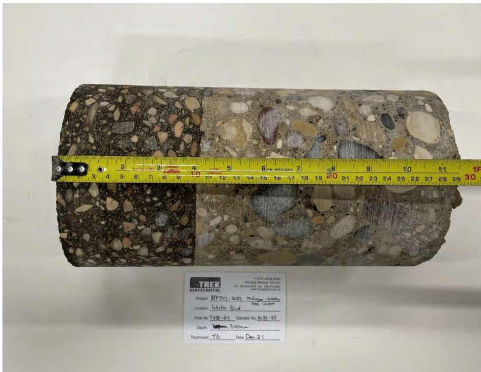
Photo 4: Pavement Core Sample at Test Hole TH23-24
