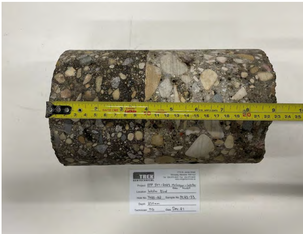
Photo 2: Pavement Core Sample at Test Hole TH23-22
