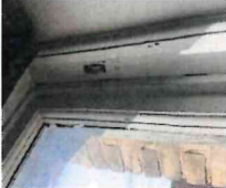
Weight pulley with sash rope cord missing on the majority of the windows.
