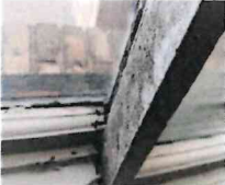
Upper sash meeting rail failure
