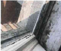
Window 2-23 - 2-30. windows are highly exposed to the sunlight and are are severely deteriorated
