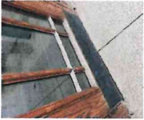
Bottom of entry door requires stripping of finish and refinishing.
