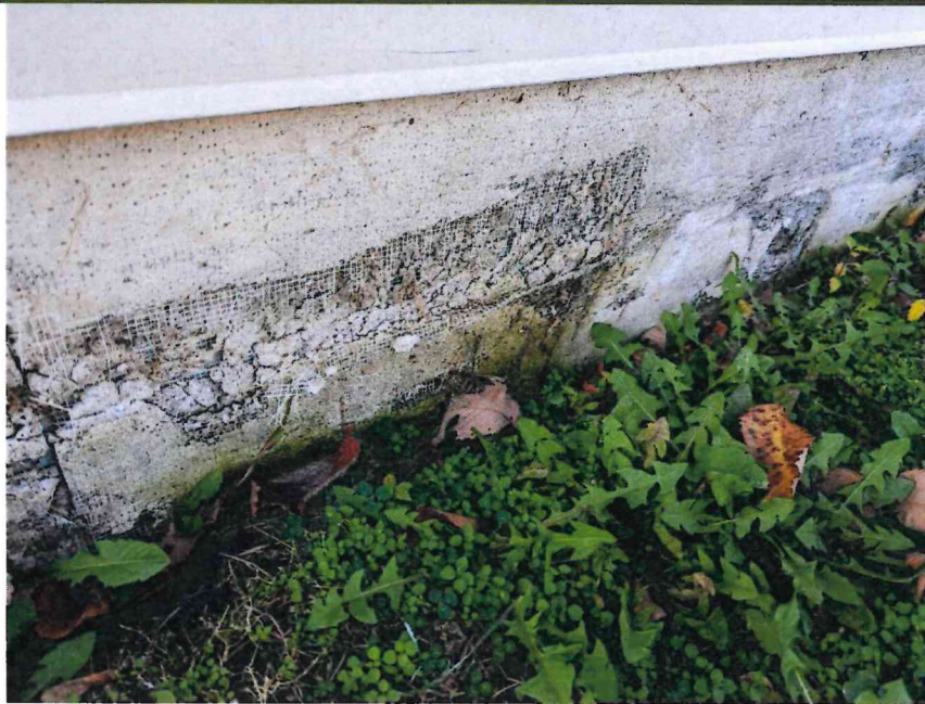
Photo 7: No asbestos-detected in the cementitious board on the foundation of the building.
