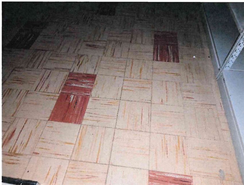
Photo 4: Previously confirmed asbestos-containing red and beige vinyl floor tiles.
