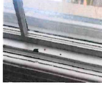
Jamb detail with window stop and interior storm are in good condition.
