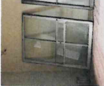
Typical venting storm sash.
