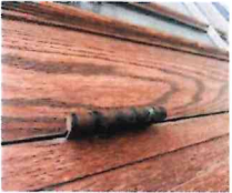
Hinges are rusted and need to be replaced with new NRP hinges
