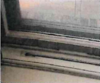
All sliding windows are weight and pulley double hung with a sash rope cord
