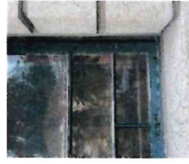
1-03: The inside check rail window is painted red on the outside, which was possibly the original colour.
