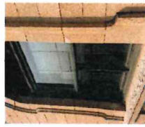
2-12, 2-13, 2-14, 2-31, 2-32, 2-33: Vertical bracing has been added to prevent the meeting rail from collapsing.
