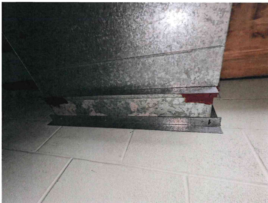
Photo 2: Previously confirmed red/brown mastic in the boiler room and film developing room.
