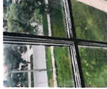
Interior storm windows are in good shape. Some require interior paint. All require a limited amount of putty work on the exterior.
