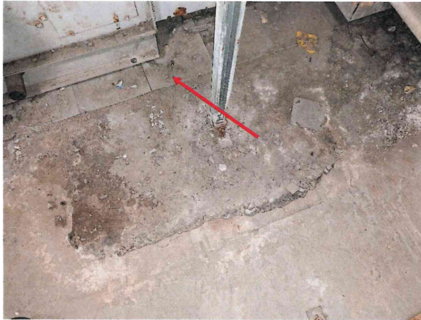
Photo 3: Non-ACM levelling compound on the concrete flooring in the boiler room, however the vinyl floor tiles beneath the air handler are asbestos-containing.
