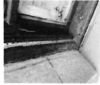
The window sill and brickmould are in good condition.
