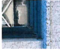
Typical sill detail. All bottom sashes and sills are rotted.
