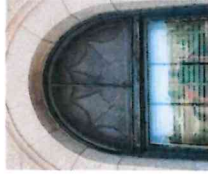
Transom sash all exhibit a combination of broken glass, rotted muntin bars, loose putty and metal bracing to hold them together.
