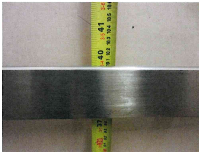
Height of existing handrails
