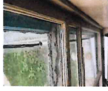
Interior view: check rail, storm window and sliding window
