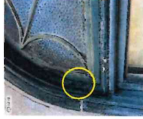
Typical transom detail. Note eye-and-hook indicate the original screens were held on by these fasteners. Current screens are nailed on with 3" nails
