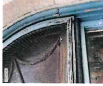
Transom detail. All transom sashes are deteriorated beyond repair.
