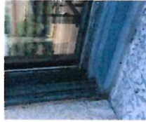
Typical sill detail with flashing to cover deteriorated sills.
