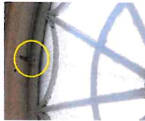
Transom clasps are either broken or seized.
