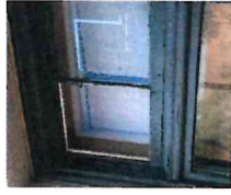
Hopper sash with chain stay
