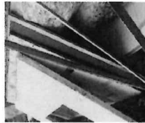
All basement windows were covered with Styrofoam and two sheets of plywood, along with a wood moulding on the outside. The interior sashes were mostly intact.
