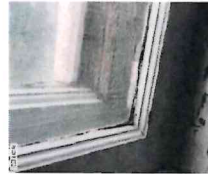
Interior storm window profile and putty deterioration
