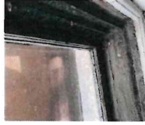
1-28: The south wall windows on the main floor have been protected from the adjacent building and have had very little sunlight as a result of the windows are in much better condition than the second floor windows.
