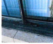
All meeting rails have failed and are held together with metal brackets.
