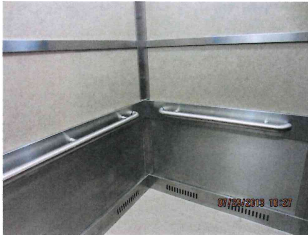
Typical modernized wall panel layout (mirror on back wall)
