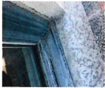
General sill condition with pressure treated repair
