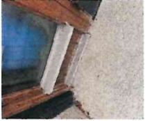
Sidelite require stripping of finishing and refinishing.
