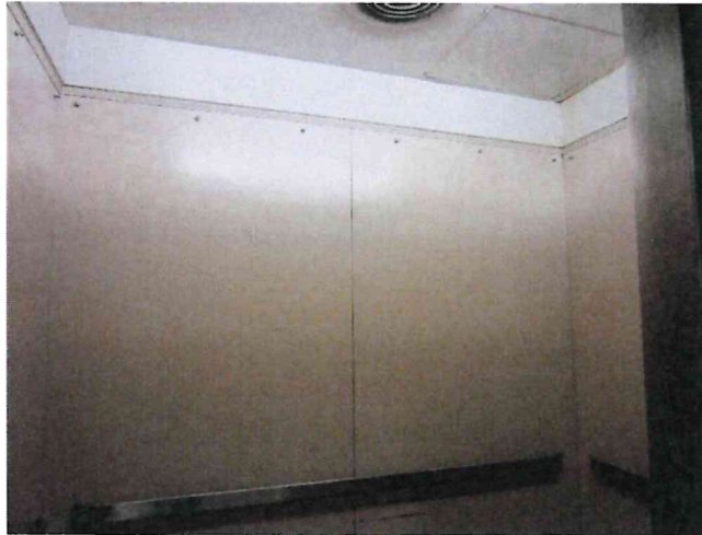
Existing steel flat wall cab design
