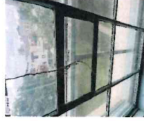
Interior storm window with hinge venting window
