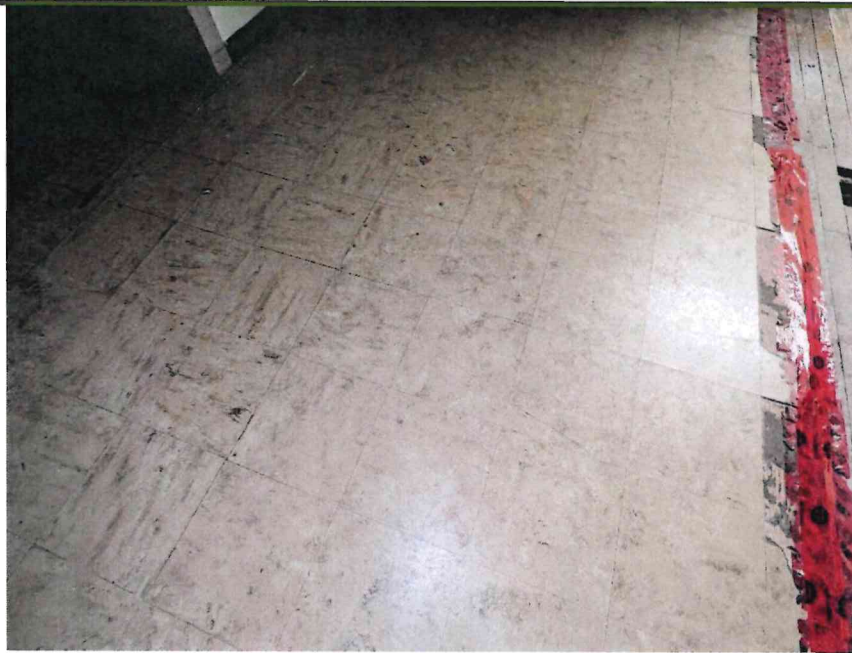
Photo 5: No asbestos detected in the 9"x9" vinyl floor tiles present through most of the main floor.
