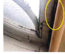
Interior view of transom sash. Hinges are rusted and need to be replaced.
