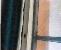
Double hung window damage occupants prying double hung sash down.
