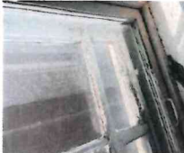
Inside view of venting storm window.
