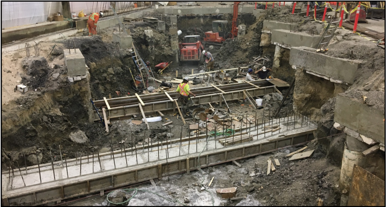
PHOTOGRAPH #1: Excavation as seen facing east from west side of excavation.
