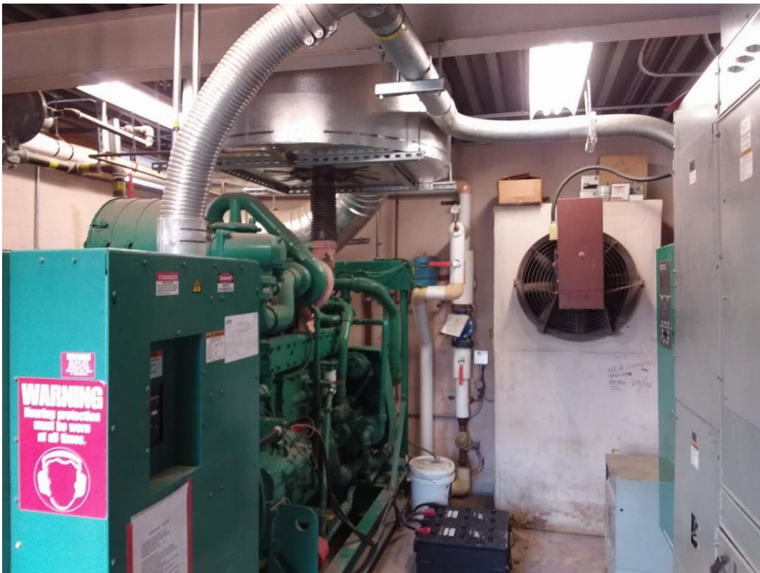
Generator Building (Location #: 3)
