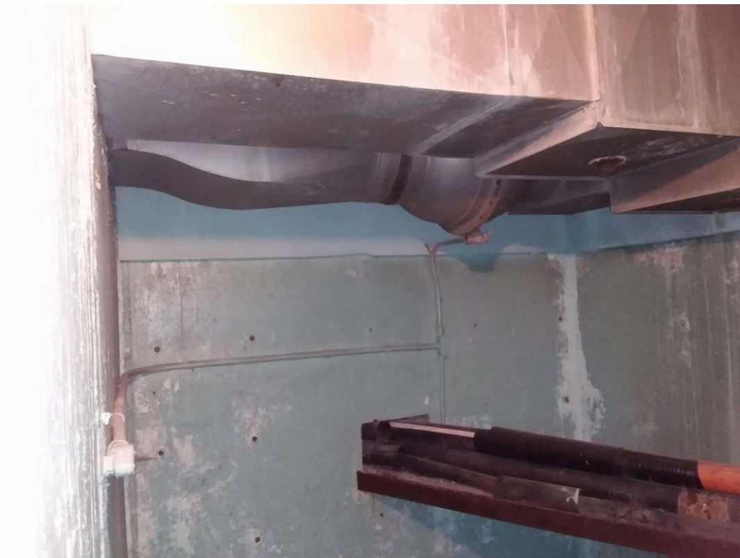
V9500 (Presumed Asbestos), Duct, Duct Connector, Textile, Decommissioned Entrance Chamber (Location #: 2)
