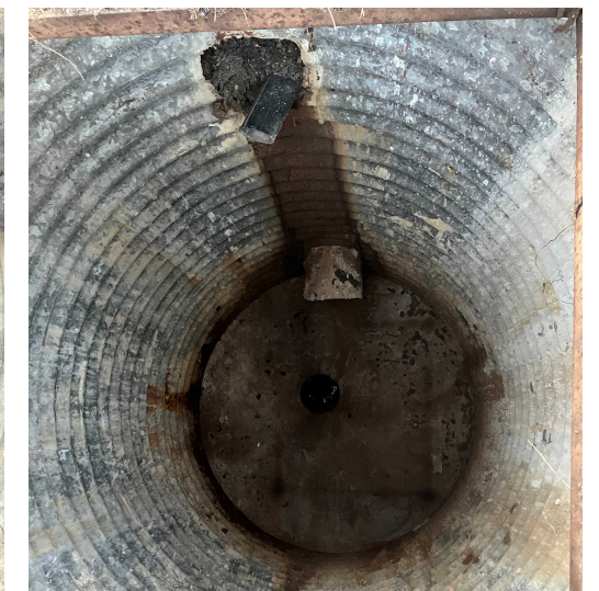
*Photo of Drainage Lines & Corrugated Metal Basin at Property Line
