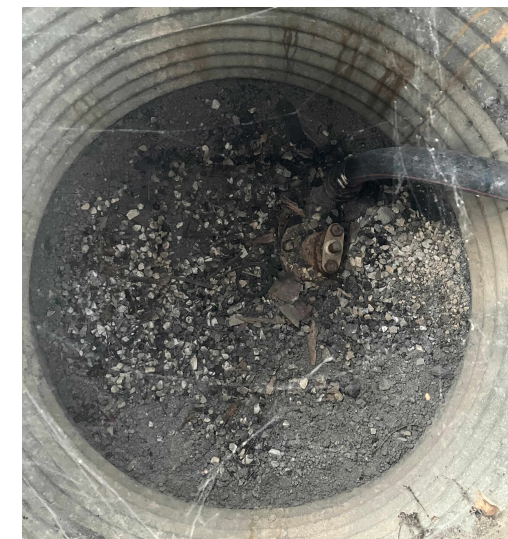
*Photo of Wading Pool Apron Vault, Drainage Valve & Lines
