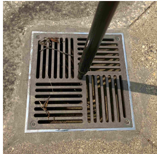
TBM3 : 232.127 *centre of wading pool drain
