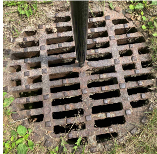
TBM2 : 231.922 *centre of catch basin lid
