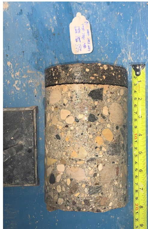
Figure 4 – Core Sample No. 237 – Simpson Ave
