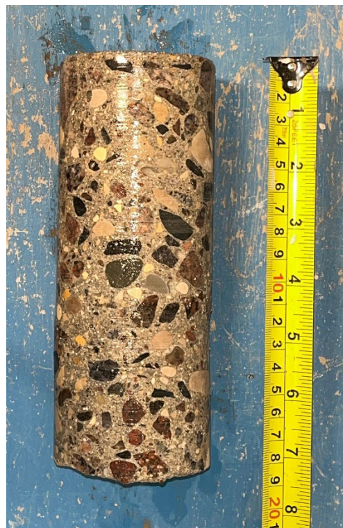
Figure 14 – Core Sample No. 265 – Thorndale Ave
